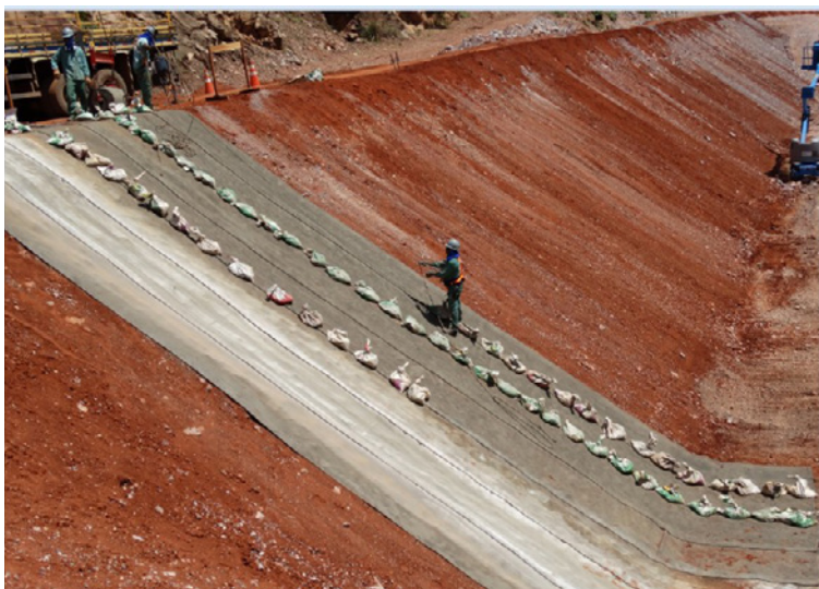
CC13™ was used to line the lagoon
