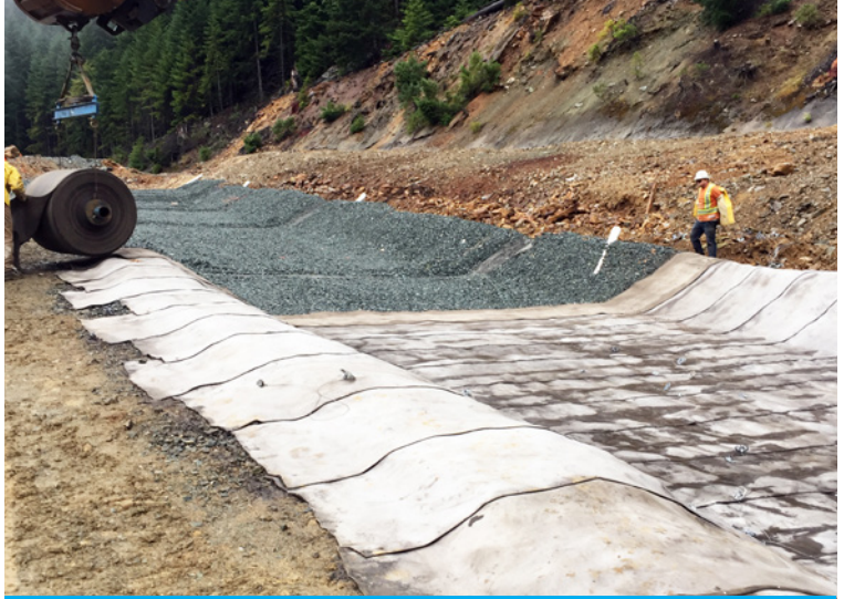
The CC was unrolled from a spreader beam mounted to an excavator
