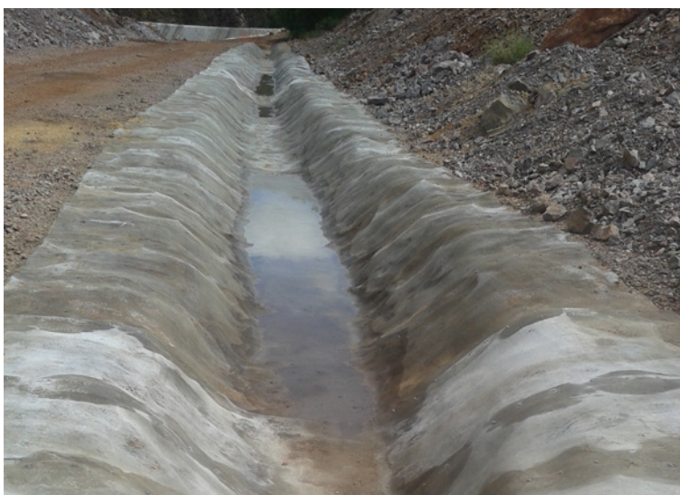
The adjoining channels were also lined with CC13™
