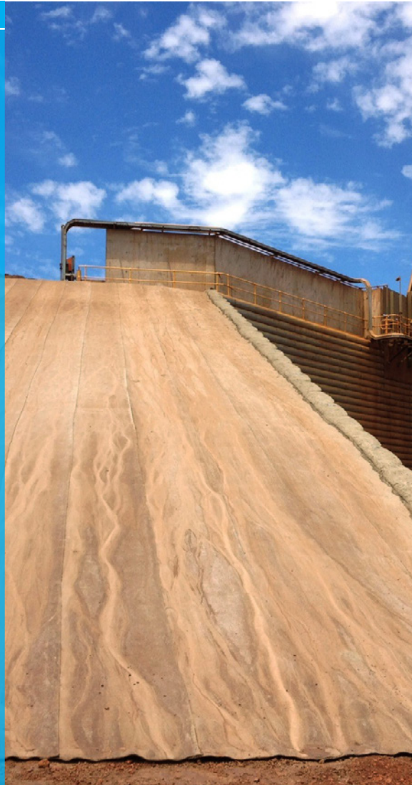
The CC was laid vertically down the slope and the side filled with poured concrete
