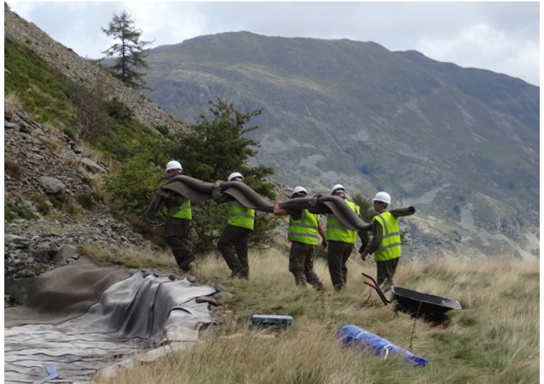
Site access was limited, so the CC had to be transported manually
