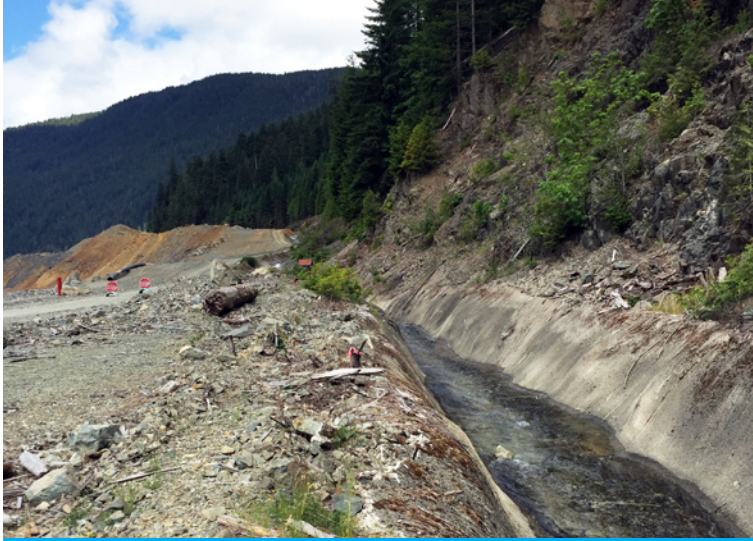
The original concrete lined channel
