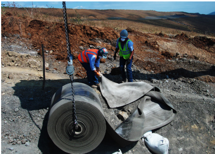
CC8™ was delivered to site in bulk rolls
