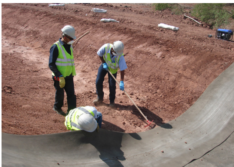
CC8™ was laid transversely across most channels
