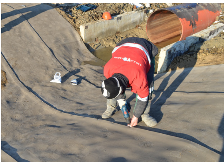
Screws and ground pegs were used to secure the CC
