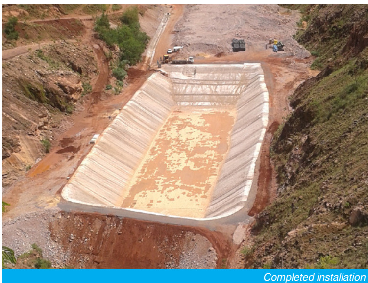
The adjoining channels were also lined with CC13™
