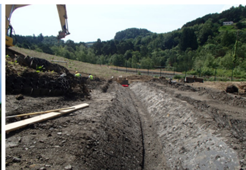
The channel was excavated prior to installation
