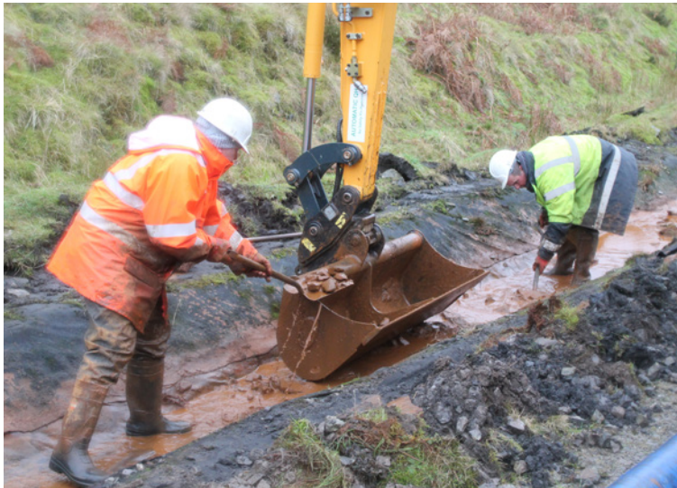
The team cleared the channel of debris and drained it prior to installation
