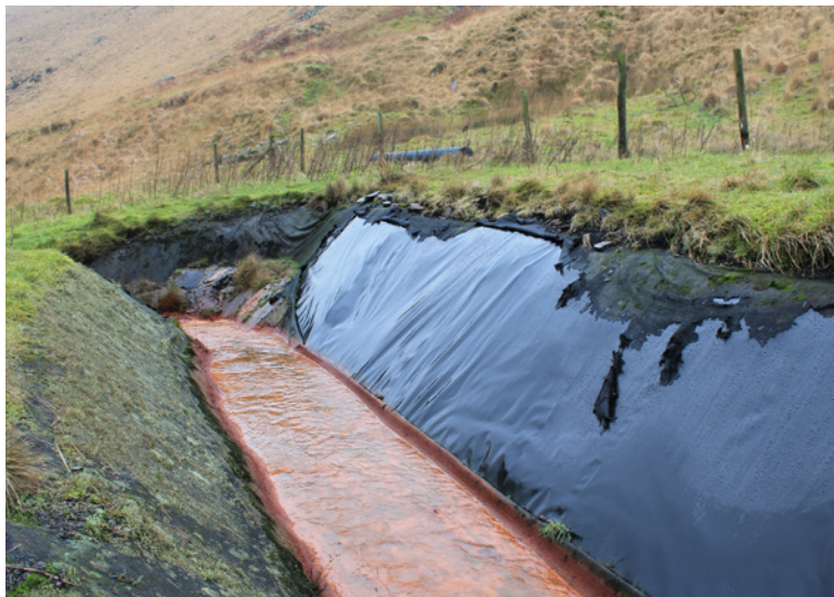
The original channel was contaminated with ochre discharge from the mine
