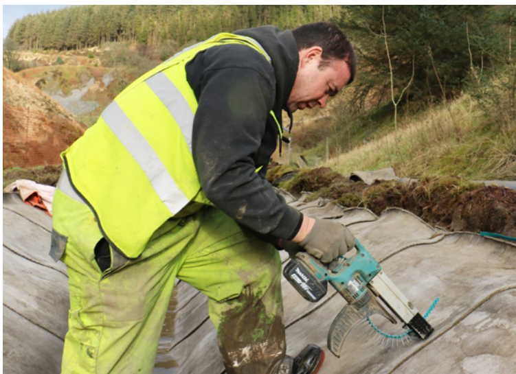
Screws were used to join the CC layers
