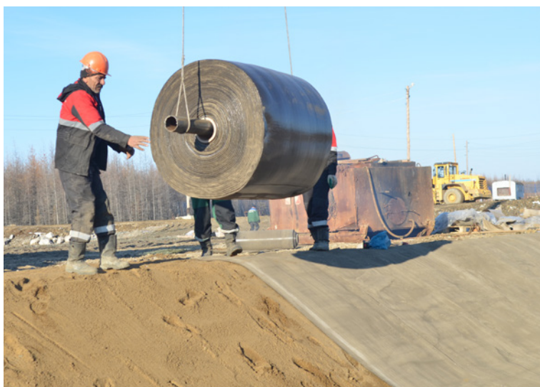
A spreader beam was used to deploy the CC
