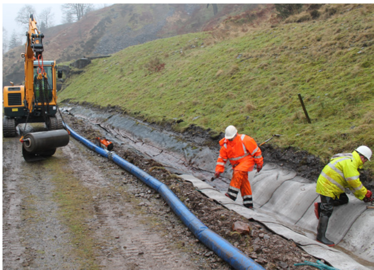
The CC was delivered in bulk rolls
