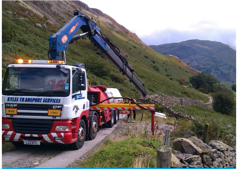
CC was delivered to site by truck and helicopter in bulk and batched rolls
