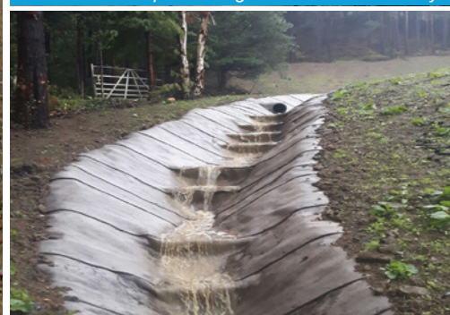
Steps were installed in places to dissipate water flow
