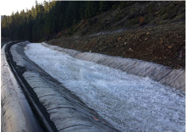
The CC channel was wider than the original to accommodate fast water flow
