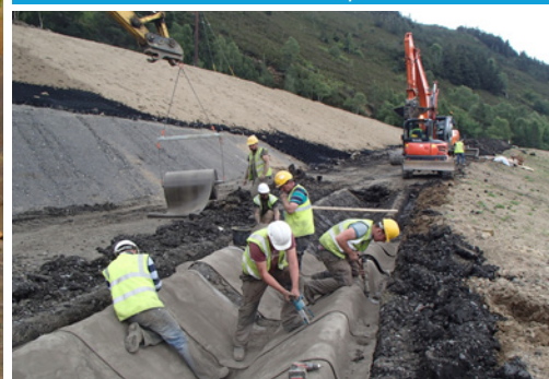
CC was cut to profile length and laid transversely
