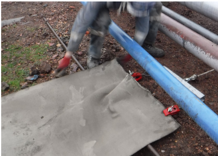
A modified light-weight spreader beam was used to pull CC under the pipes
