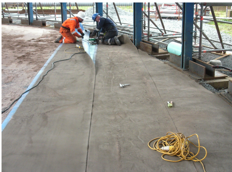
Thermal welding and testing of the joints
