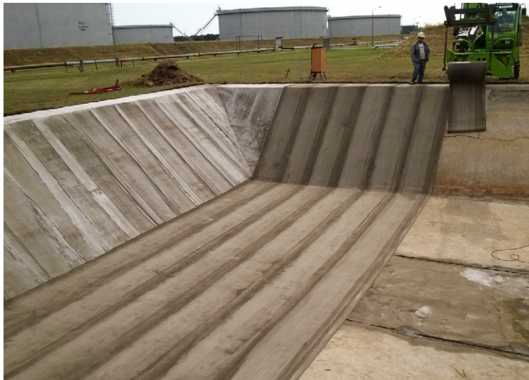
CC was unrolled from a spreader beam loaded on a Zoom Boom
