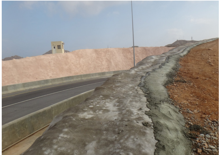
Edges of the CC were backfilled using concrete at the crest of the slope
