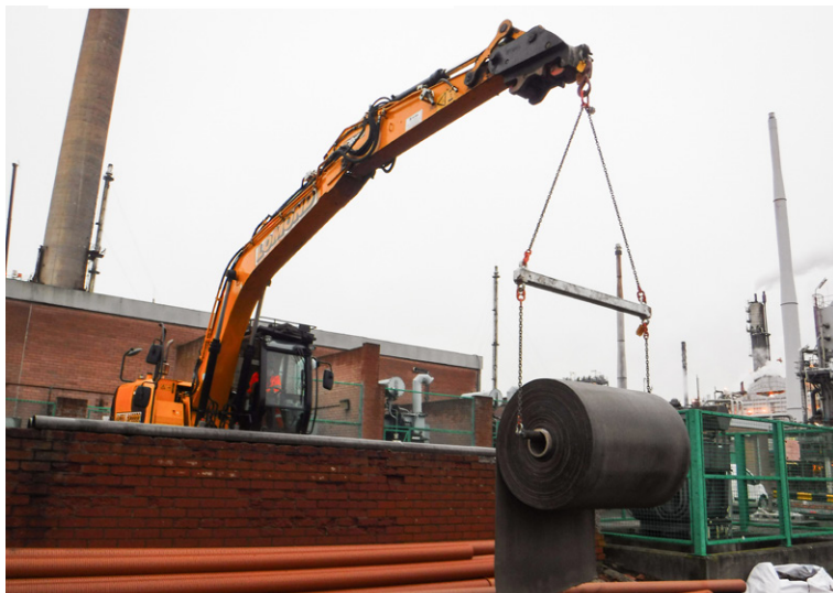
CC was delivered to site in bulk rolls and unrolled from spreader beam
