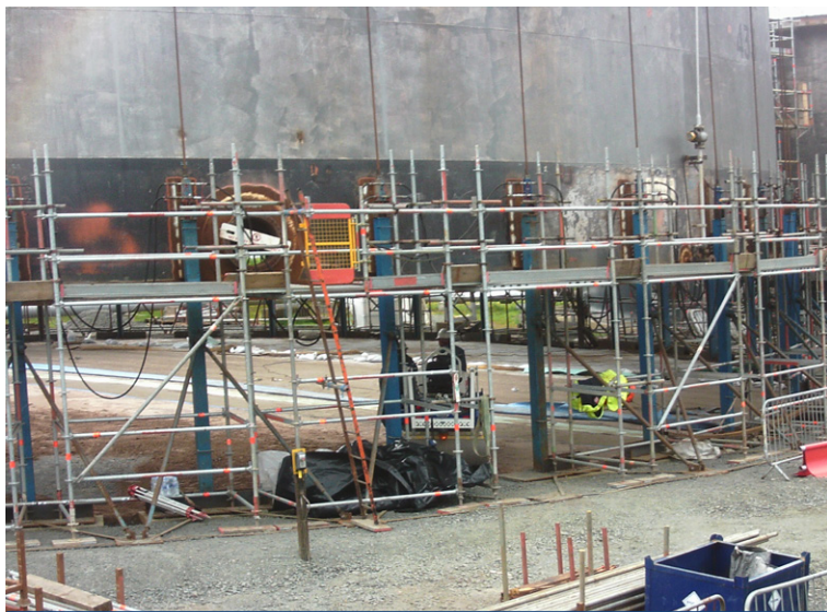
Tank jacked up by 2m around the full perimeter
