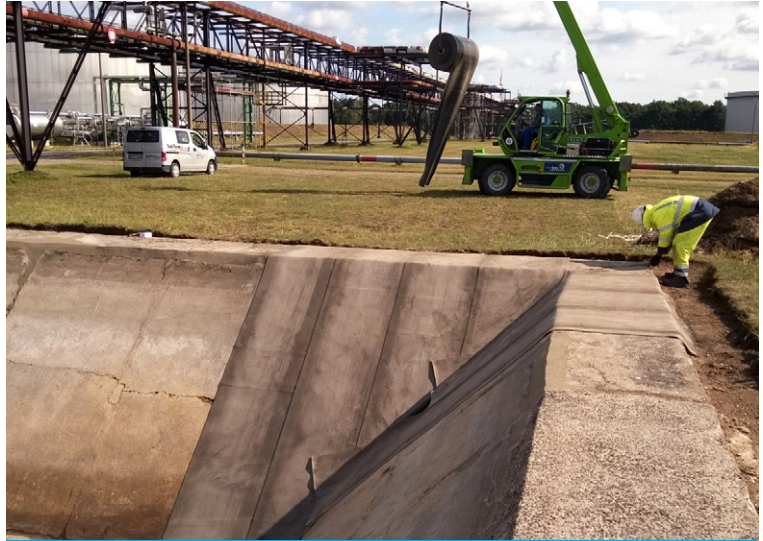
The team first laid alternating perpendicular layers at the corners
