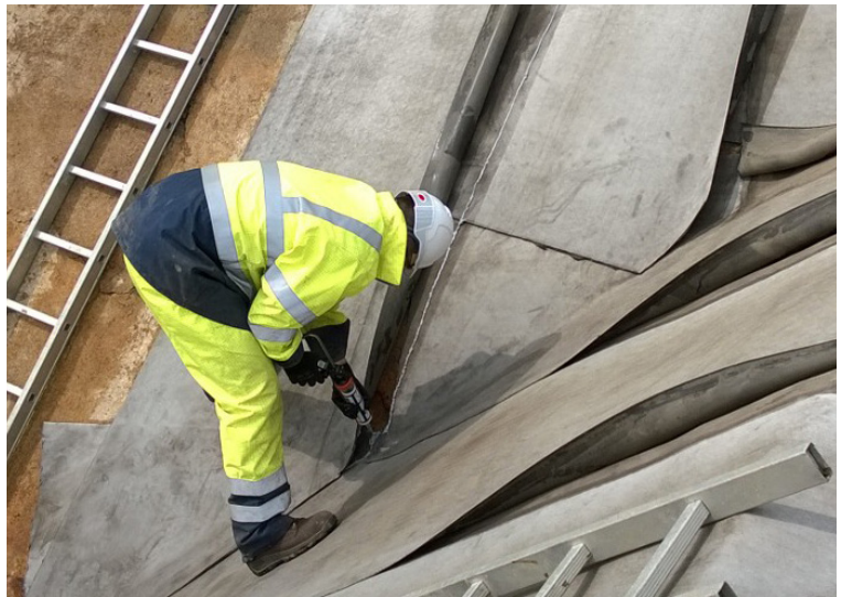
Overlapping layers were sealed with an adhesive sealant
