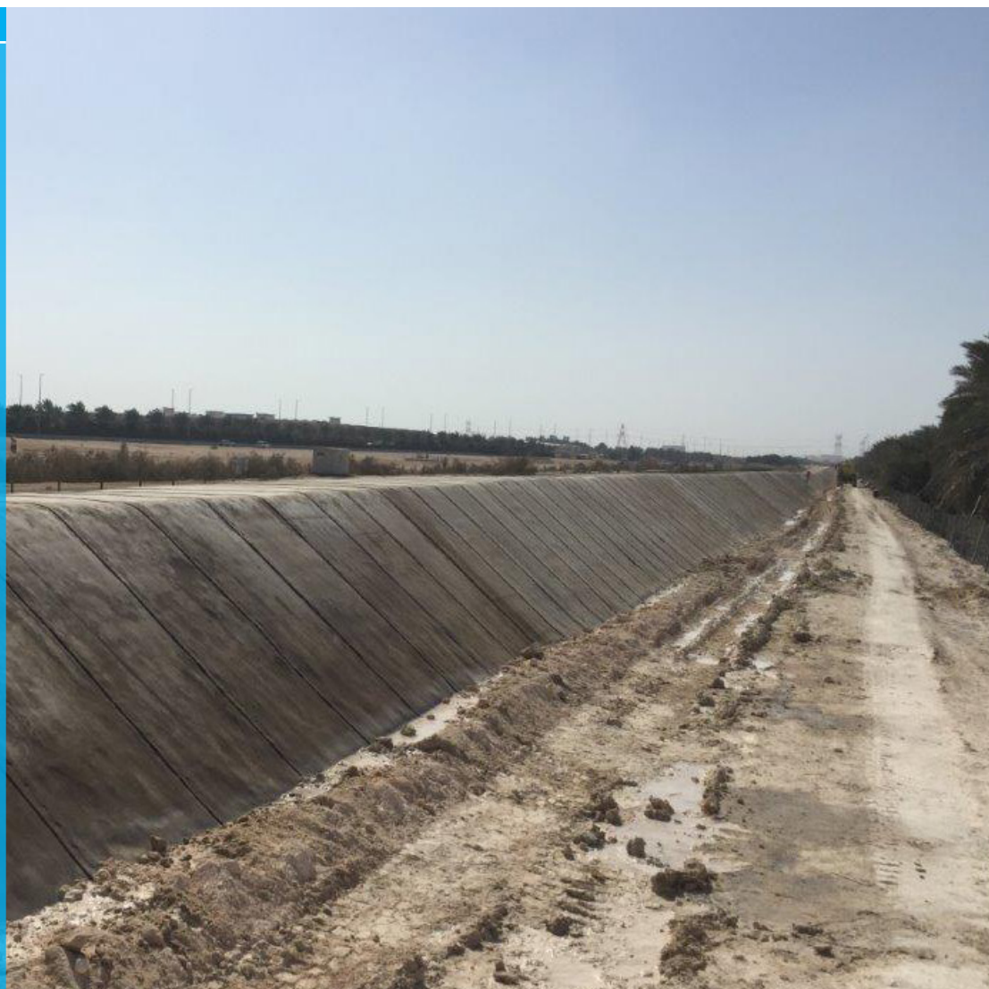
Completed bund lining installation
