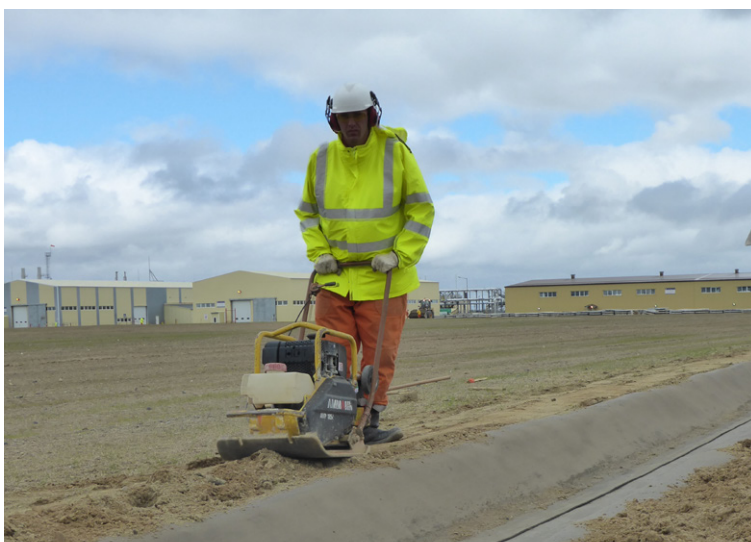
Anchor trenches were backfilled with soil and packed down
