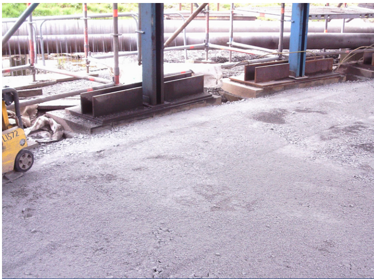
Preparation of the substrate
