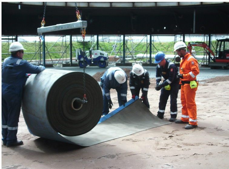
Deployment of the CC Hydro™
