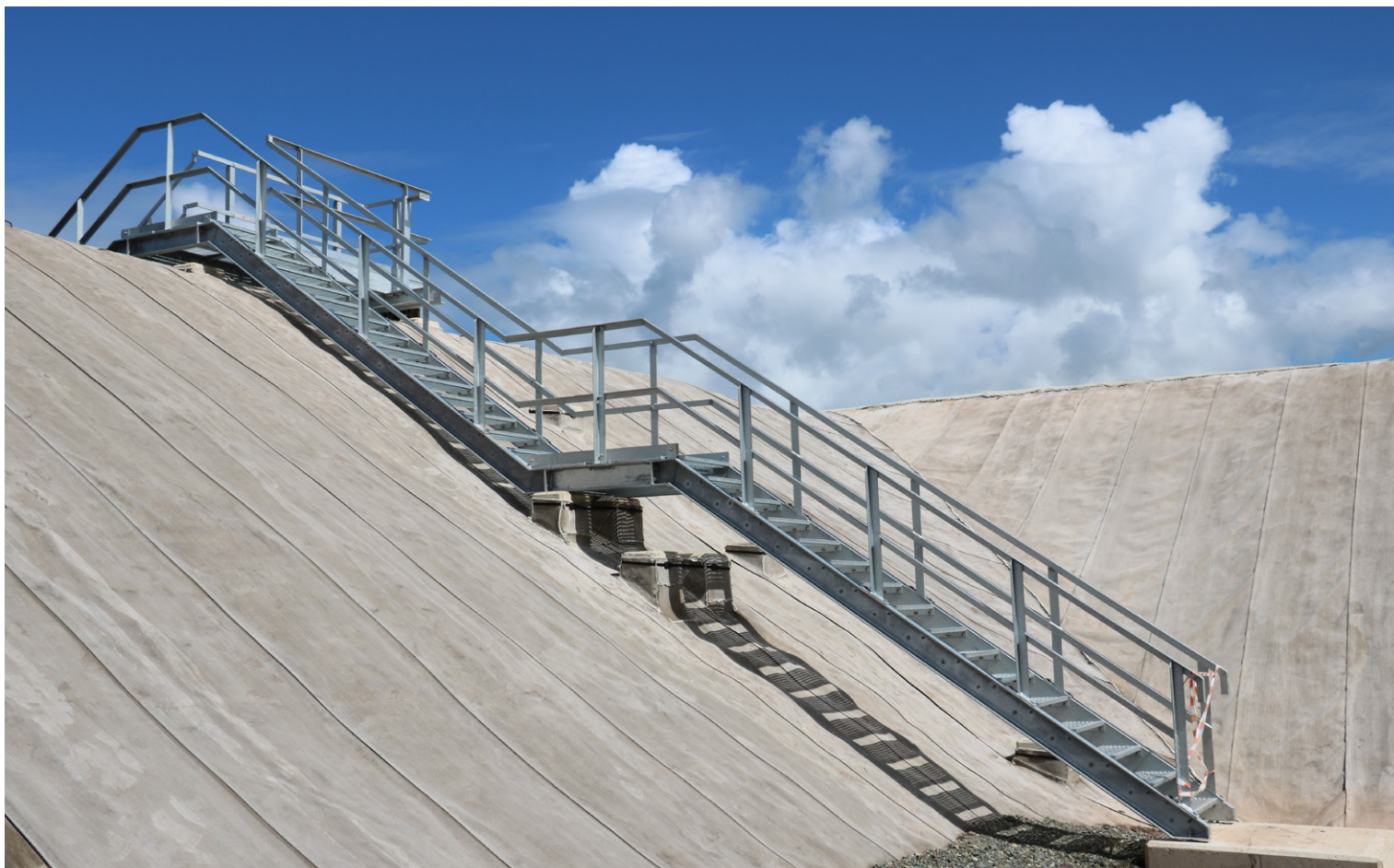
CCH installed around the steps
