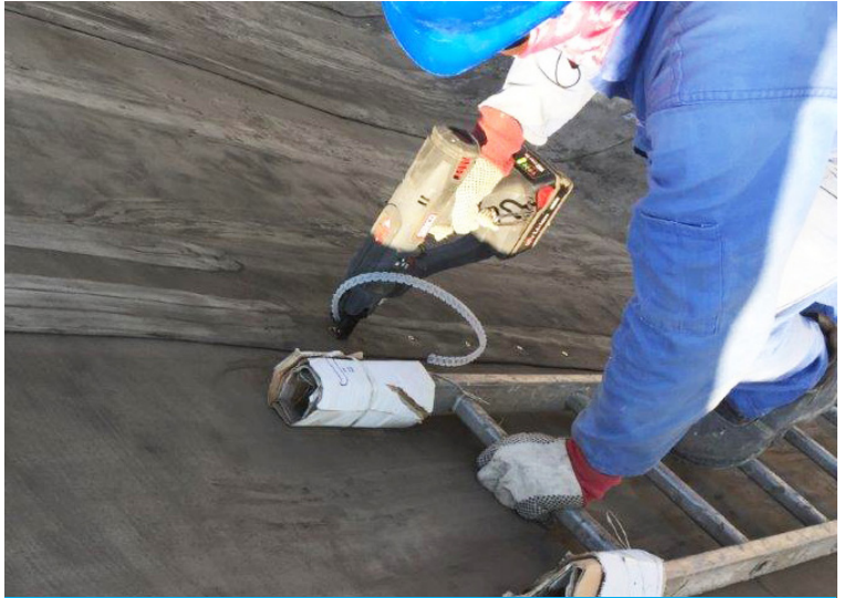
Screws were used to secure the CC
