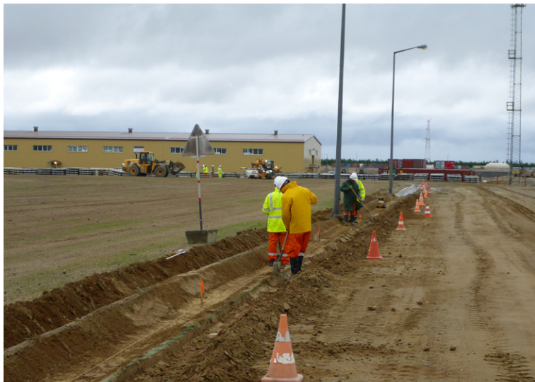
The channels were prepared by hand and anchor trenches dug
