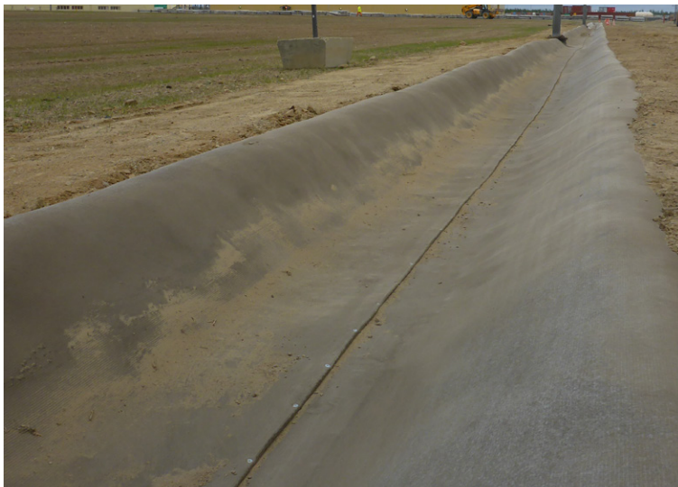
Both longitudinal and transverse layups were used
