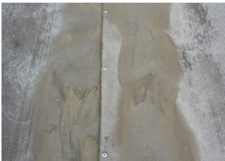
CC was fixed with adhesive sealant and screws
