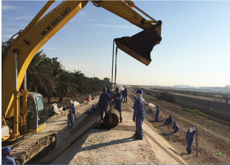
CC was delivered to site in bulk rolls and deployed from a spreader beam
