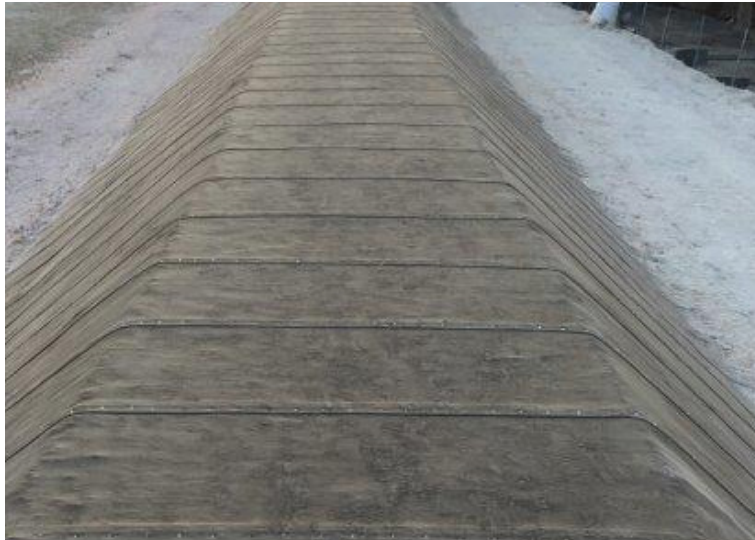
The CC was laid transversely across the bund
