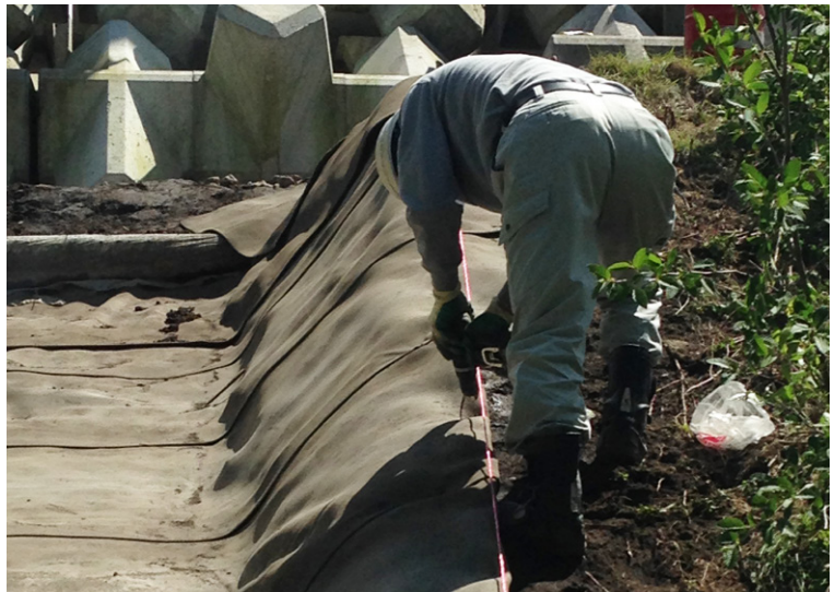
The CC edges were folded beneath themselves for neat termination
