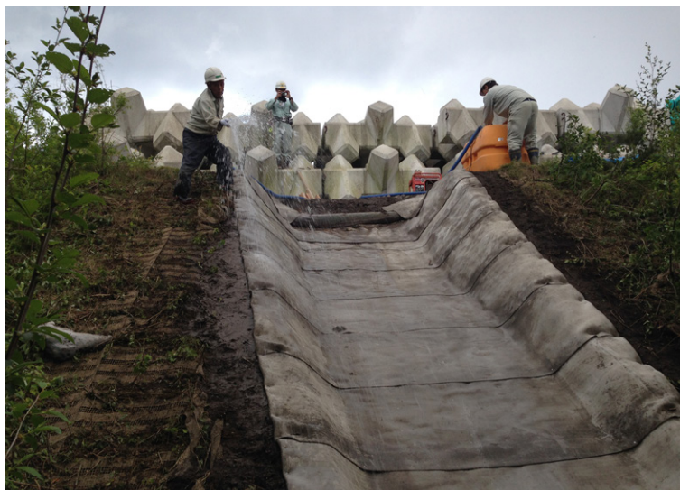
Hydration of the completed installation
