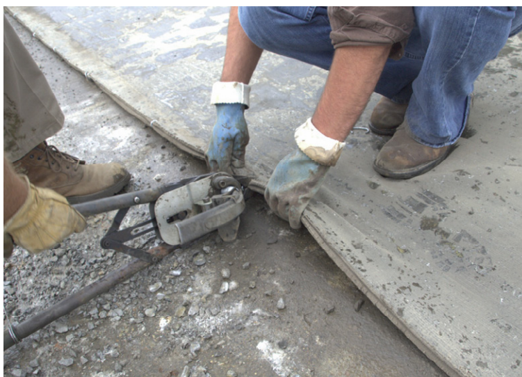
Connecting the CC panels with hog rings
