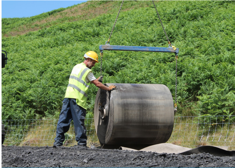
CC was delivered to site in bulk rolls
