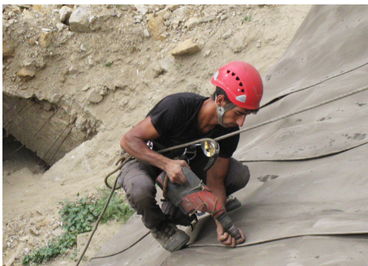
Screws were used to fix and join the layers of CC
