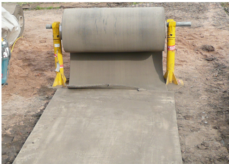
CC was delivered to site in bulk rolls and batched to length on site
