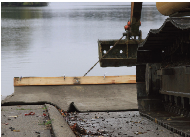
Deploying the CC into the lake
