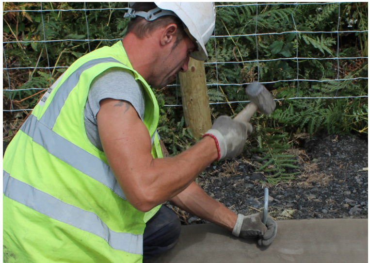
The CC was fixed to the ground at the edges using ground pegs
