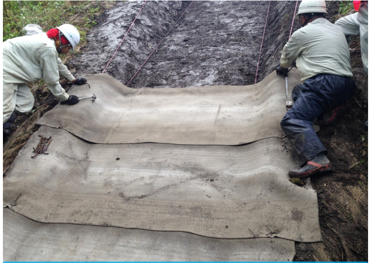
The CC was laid horizontally down the slope
