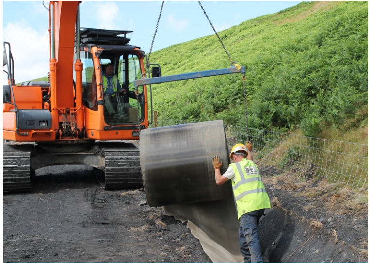
A spreader beam and heavy plant were used to deploy and lay the CC
