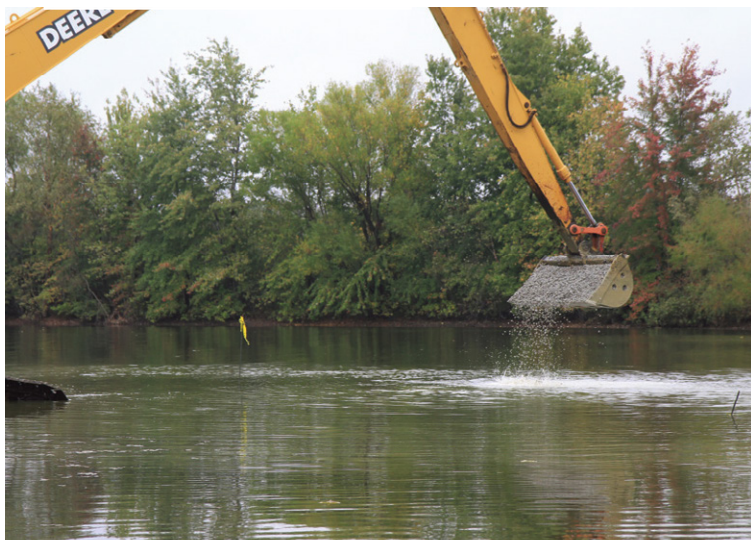
Removal of old gravel ramp extension
