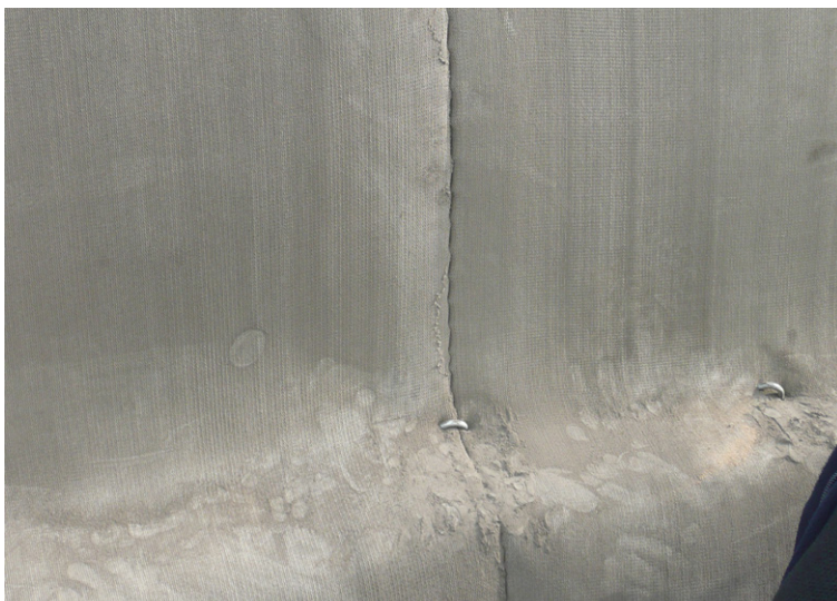
The CC was secured with hog rings and staples
