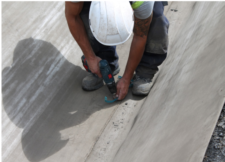
Screws were used to joint the CC at the overlaps
