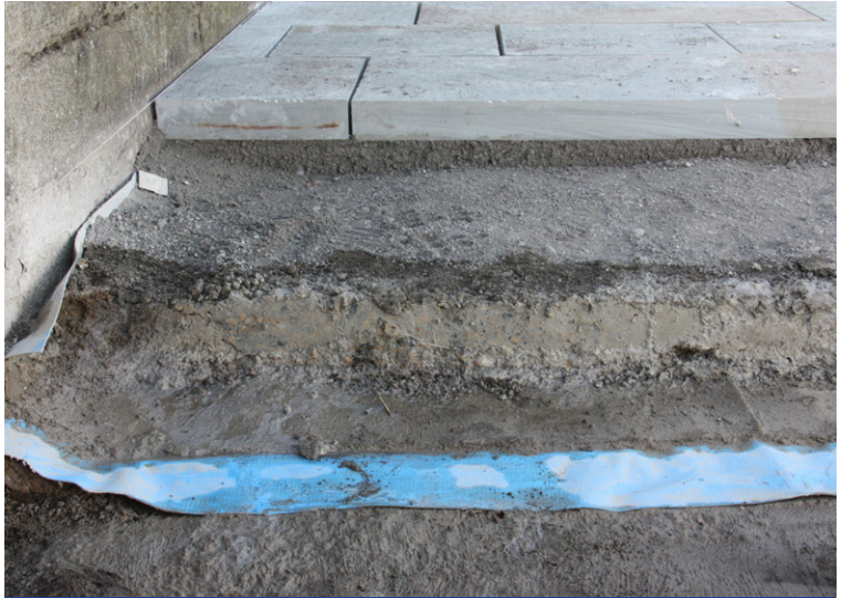
CCH layer underneath re-laid substrate and flagstones
