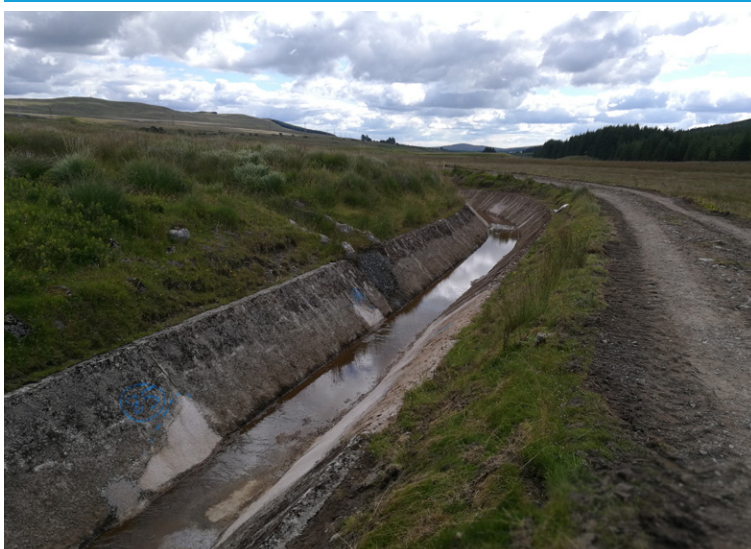
Vegetation & algae removed and water diverted out of the flume
