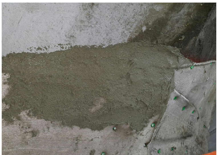
Mortar and sealant was used to prevent ingress at the edges of the CC
