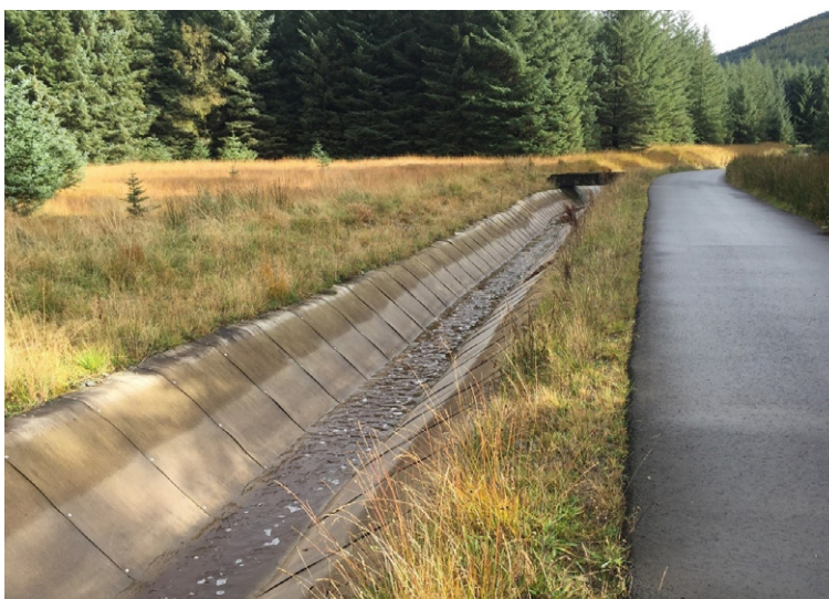
Original Bowburn Flume 4 years after installation requires minimal maintenance
