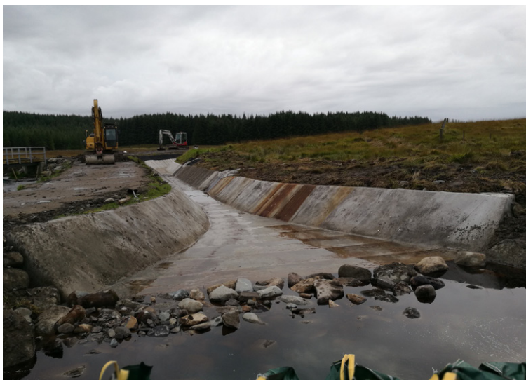
Flume inlet with an anchor trench running across the width of the channel
