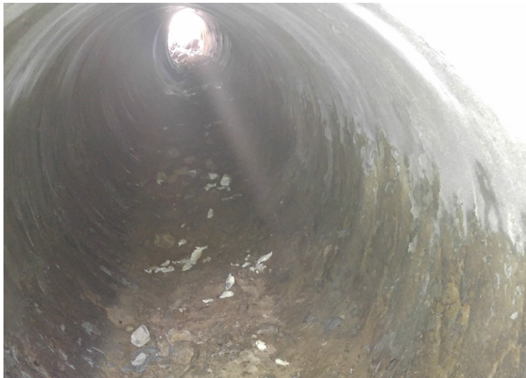
The inside of the pipe had to be cleared of rocks and debris prior to works
