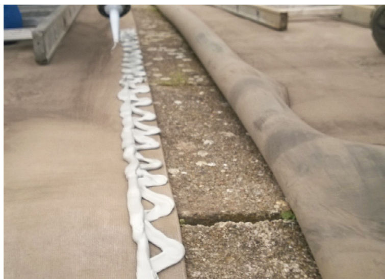
Sealing under the overlap
