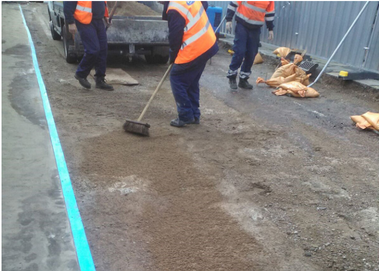
The substrate was flattened before installation
