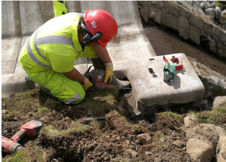
Installing 34mm Hilti nails with 25mm washers
