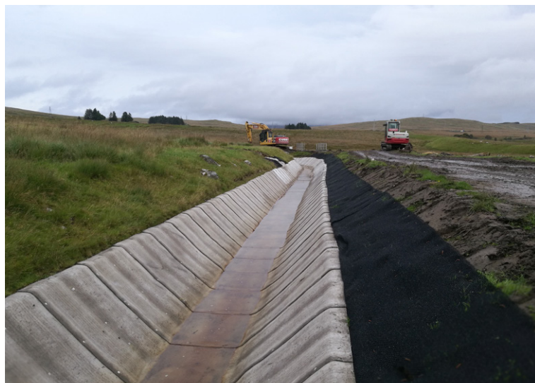
CC layers overlapped in the direction of water flow providing natural weep paths
