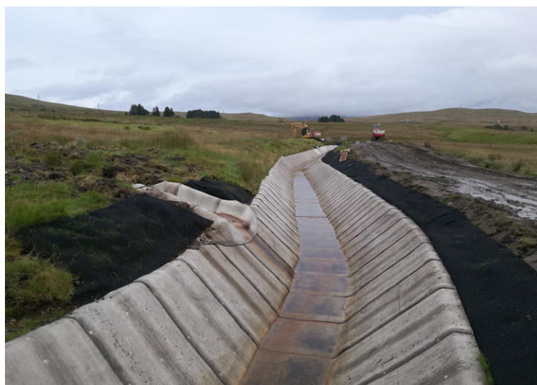
Remediated flume lined with CC8™ transverse layers
