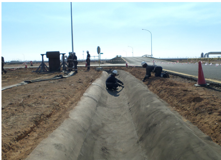
CC5 was laid down the middle, with CC8 laid either side
