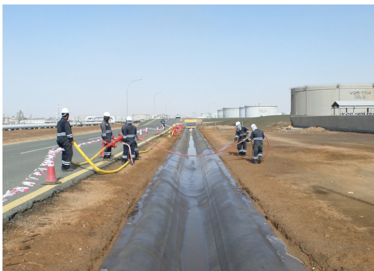
CC was hydrated using a fire hose
