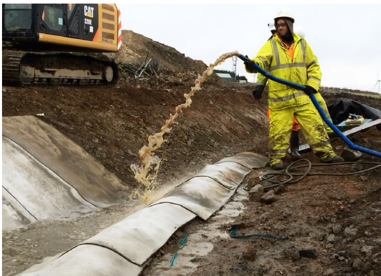
Hydration of CC8™ via bowser and petrol pump
