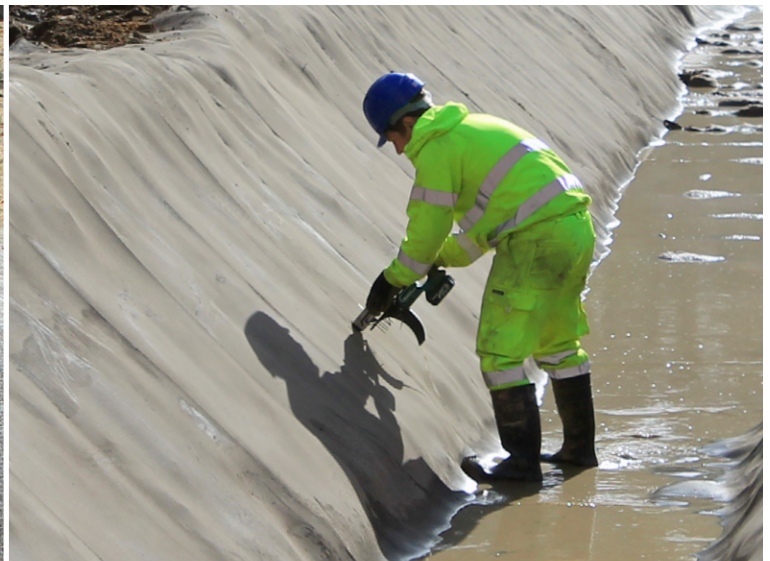
The CC was jointed with screws
