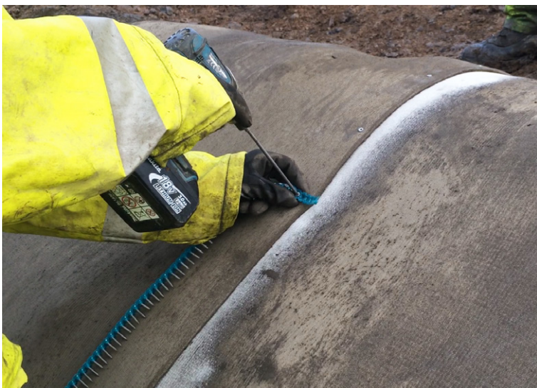
Transverse layers with a 100mm overlap were screwed in place
