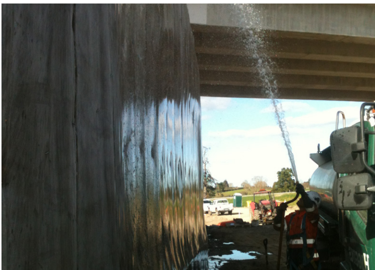
Hydration of the CC installation
