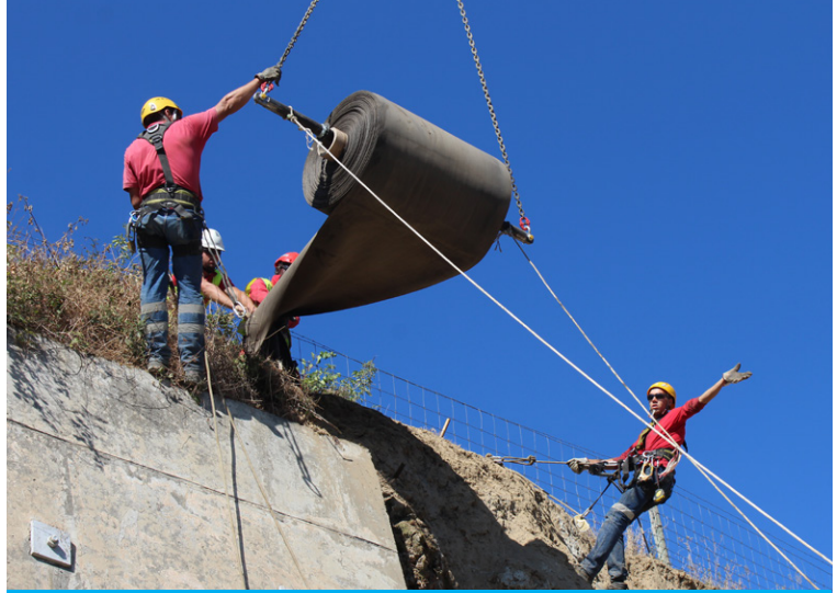
CC was attached to existing concrete with masonry screws
