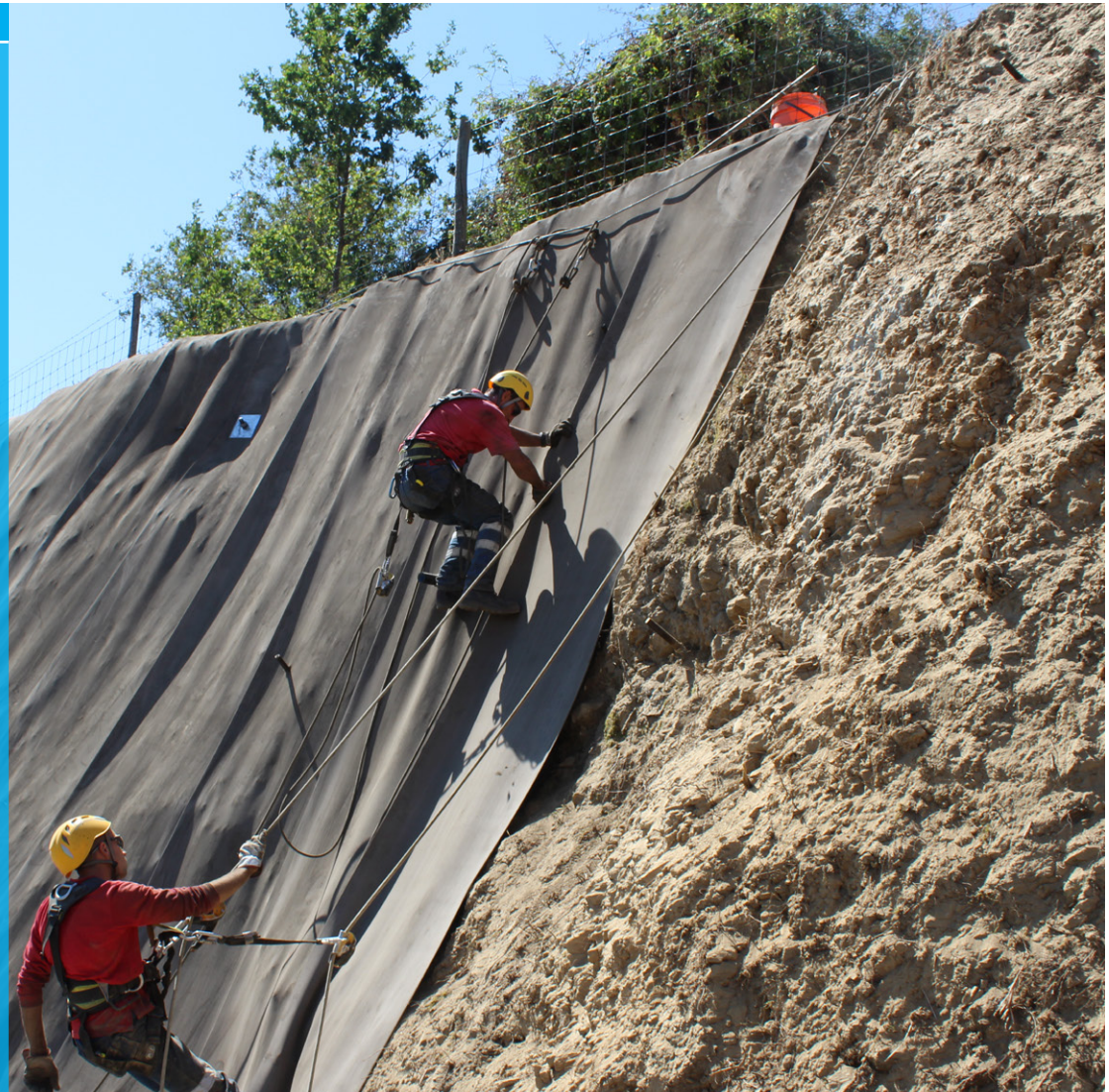
Installation of CC at Highway A24, Nó da Régua
