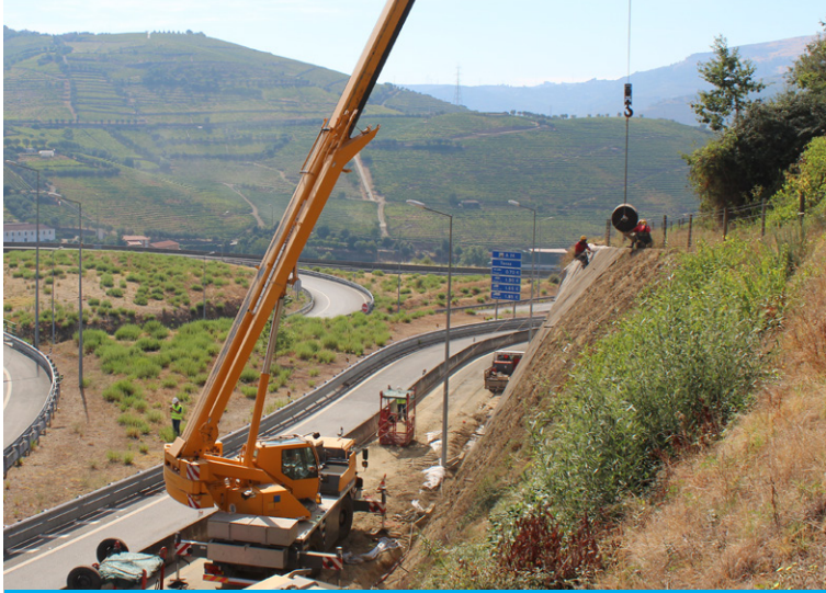
CC was craned from the base of the slope to the top on a spreader beam
