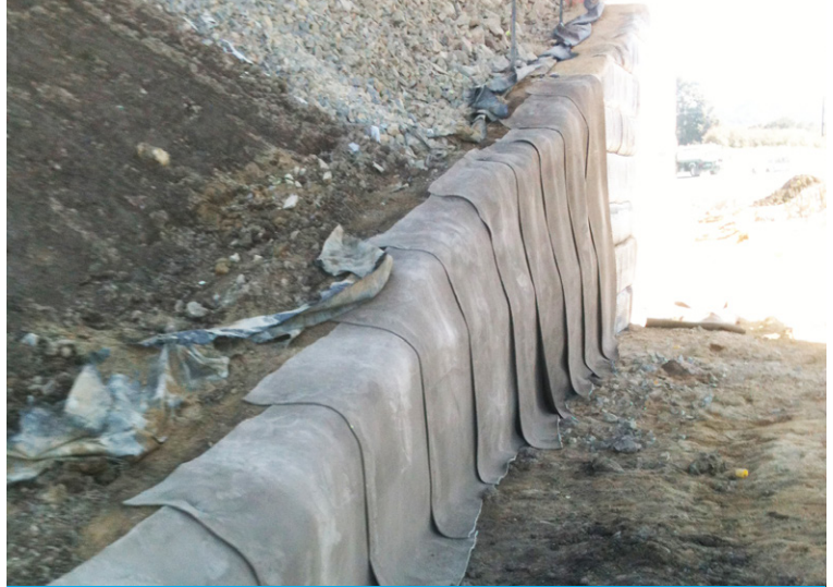
CC was cut to length on site to match length of each slope section
