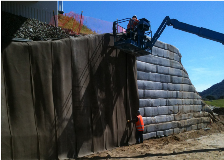
A cherry picker was used to assist during installation
