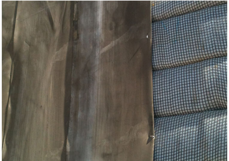
CC was jointed using 30mm screws
