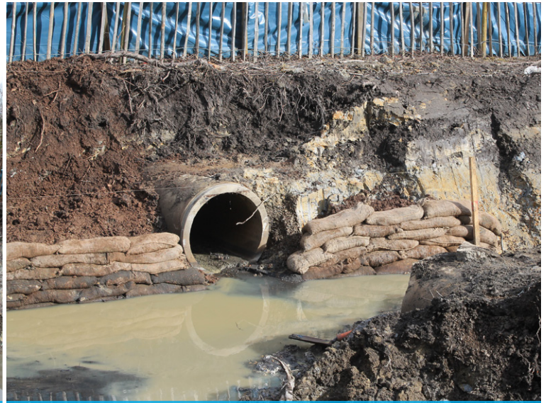
Sandbag retaining wall
