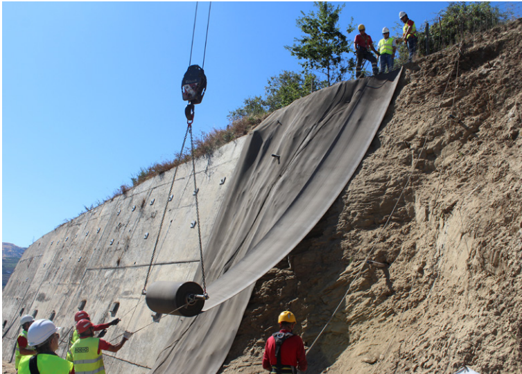
The team ensured an overlap of 100mm during deployment
