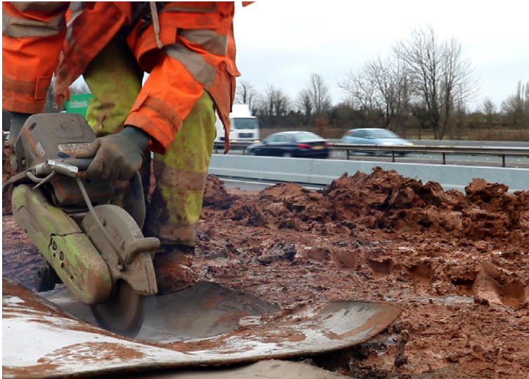
Power tools were used to cut the CC
