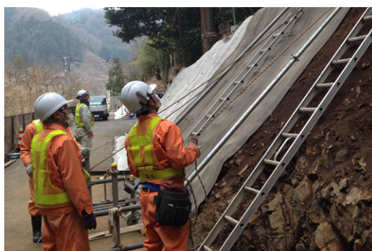
A pulley system was used to deploy the CC
