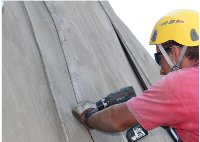
Every other screw was closer to the edge, forming a triangular pattern
