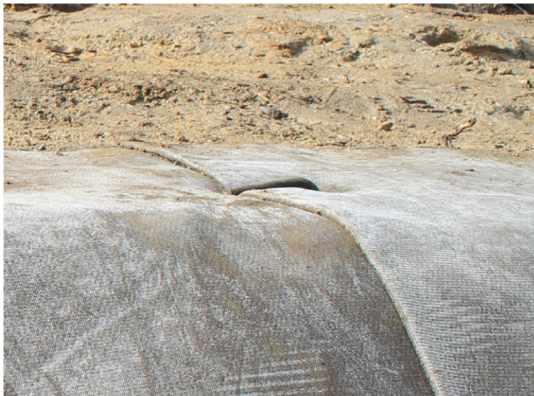
Pegs were inserted through the overlap
