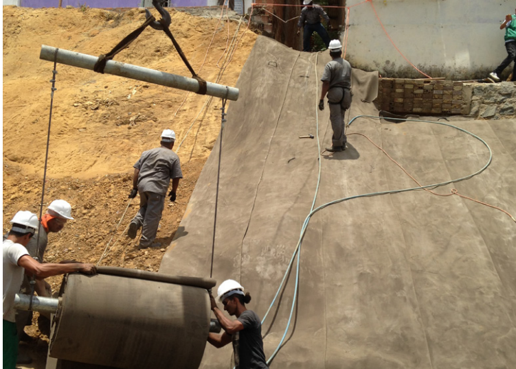
CC spooled down the slope
