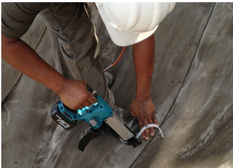
Joints were screwed every 200mm with a double row of screws
