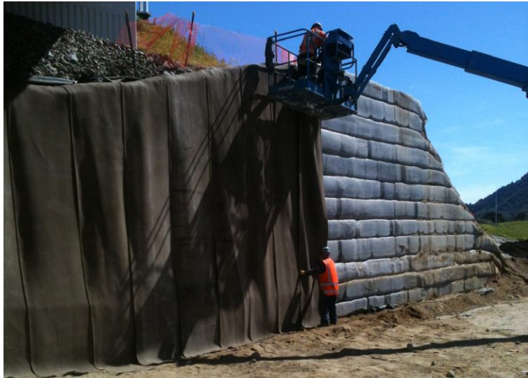
A cherry-picker was used to lift sections of CC to the top of the slope
