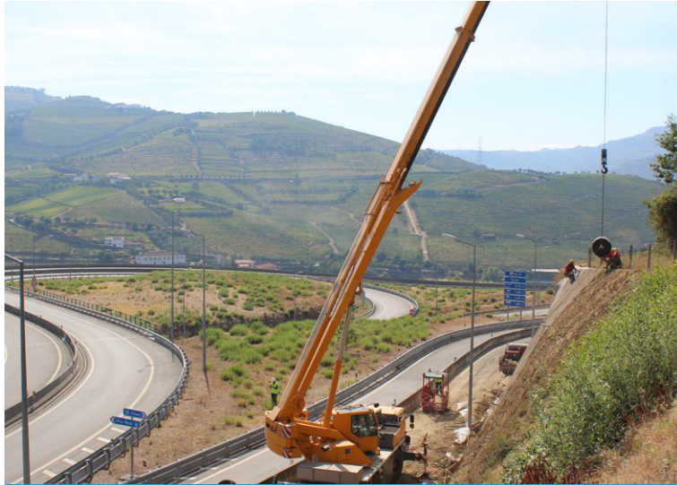
The CC was mounted onto a spreader beam and hung from a truck crane
