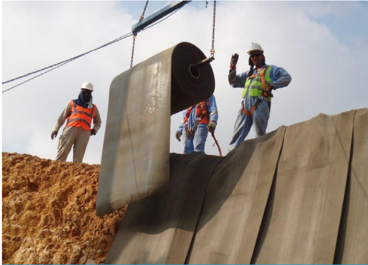
CC being lifted into position
