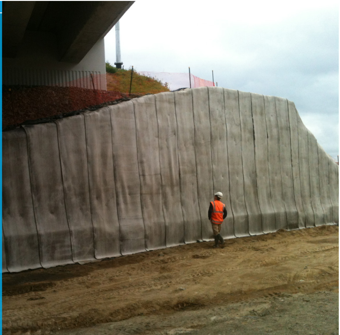
Completed section of slope lined with CC5
