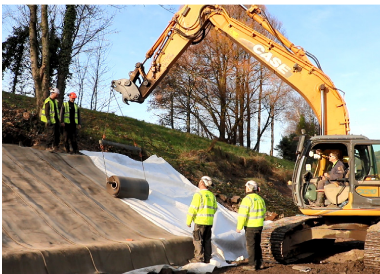
Deployment of CC over the geotextile
