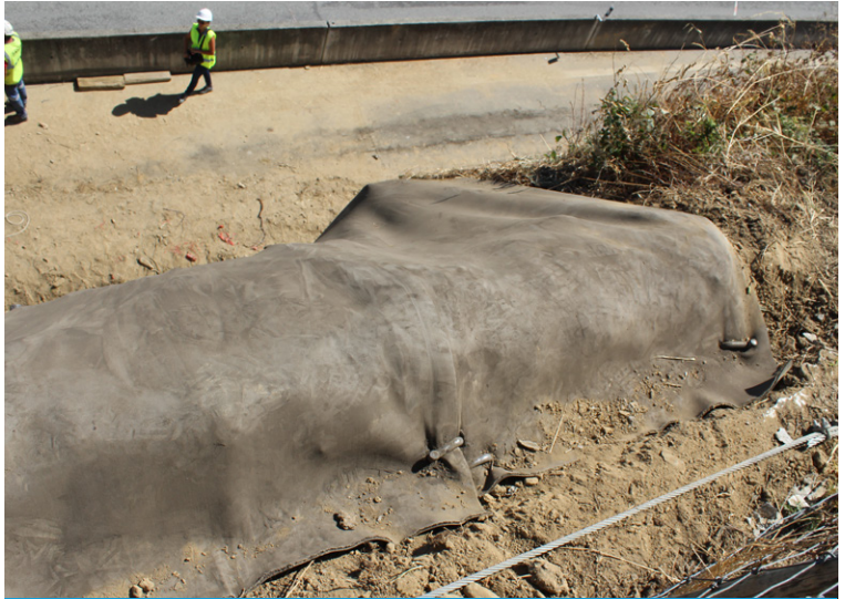
380mm ground pegs were inserted every 1m
