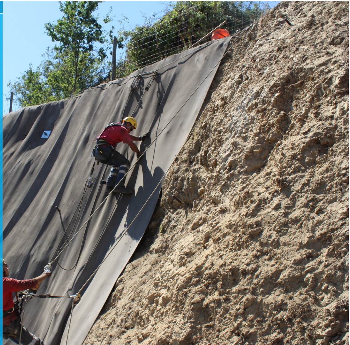
The installation team at Highway A24 had to use climbing equipment due to the restricted access of the site
