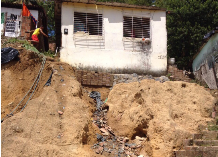
Extensive erosion of the slope
