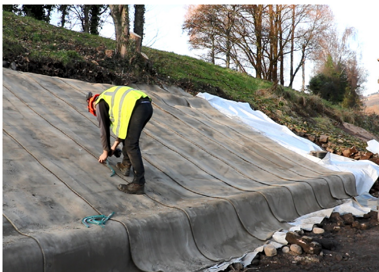
Fixing of the CC layers using screws
