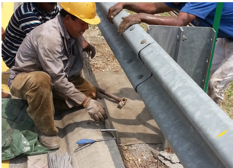
Fixing at the crest with ground pegs
