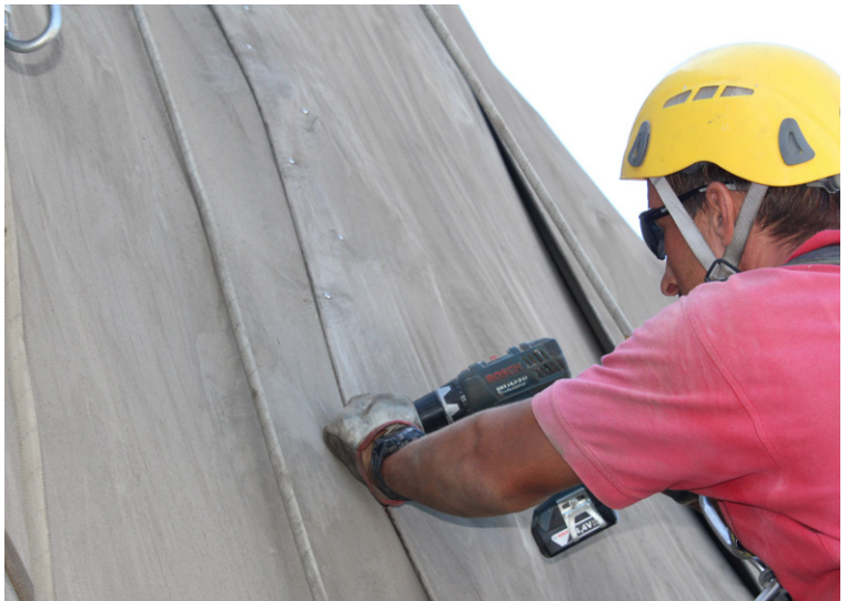
Every other screw was closer to the edge, forming a triangular shape
