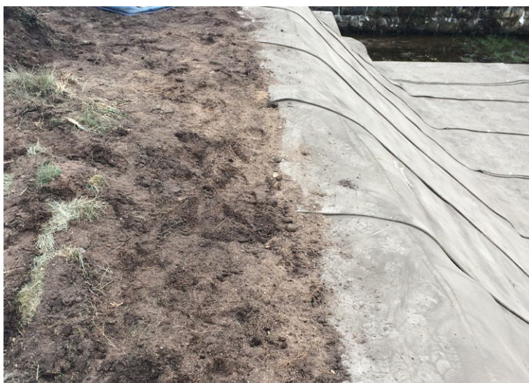
The CC edges were buried in pre-dug anchor trenches
