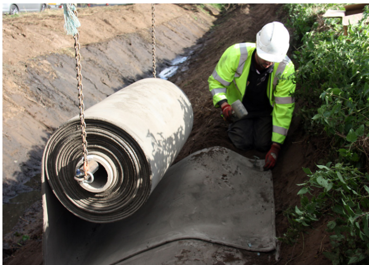
Fixing CC layers to substrate using plastic pins to comply with NG regulations
