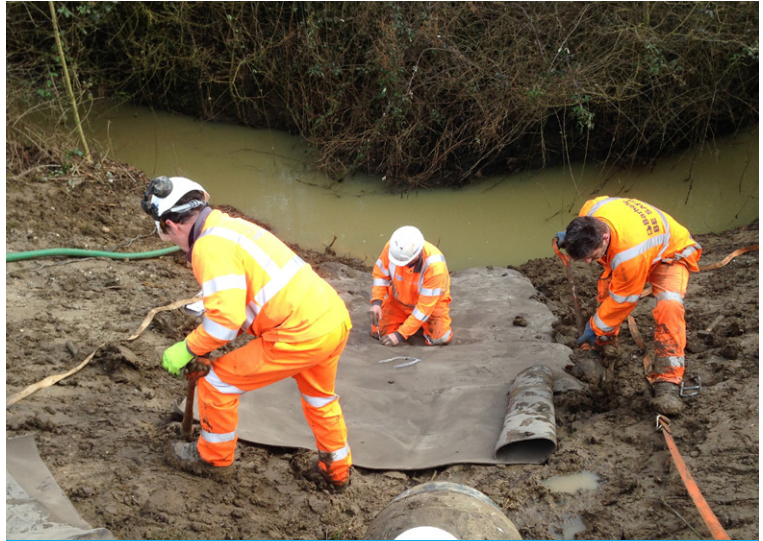
The CC was laid horizontally, working up the slope
