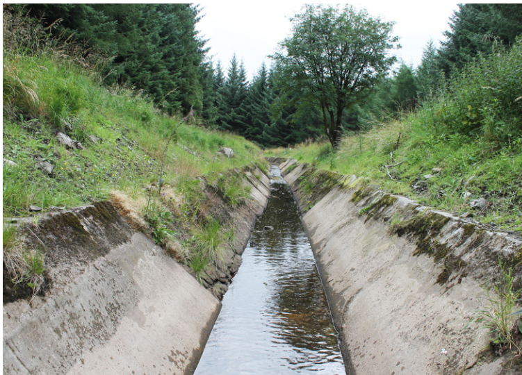
The existing concrete channel was damaged and overgrown
