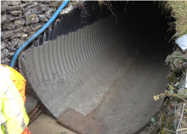
Semi-dry grout was applied to fill in the corrugations in the ARMCO pipe
