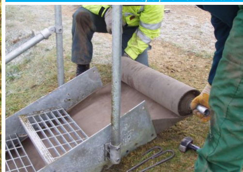
The batched CC was unrolled underneath the steps
