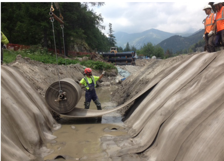
Deployment of CC5 bulk rolls via spreader beam equipment
