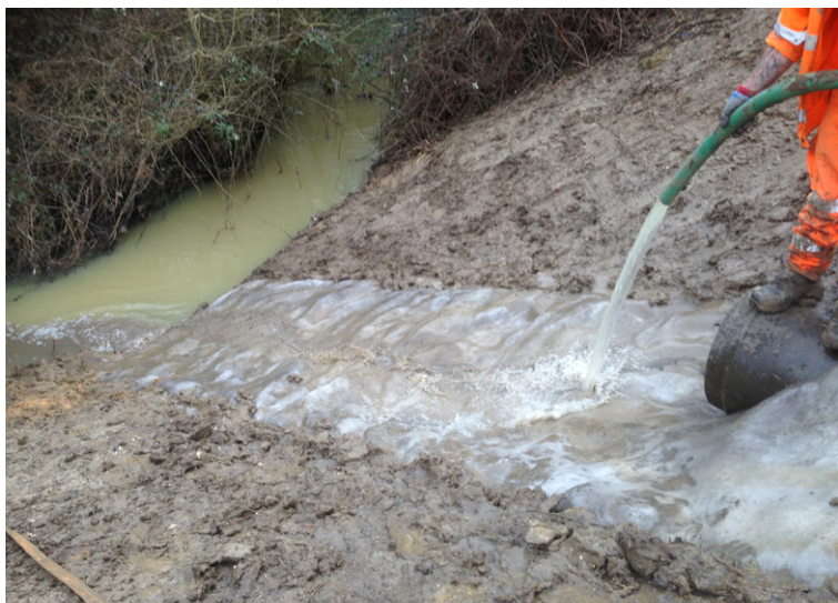
Hydration of the CC from local water course
