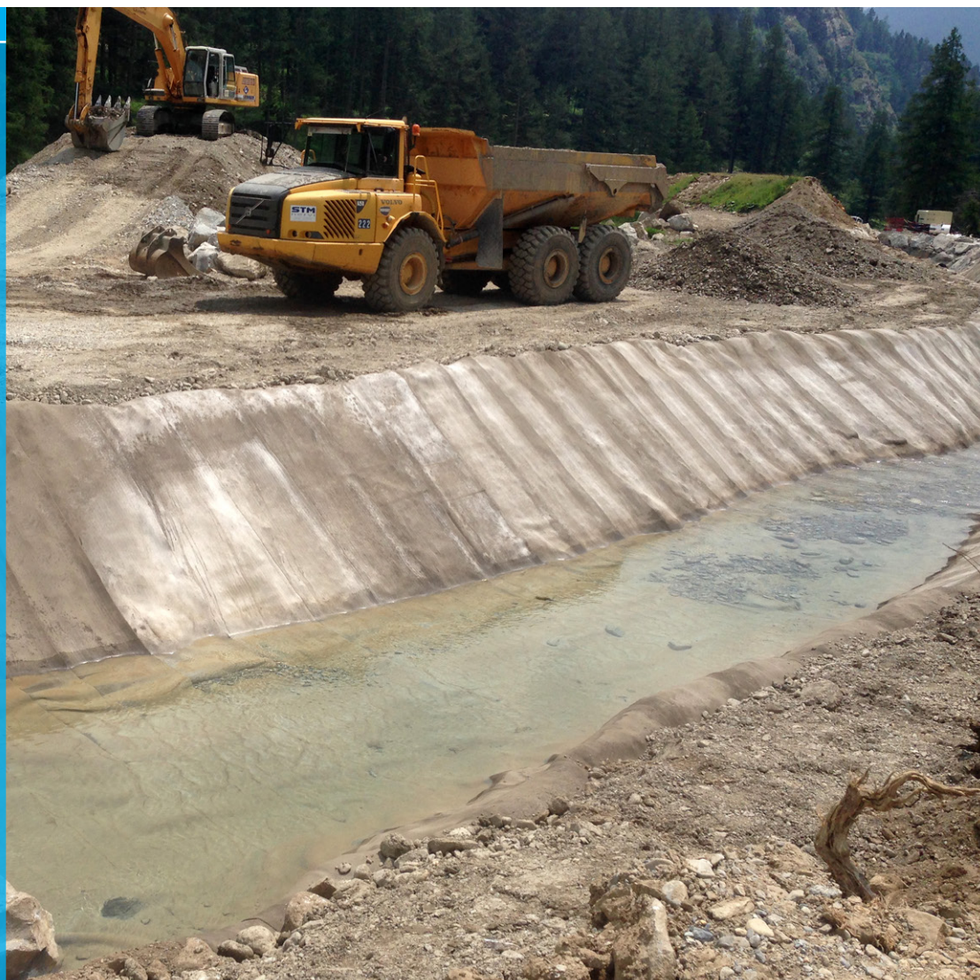
CC lined diversion bank showing stages of hydration
