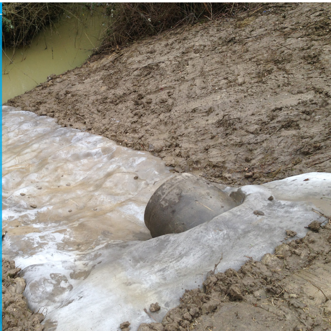
Completed Concrete Canvas scour protection
