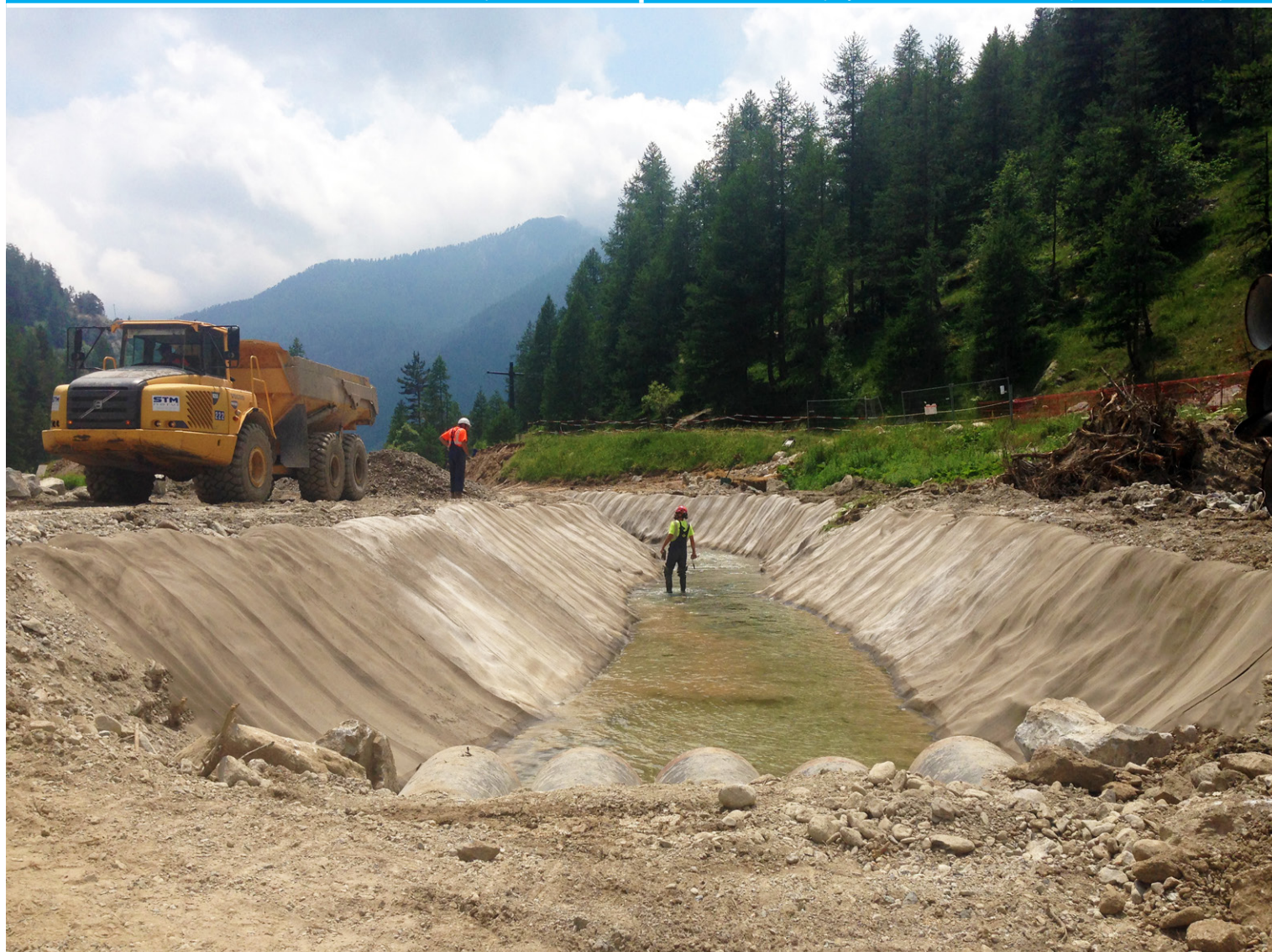
Completed lined diversion.
