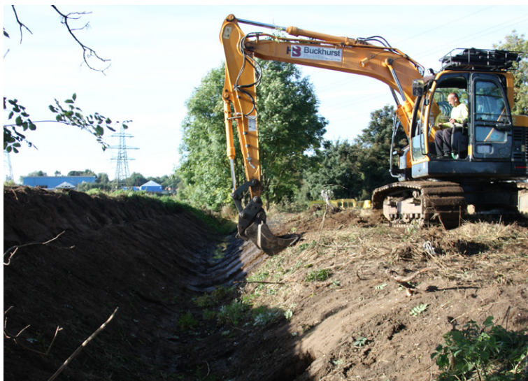
Profiling of the channel via plant machinery
