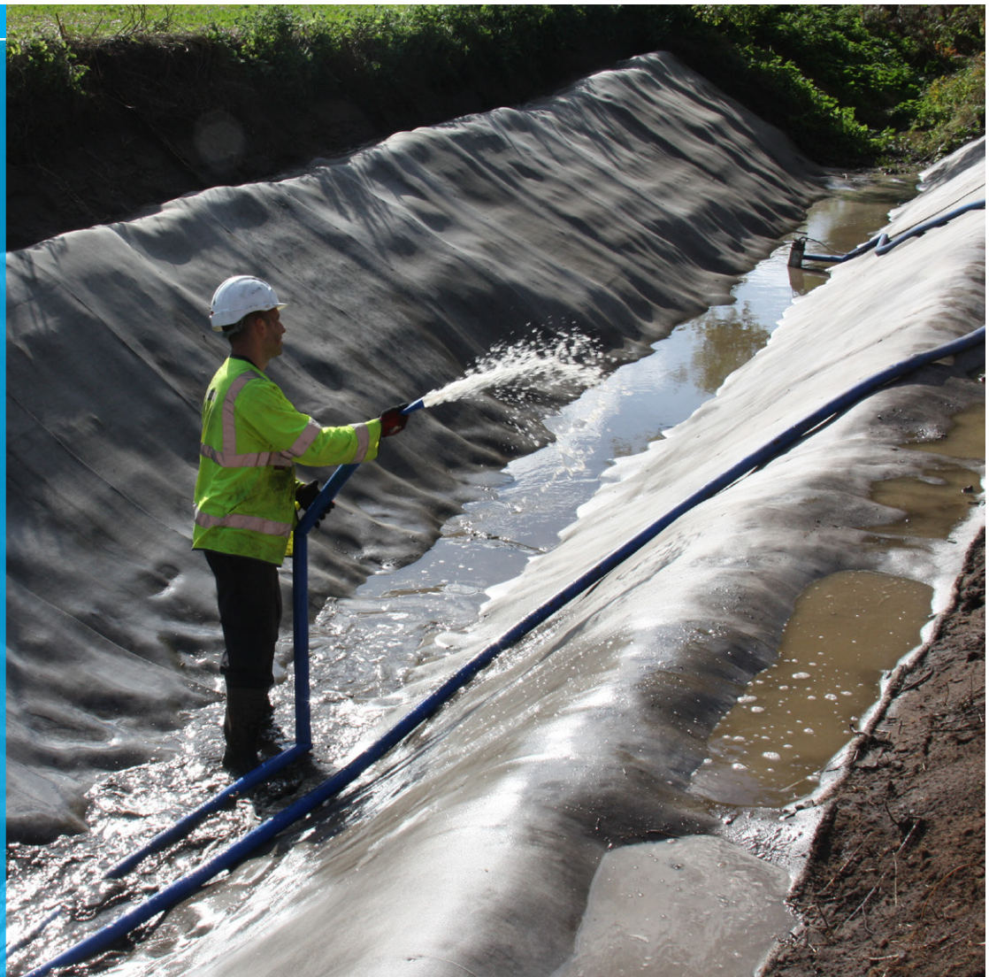
The objective was to provide a rapid method of protective cover to a National Grid key gas main
