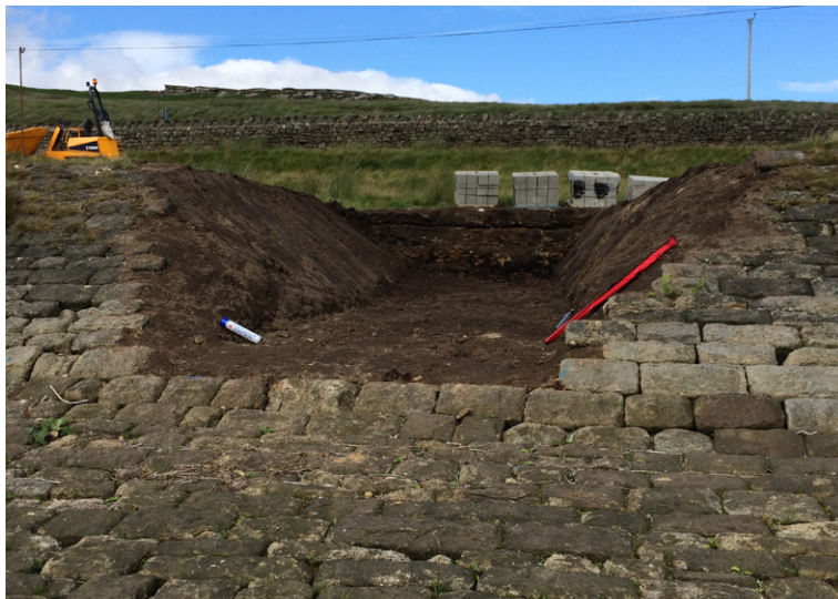
The channel was excavated before installation began
