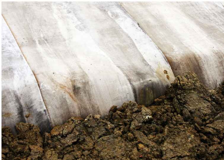
Anchor trench at the toe of the bank
