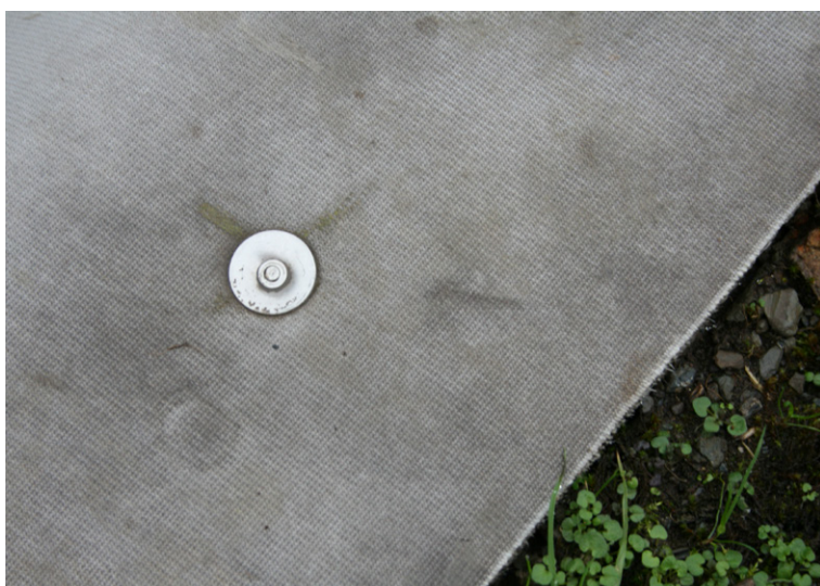
Hilti screws and washers were used to fix the CC to the concrete
