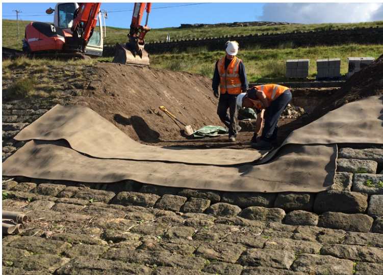
The CC was laid transversely
