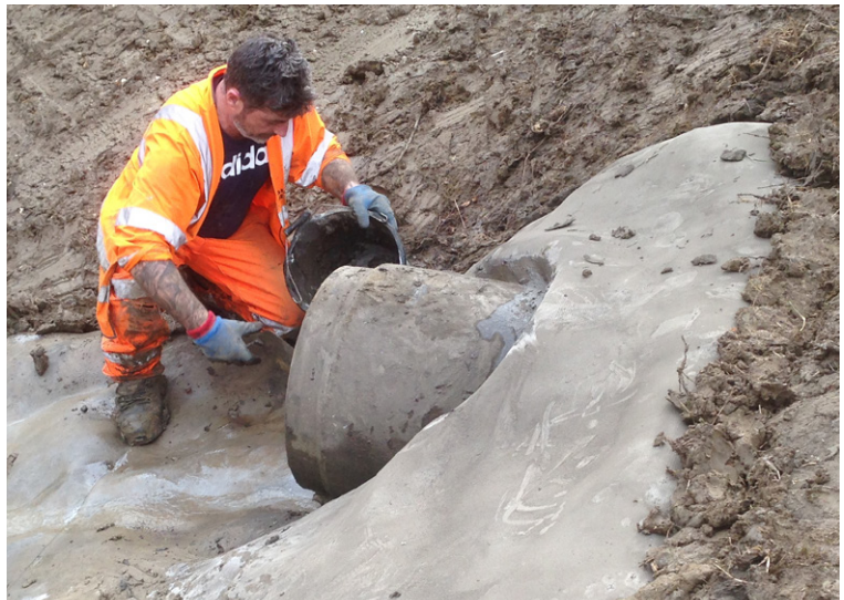
Grout was used to seal the CC around the existing pipe
