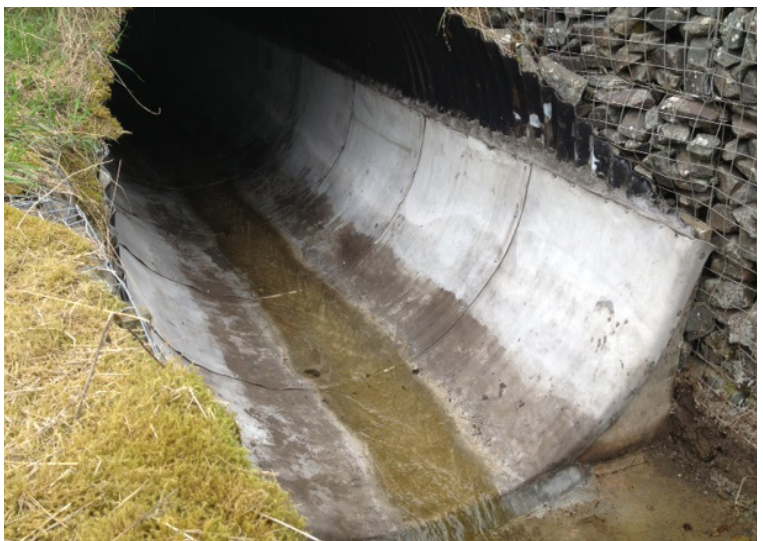
Relined culvert section
