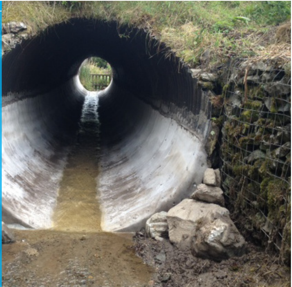
Completed culvert installation
