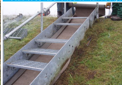
The CC was fixed using screws and hydrated
