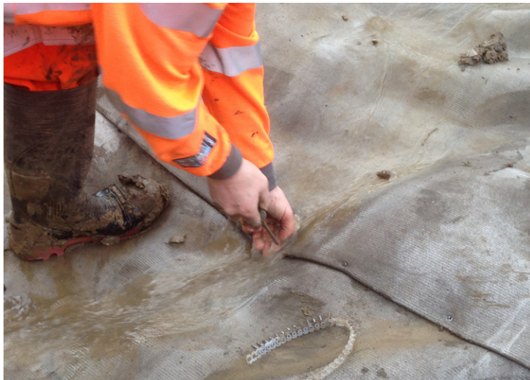
The CC was fixed along the overlaps using screws
