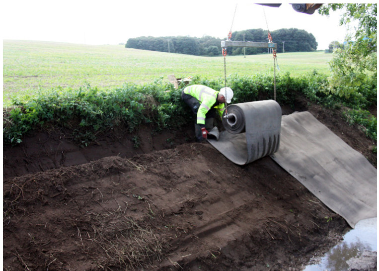
CC bulk rolls deployed via spreader beam, transversely across channel
