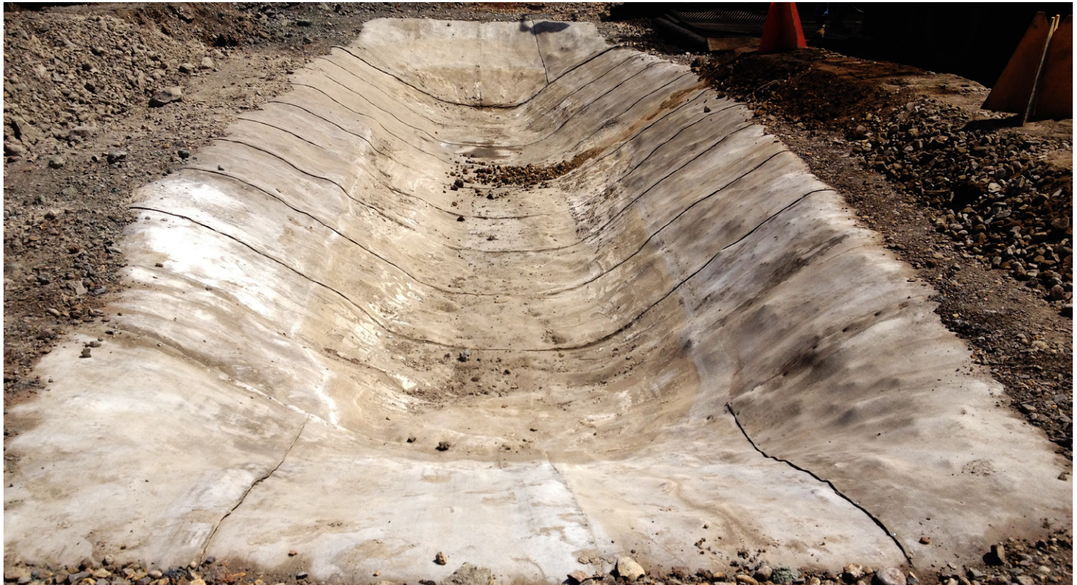
Completed diesel containment pit
