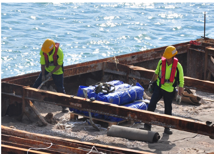
The batched CC was pre-cut to required lengths
