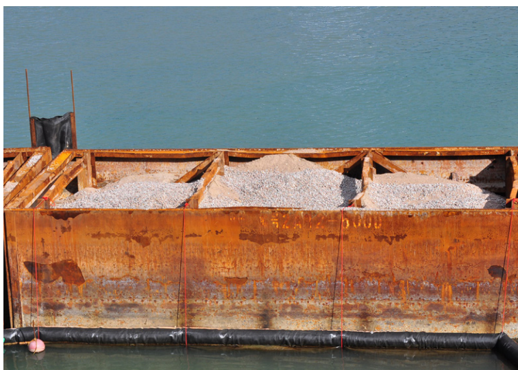
The rockfill material used to fill the steel boxes
