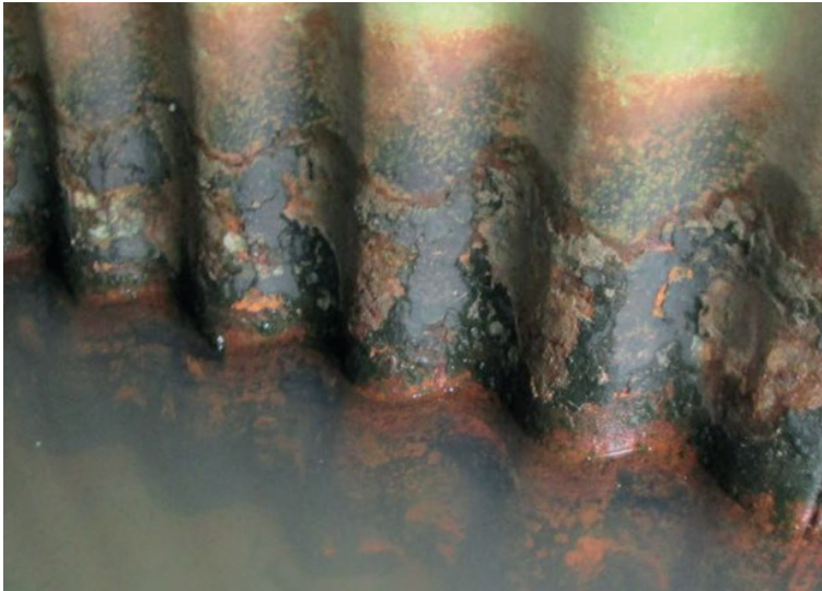
Silt build up and corrosion of culvert floor
