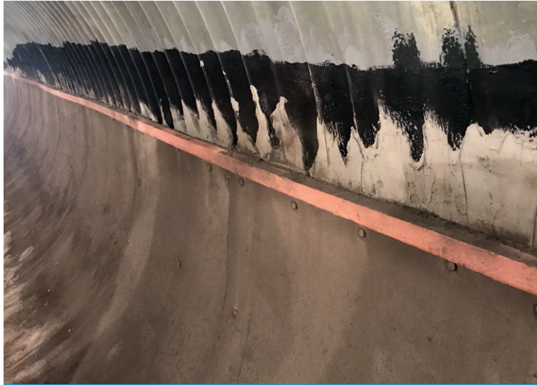
Wood bar fitted to secure CC edges and provide cutting guide for termination
