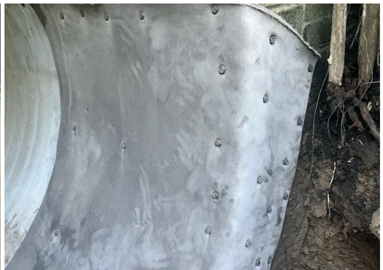
Fixing of first CC length to culvert and outside wall
