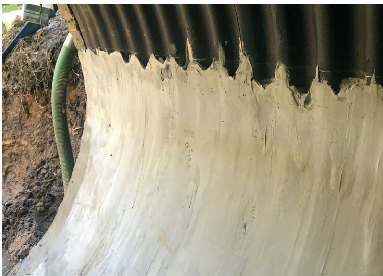
Inverts filled with concrete mortar
