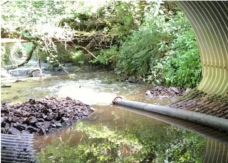
And water redirected using overpumping
