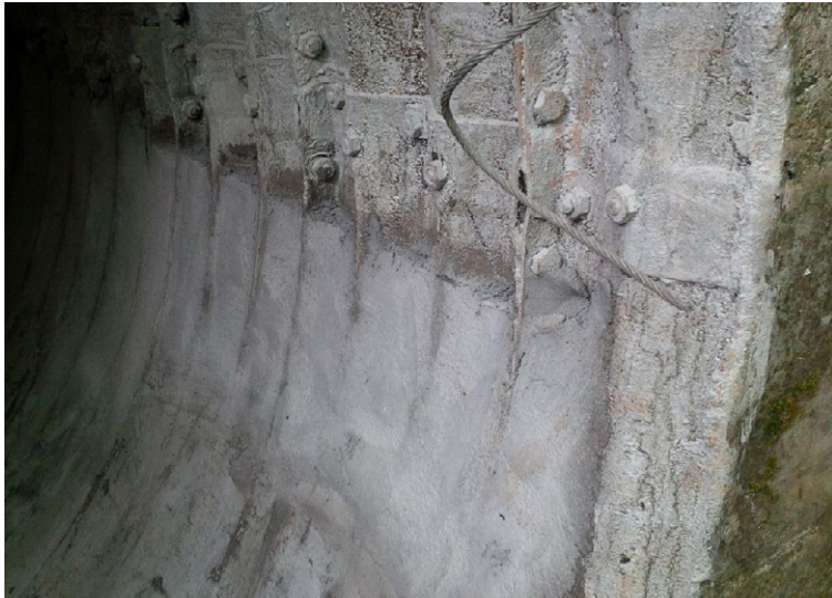
Grout applied to corrugated section
