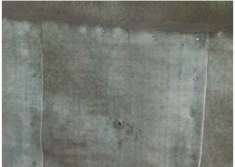
Overlaps screwed and a grout applied to the top
