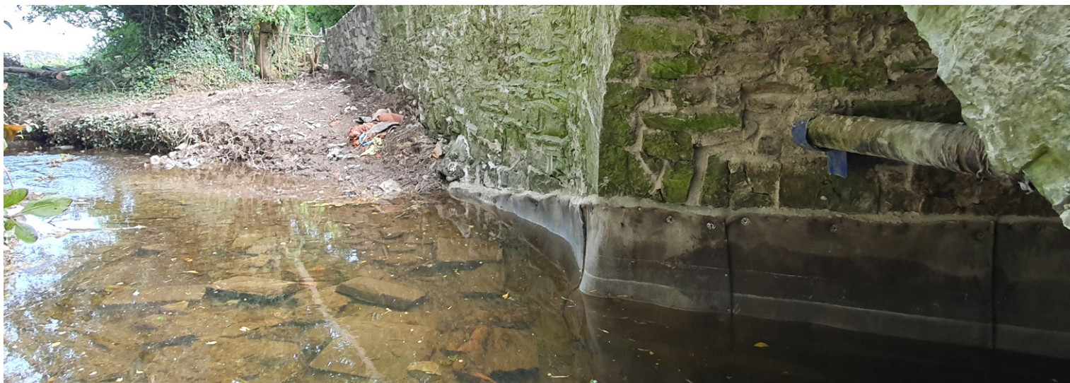
Grout applied to top edge of CC to prevent water ingress
