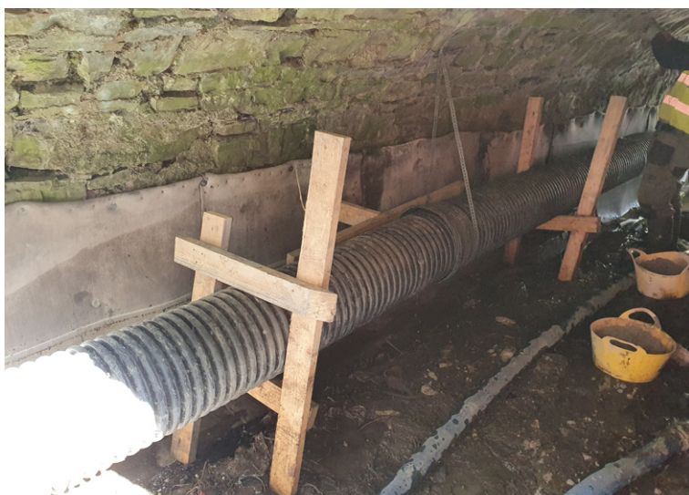
CC laid transversely across culvert with riverbed reinstated in invert
