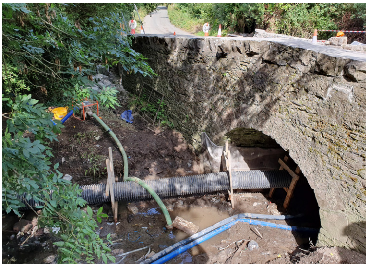
Water overpumped & diverted with HDPE pipe
