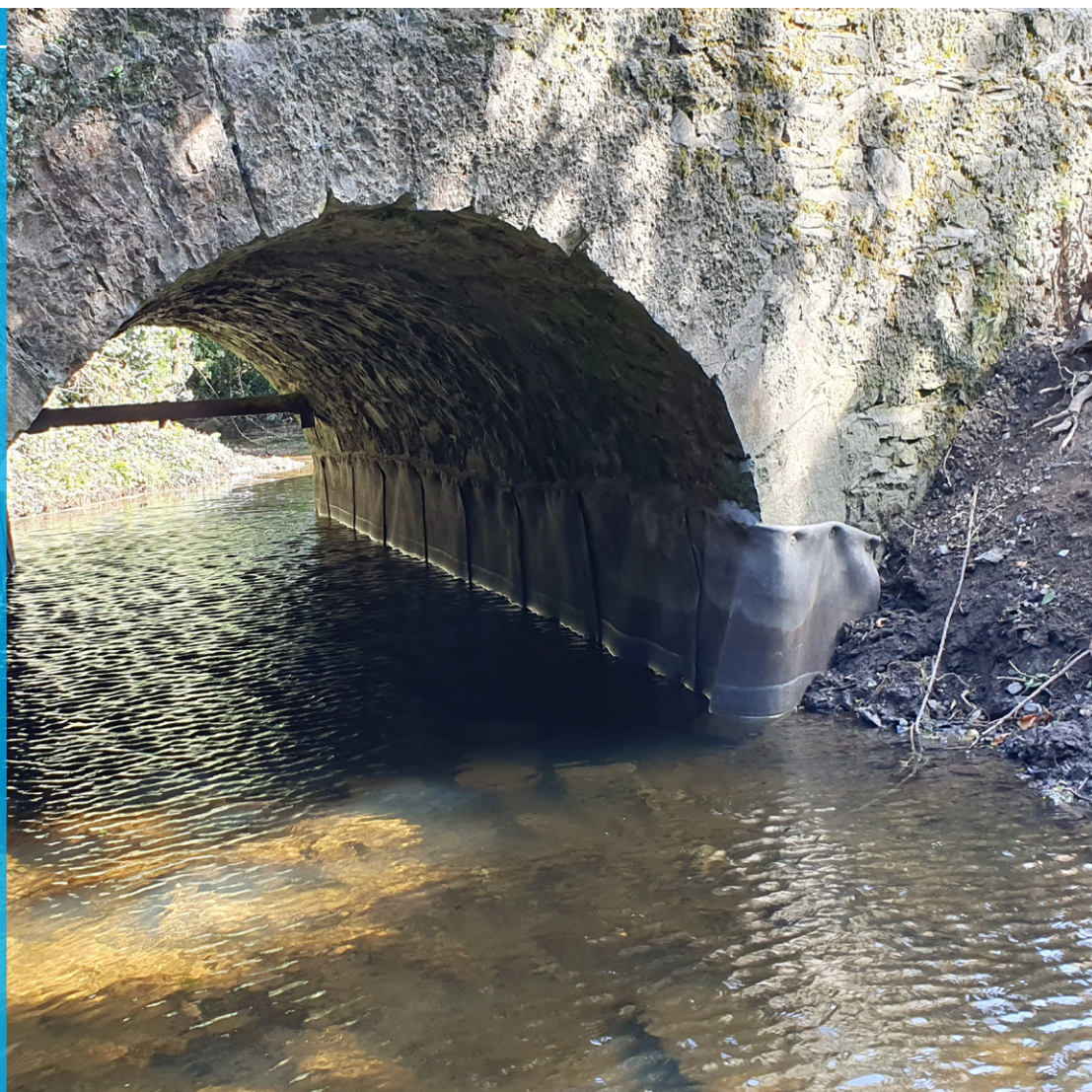
Completed CC culvert lining installation in Dublin
