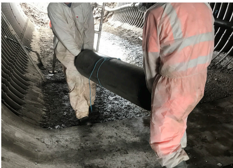
Pre-cut layers transported on side using scaffold pole
