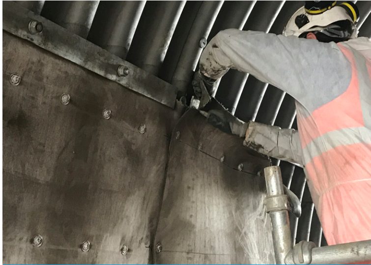
CC edges secured under pre-installed clamp bar supplied by Asset
