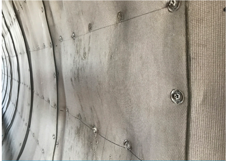
Completed wall section of CC lined culvert
