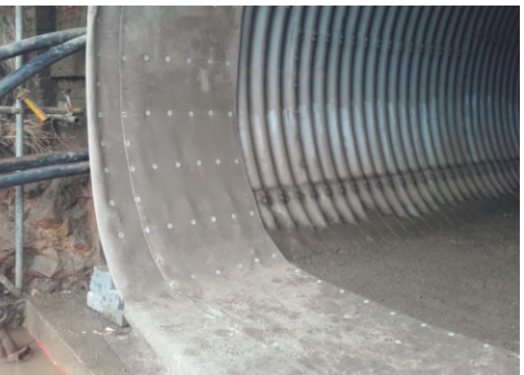
Typical end tie in detail
