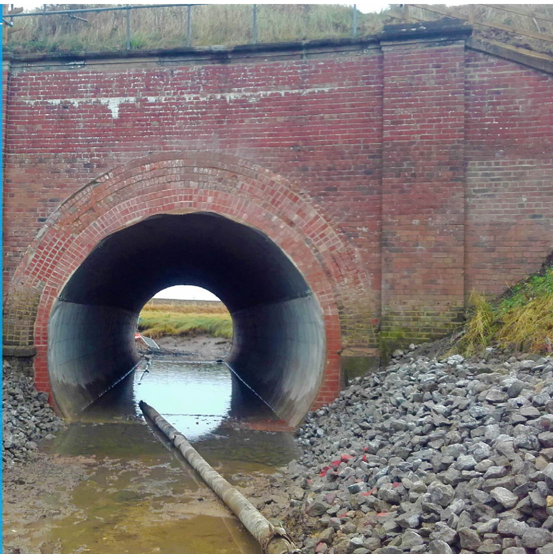
Completed CC-lined culvert structure in Hartlepool
