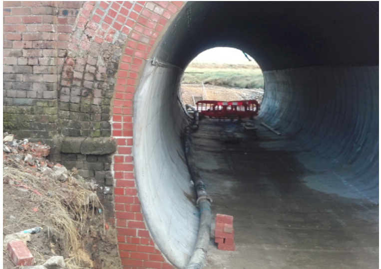
End tie in detail: CC folded around culvert end and sealed with concrete mix
