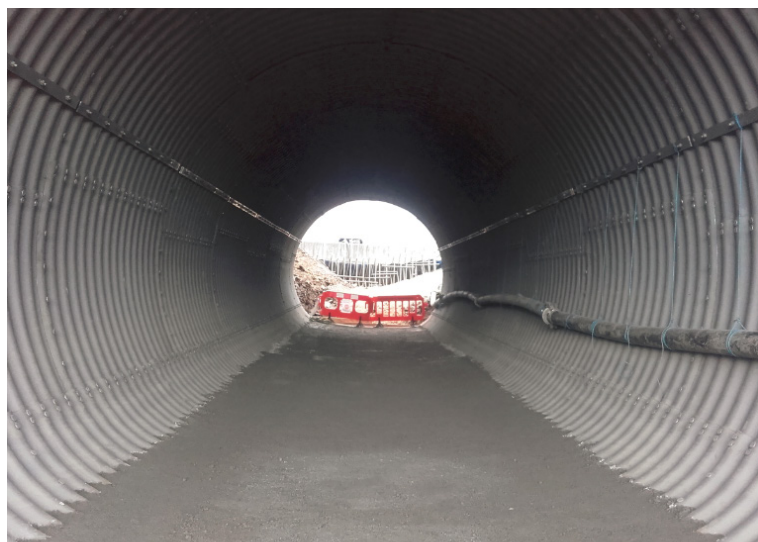
Inverts lined with concrete to support CC
