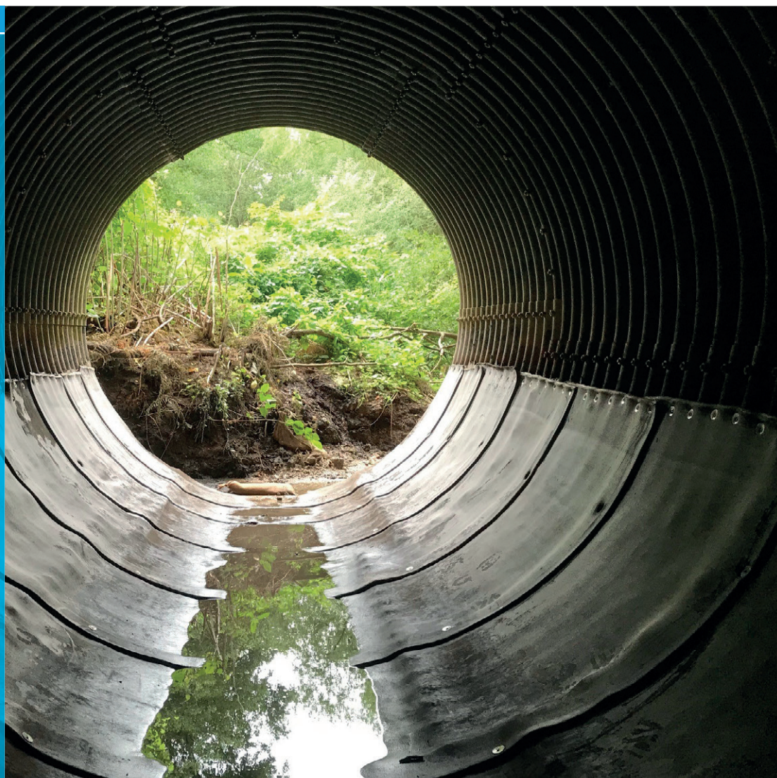
Completed CC culvert lining installation
