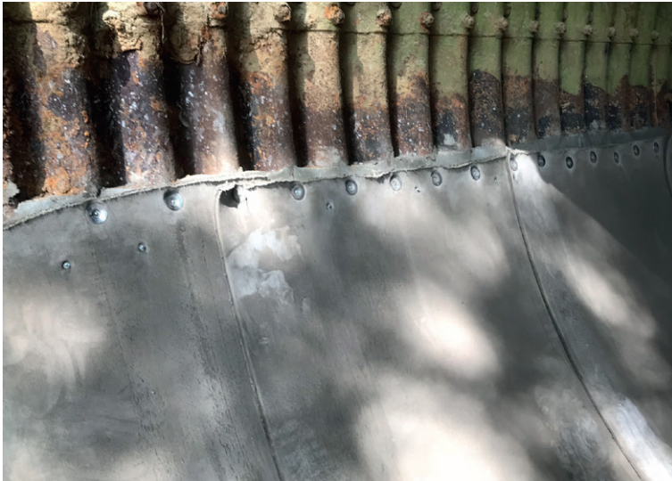
Hilti shot-fired nails used to fix CC to culvert
