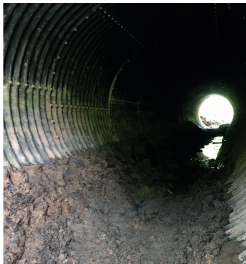
Thick silt build up in culvert 1
