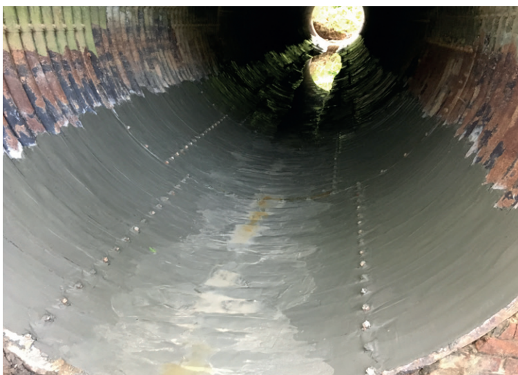
Grout applied to inverts following damming to prevent waterflow
