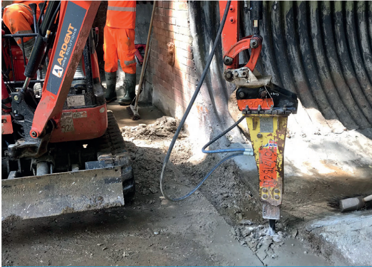
Existing concrete outside culvert removed to create anchor trench
