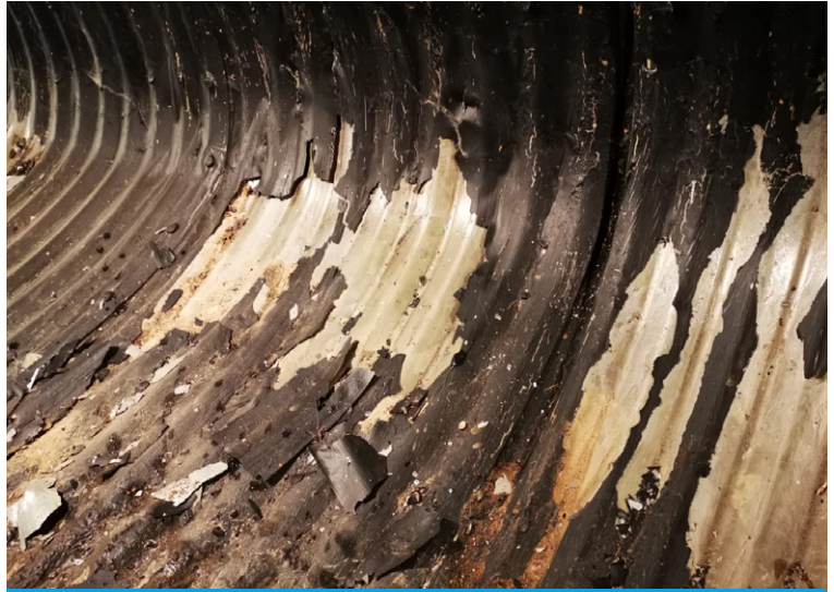
Signs of degradation, rust and flaking of the bitumen coating
