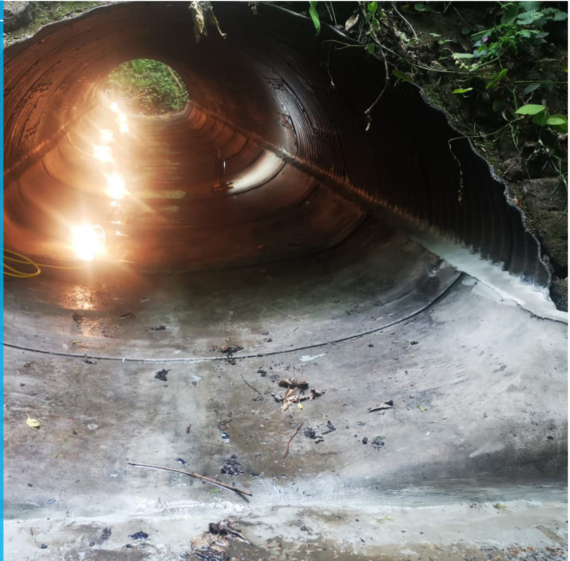
Completed culvert lining installation in Kent, England
