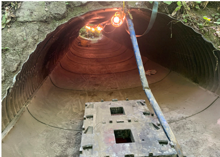
Batched rolls of CC were transported through the culvert on a trolley
