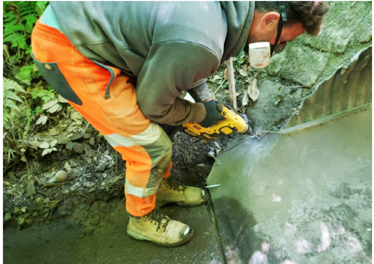
CC attached to masonry exterior using shot-fired nails
