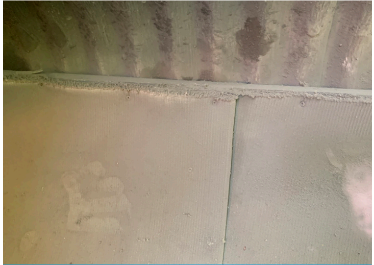
CC edges cut level with wooden batton for neat termination
