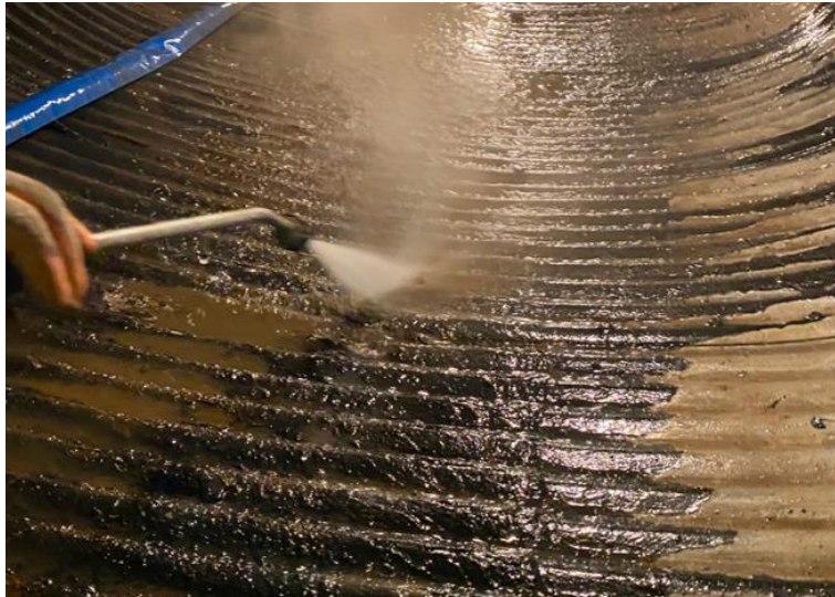
Power hose used to remove bitumen coating, sediment and surface rust
