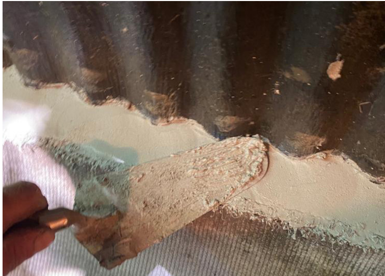
Grout applied around edges to prevent ingress post-hydration
