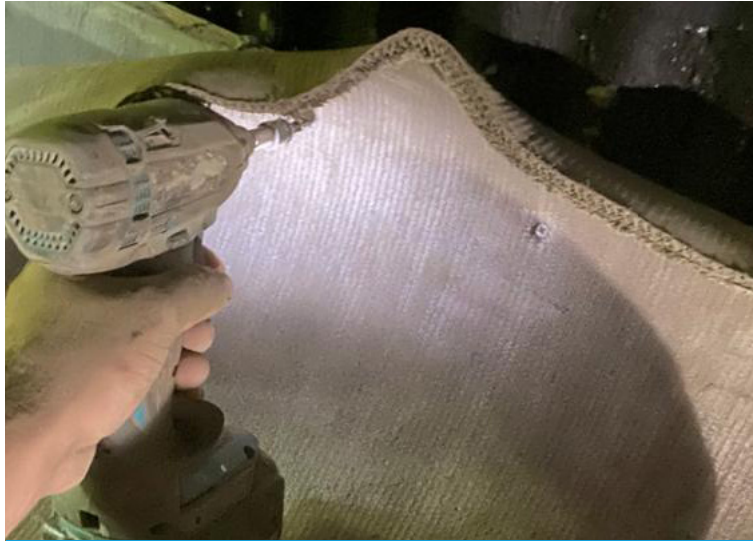
CC attached to wooden battons using stainless steel screws
