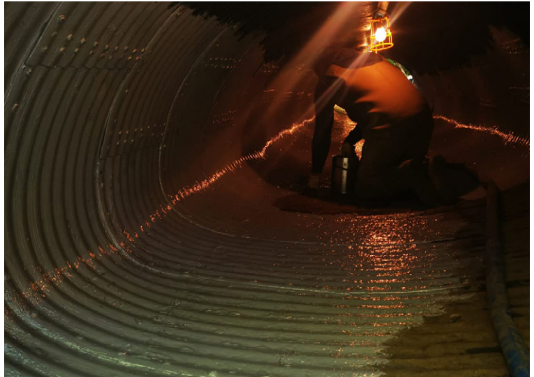
Application of grout to culvert floor and walls
