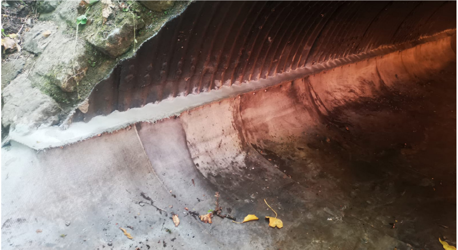
Completed culvert lining installation
