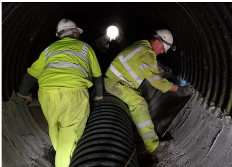
Batched rolls of CC8 were laid transversely across the width of the culvert
