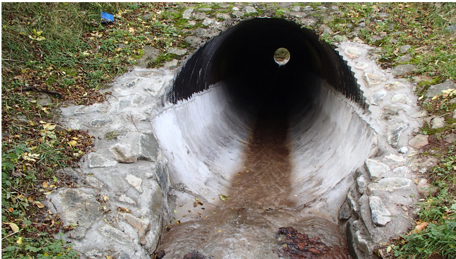
Completed relined culvert on upstream side
