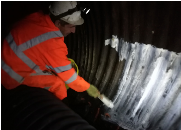
An Everbuild PVA adhesive & bonding agent was applied to crenulations
