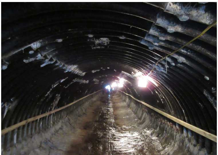
Culvert following preparation works and installation of wooden battens
