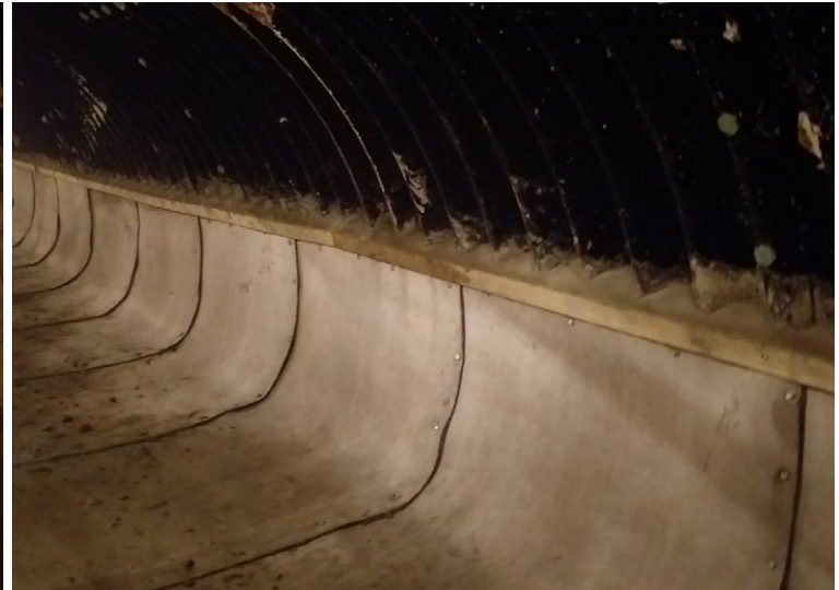
CC laid transversely across culvert floor and secured to walls
