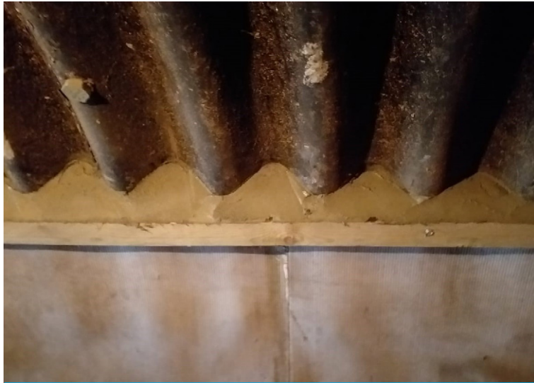
Grout used to fill voids behind material edges to prevent ingress
