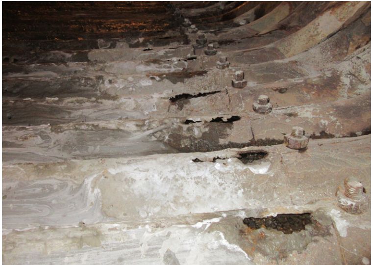
Corroded culvert floor and protruding bolts
