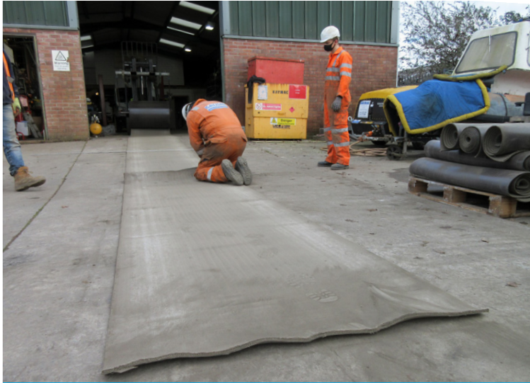
CC batched to required lengths off site
