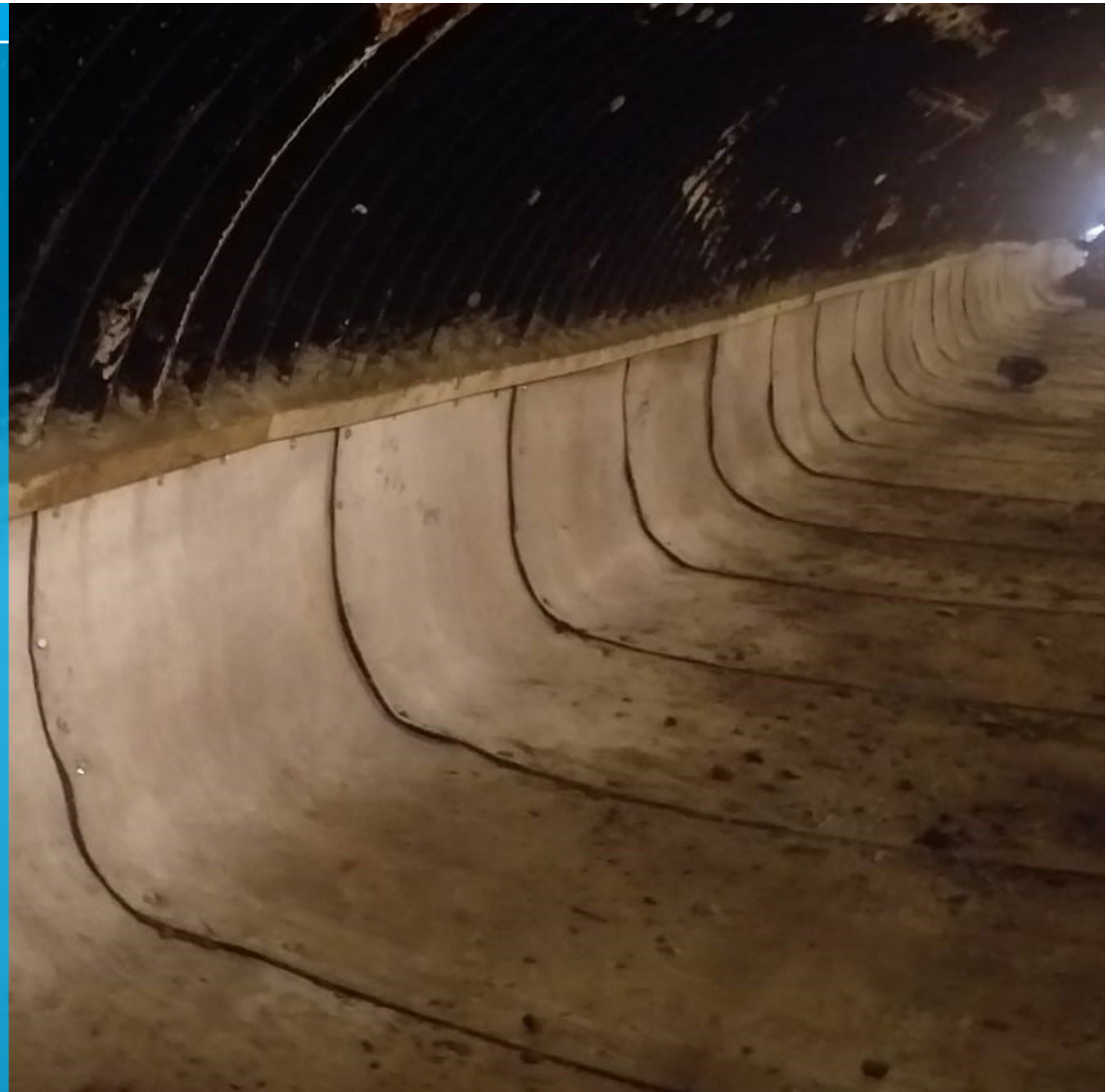
Completed culvert lining project below the M4 near Hendy, Wales
