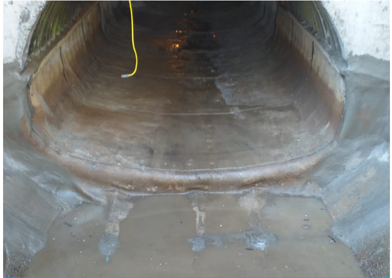
Termination of CC edges outside culvert
