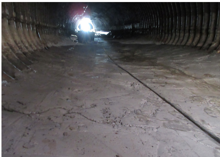
Corrugation inverts filled and floor levelled with grout to cover protruding bolts
