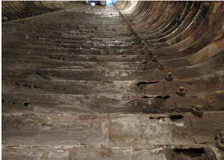
Damaged culvert floor and sediment build up
