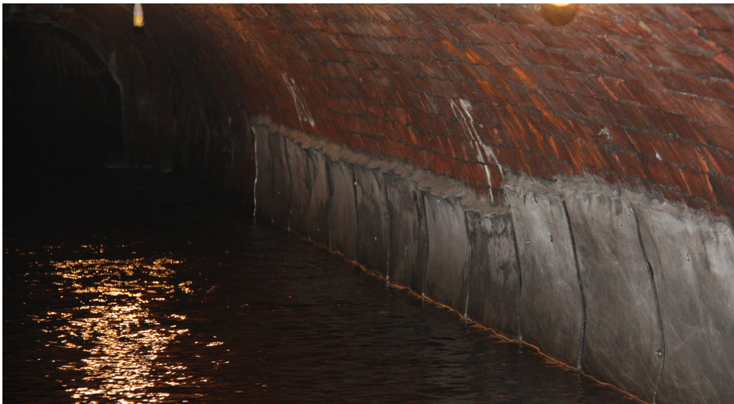
Completed section of CC installation within the culvert below Spencer Court
