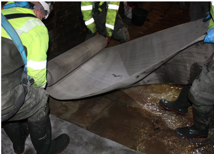
Deploying CC batched roll
