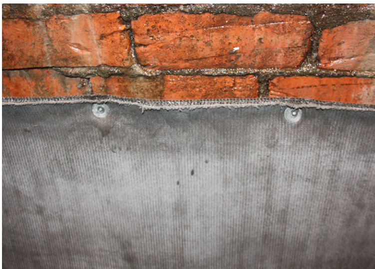
CC edges were trimmed for neat finish
