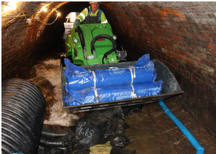
Batched rolls of CC transported through culvert
