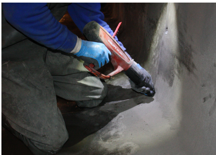
Securing CC to culvert floor
