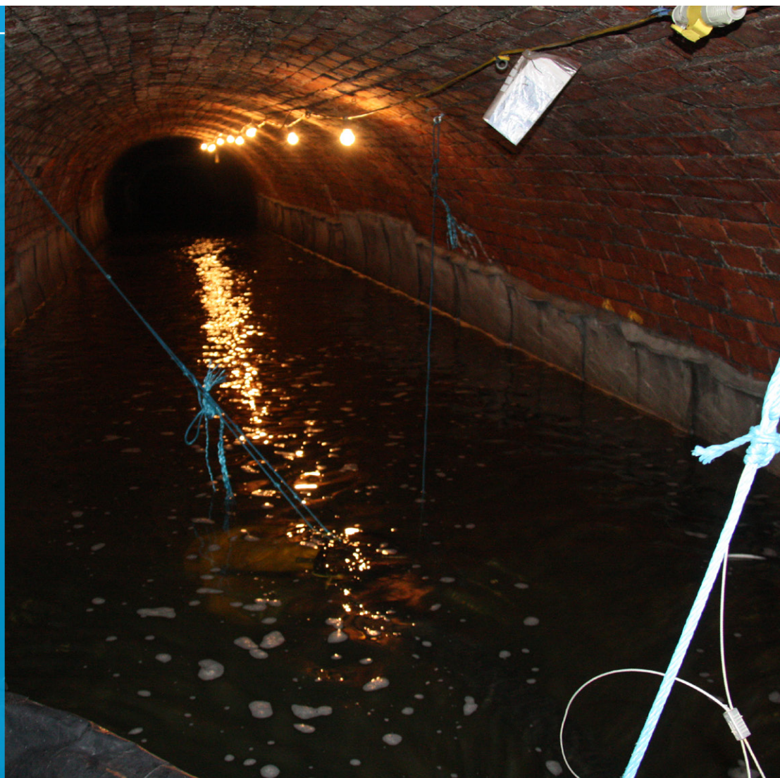
Completed CC installation within Newburn Culvert
