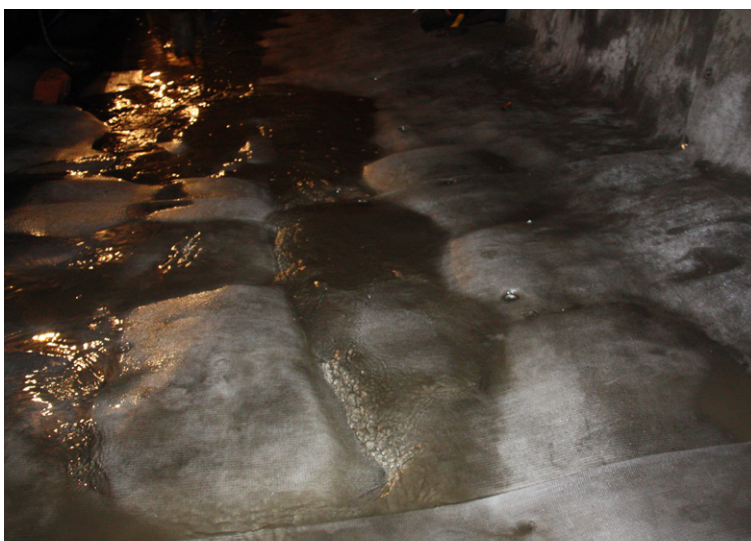
CC easily conformed to the culvert profile
