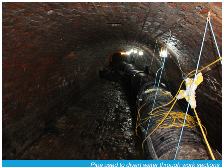
Pipe used to divert water through work sections
