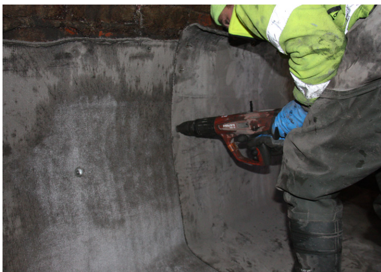
Securing leading edge of CC to culvert wall
