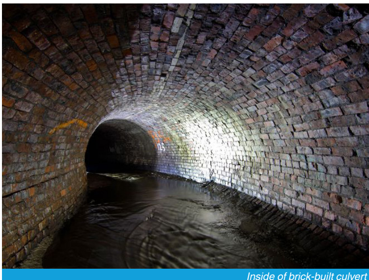
Inside of brick-built culvert
