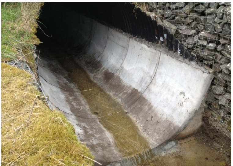
Relined culvert section
