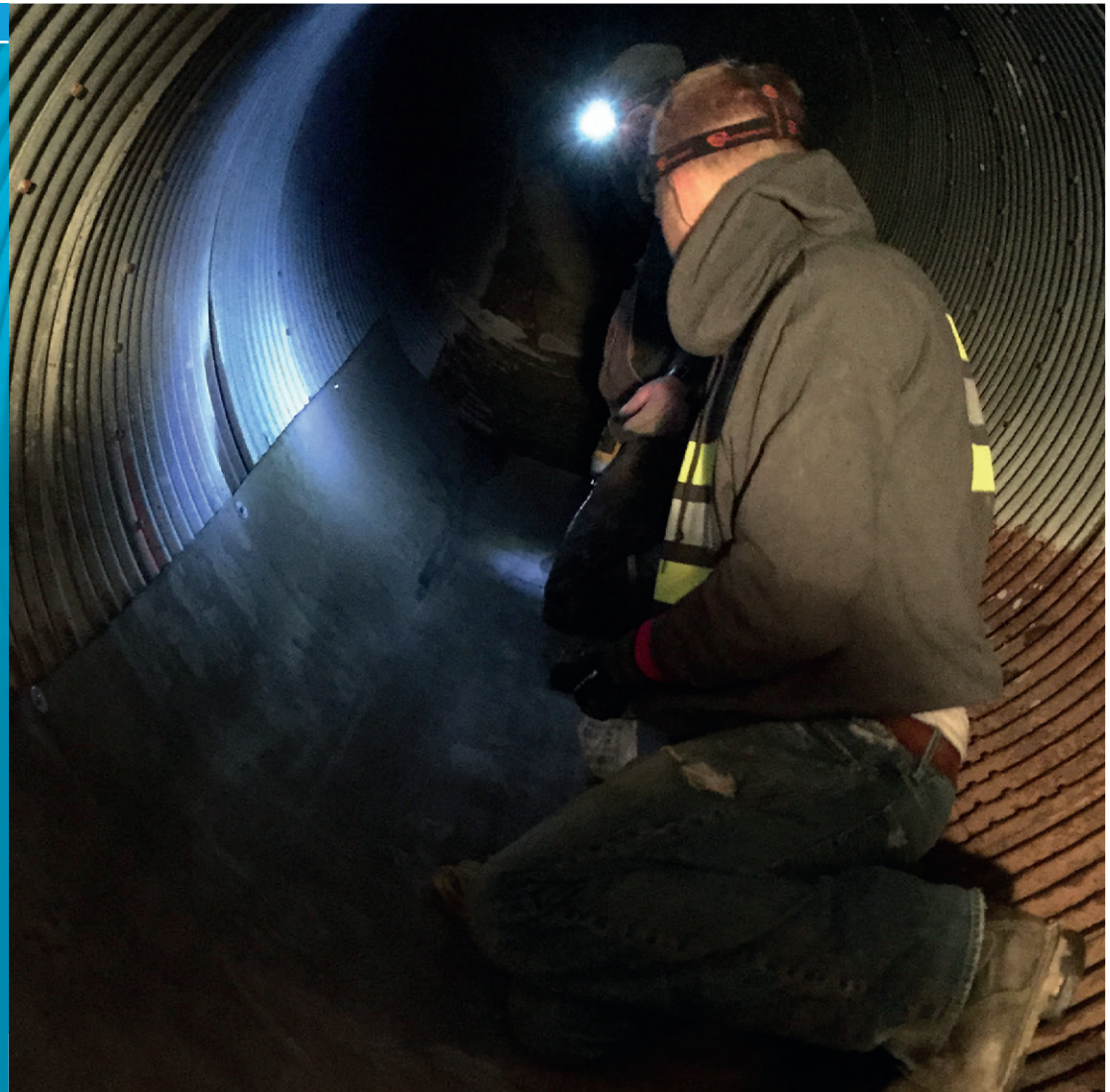
Joining CC layers using self-tapping screws
