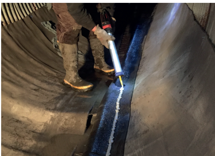
Sealant was used to create a waterproof joint at the overlap of CC layers
