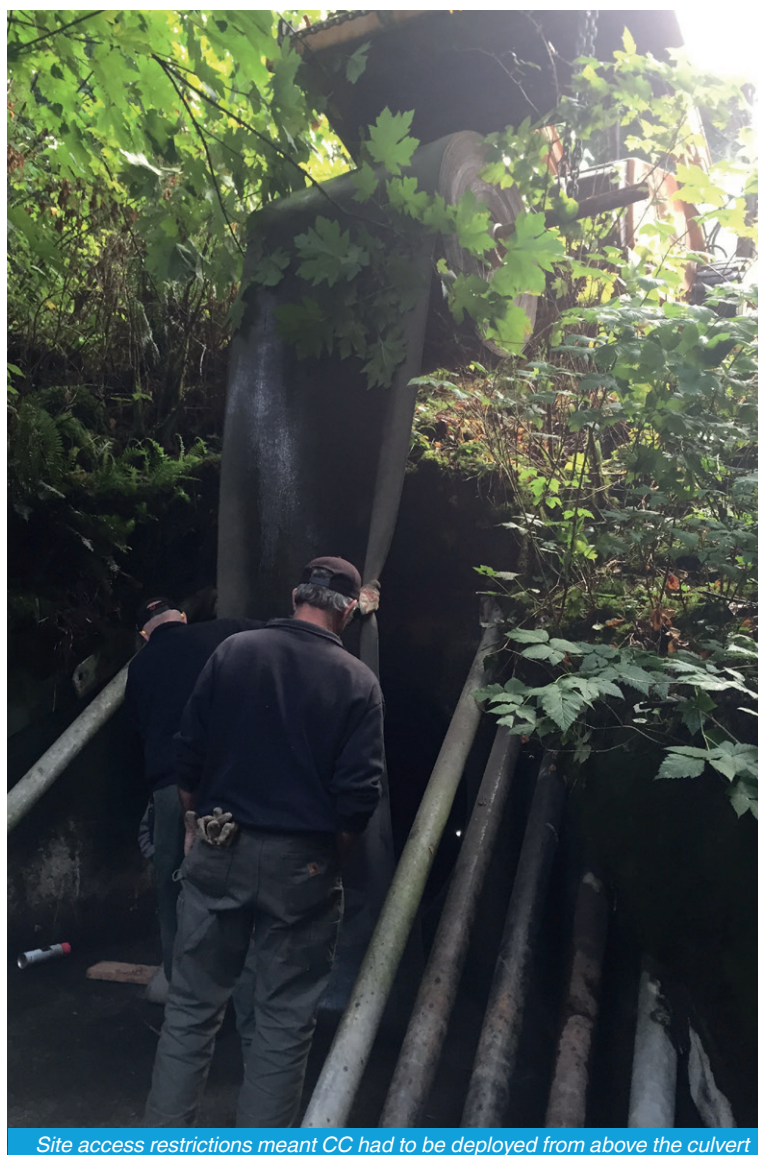
Site access restrictions meant CC had to be deployed from above the culvert
