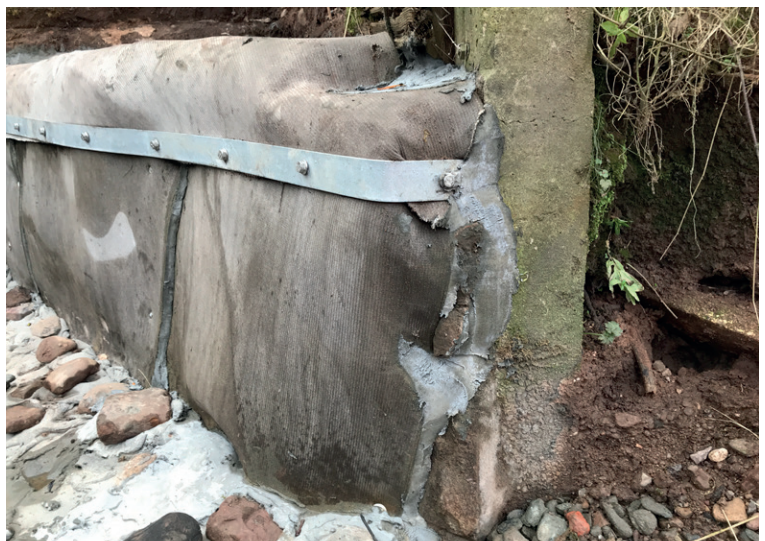
CC edges grouted to prevent ingress at wall
