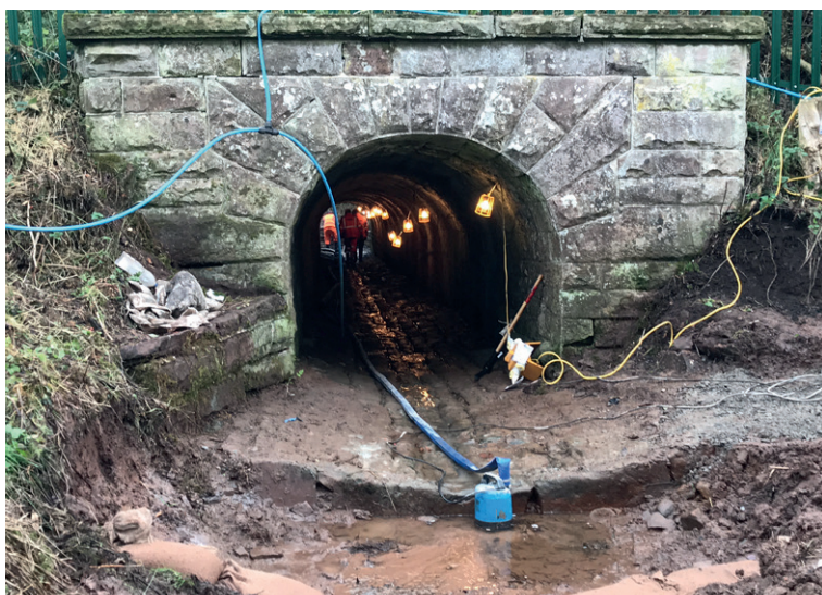
Water overpumped
