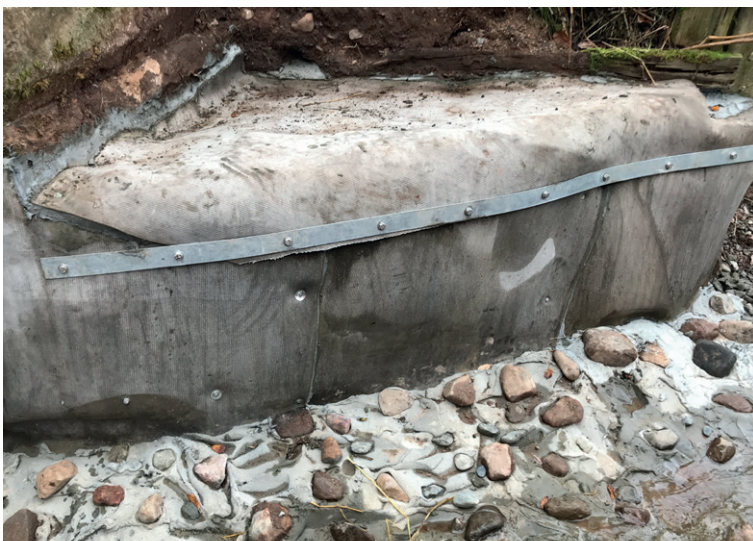
Termination details on wall outside culvert
