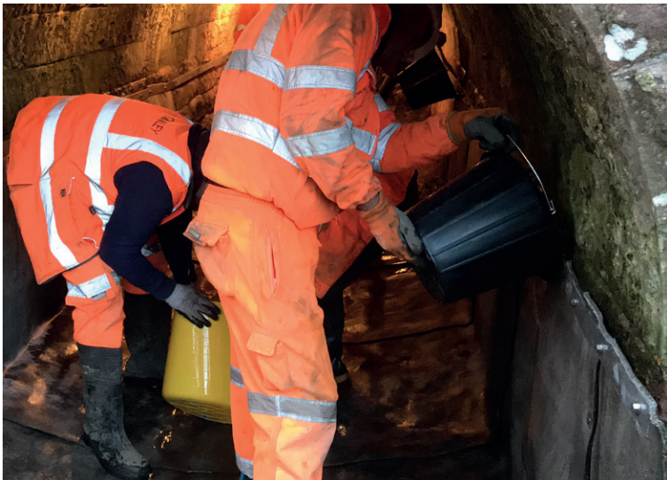
Hydration of CC on walls
