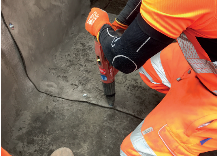
Jointing overlaps using shot-fired nails
