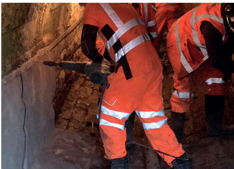
Fixing CC to masonry wall
