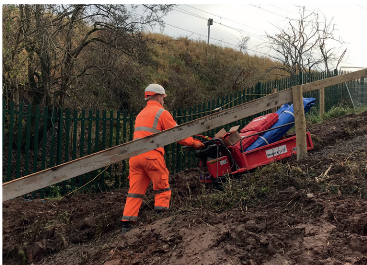
CC batched rolls transported by trolley
