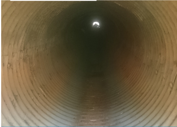
Existing corrugated steel culvert
