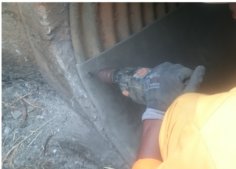
Fixing with pop rivets
