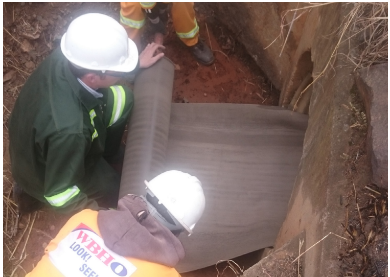
Laying CC5™ lengths in culvert
