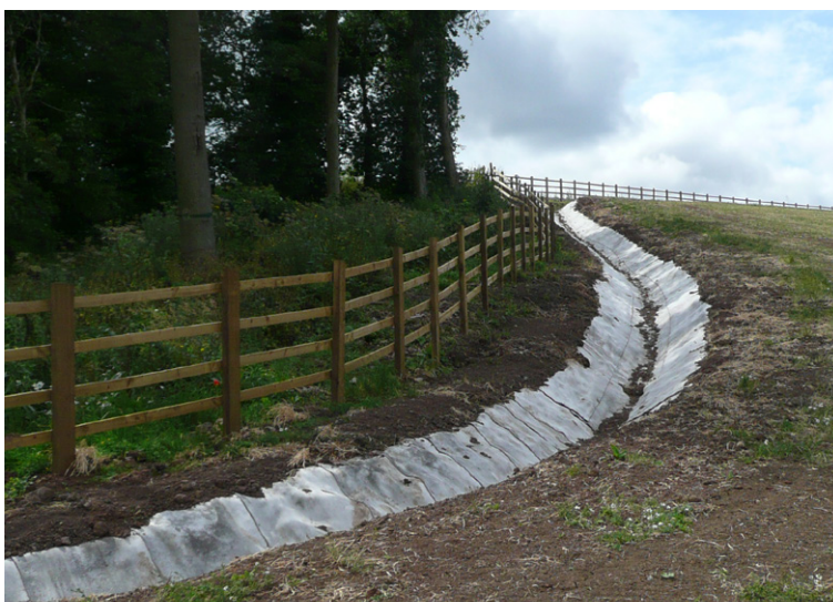
Section of completed channel where transverse layup meets longitudinal layup
