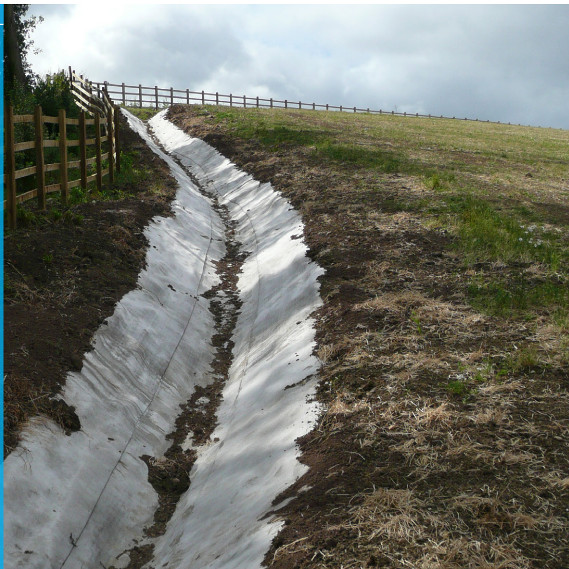
CC lined channel after installation
