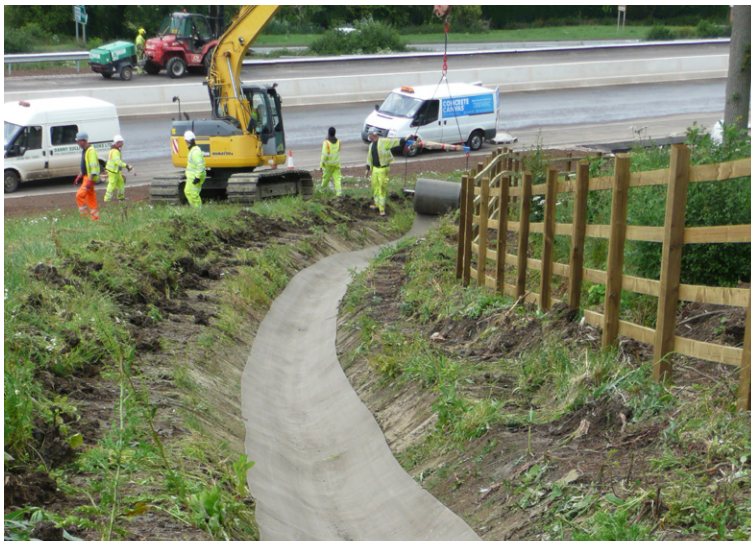
CC8 bulk roll laid from spreader beam for the steep section in 20 mins
