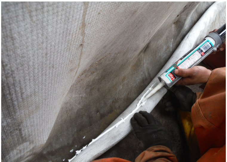
Sealing overlaps using FT 101 sealant
