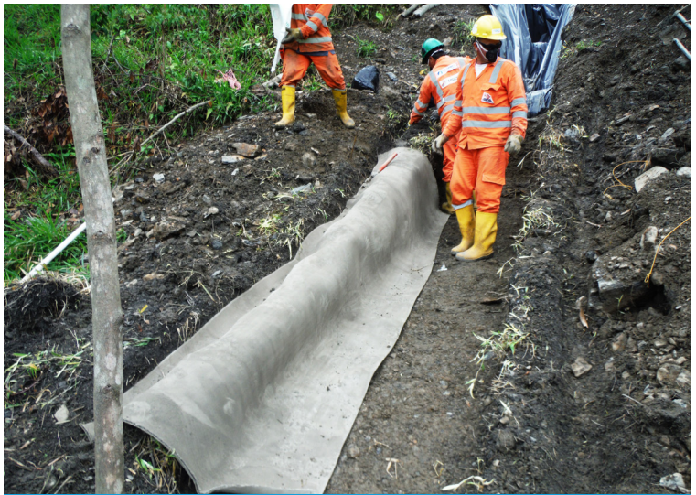
CC laid over the sides of ditch and into an anchor trench
