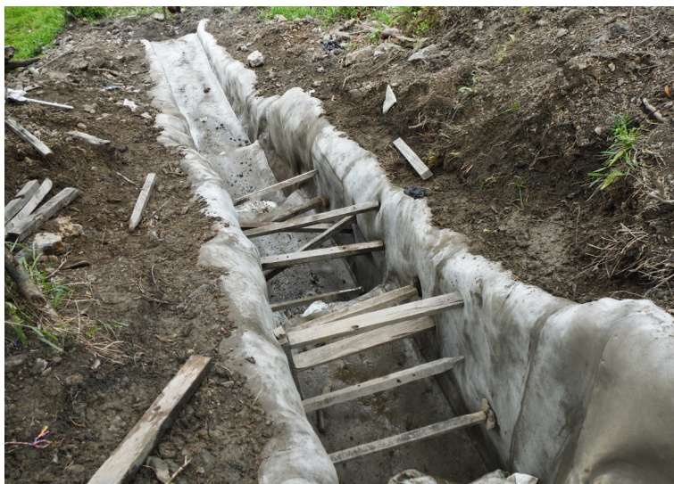
After hydration, planks were used to prevent voids behind the CC
