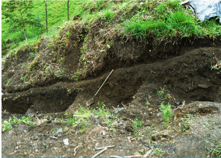
Ditch was excavated and steps introduced
