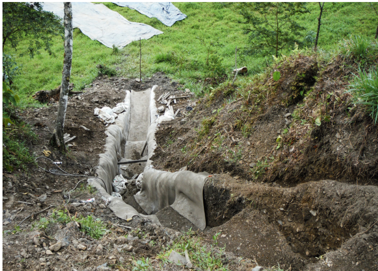
Sides were lined first, then CC applied to ditch base
