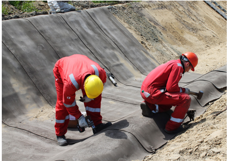
CC8™ sealed, screwed and fixed to the substrate with ground pegs
