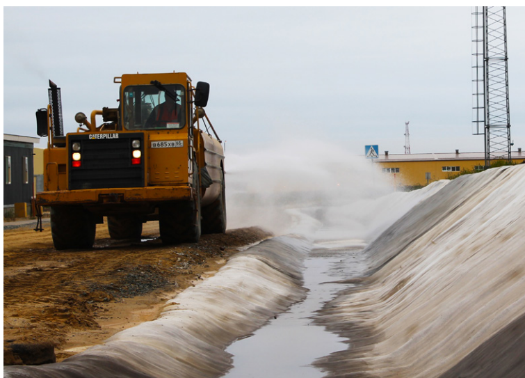
Hydration with a pressure hose from a 7000 litre bowser
