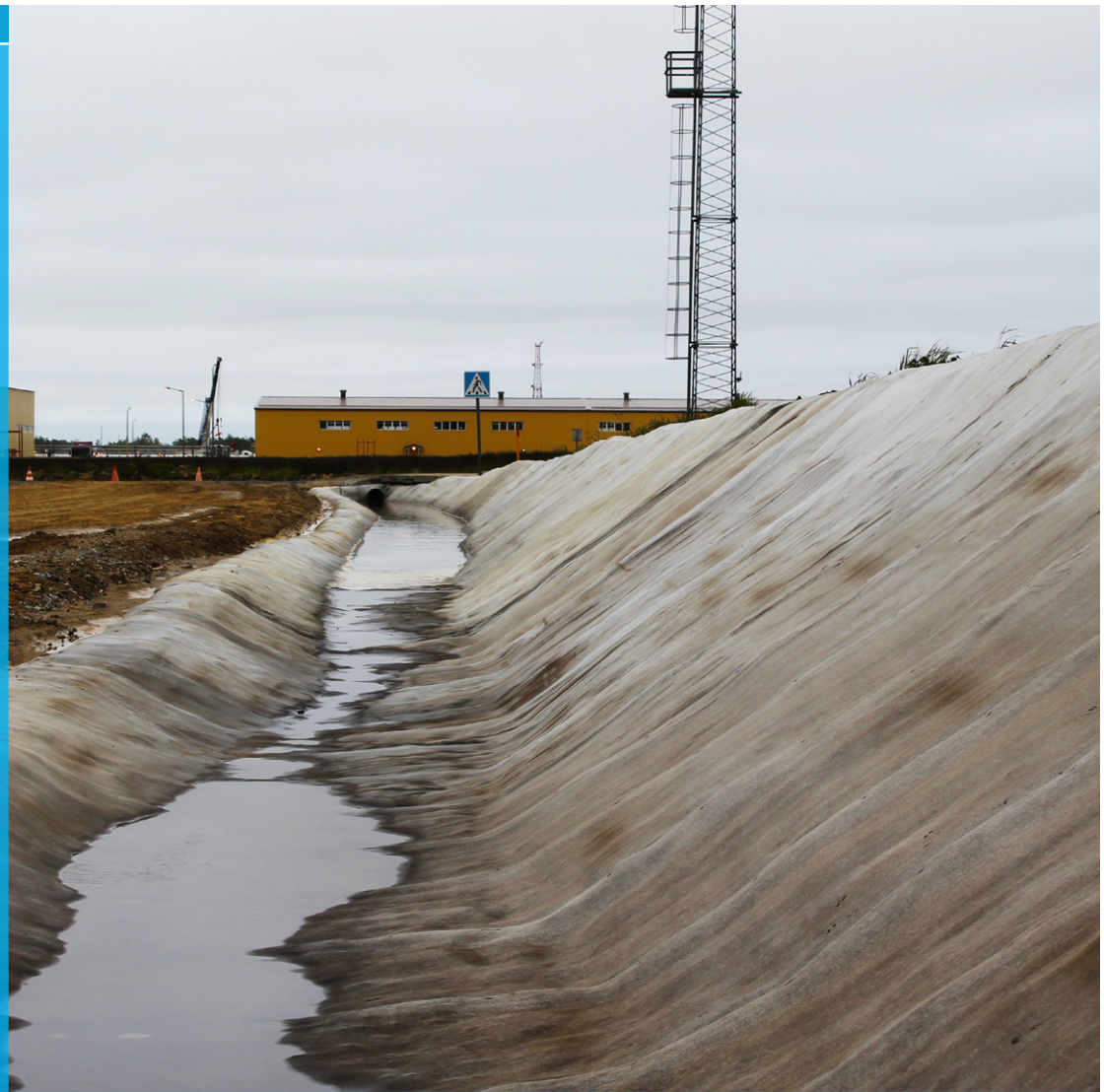
Completed section ditch lined with CC8™
