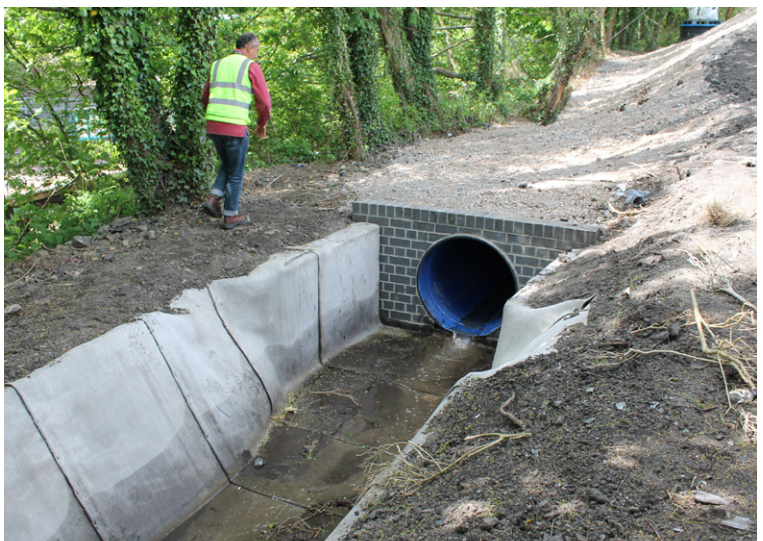
CC was able to be tailored easily around an existing culvert wall
