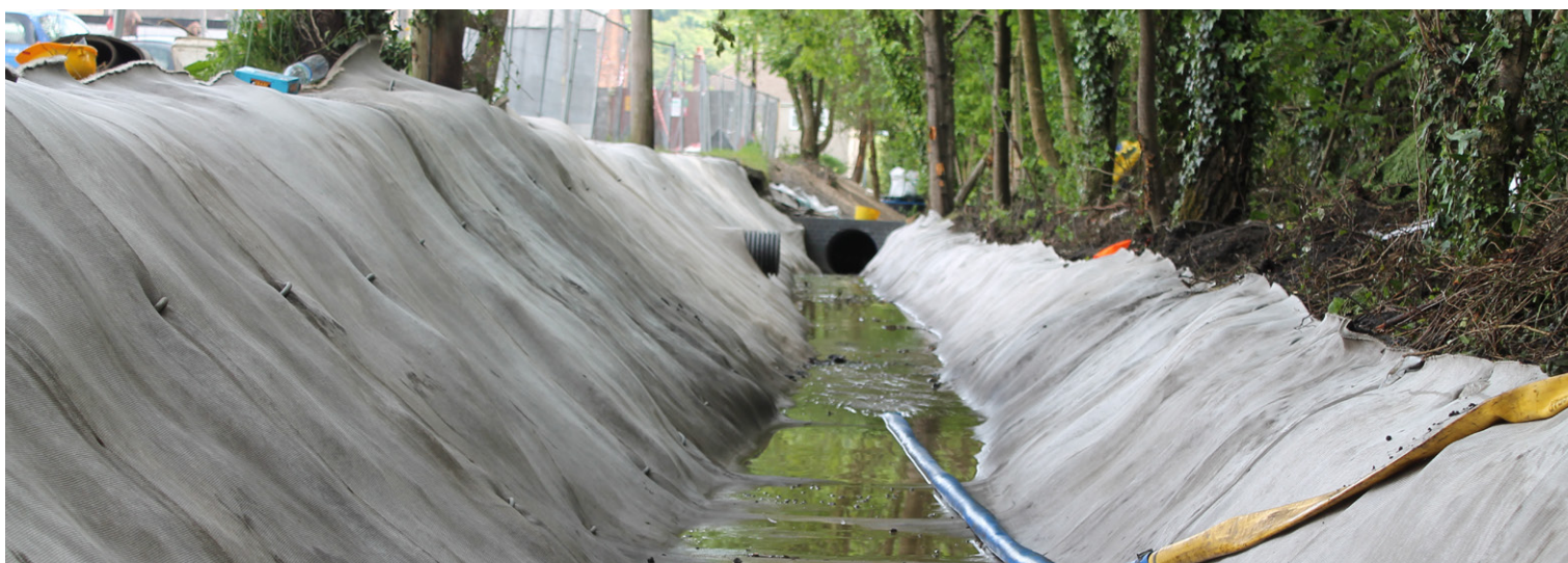
CC was backfilled at the crest of the ditch, providing a neat termination
