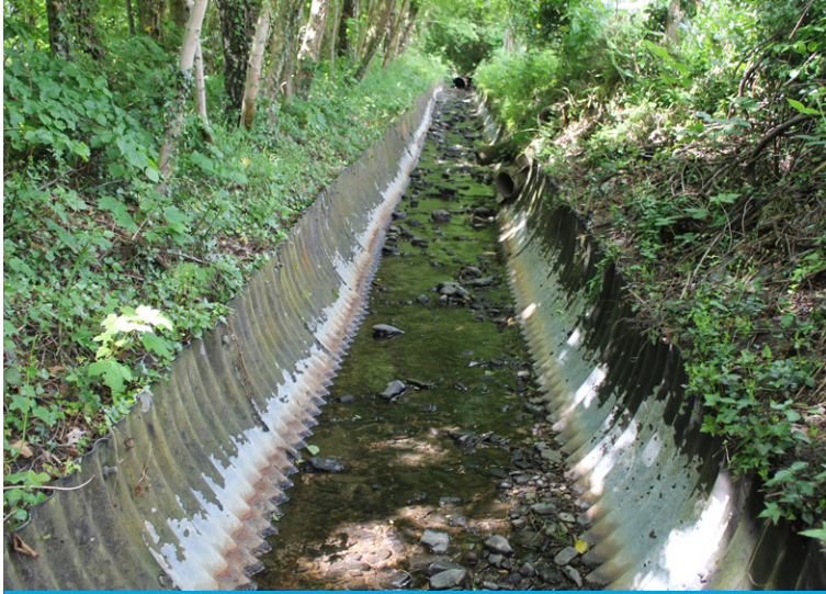
The corroded corrugated steel liner, showing signs of dilapidation
