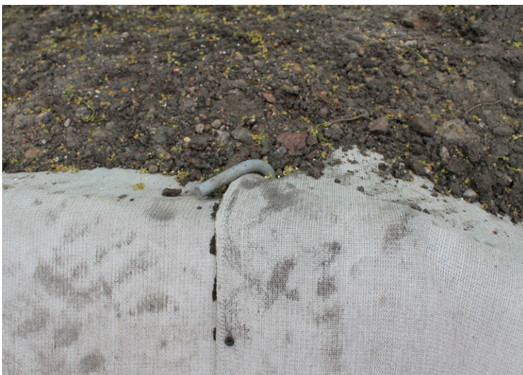
CC was fixed in place using steel ground pegs and backfilling
