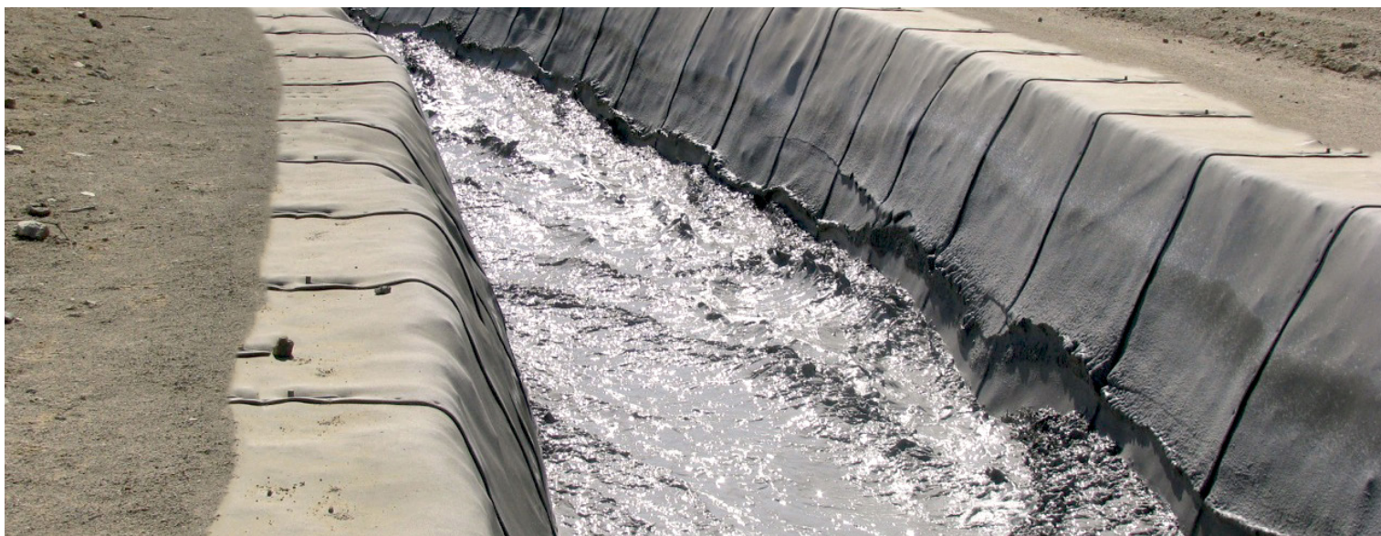
Completed installation showing sedimentation build up along ditch sides
