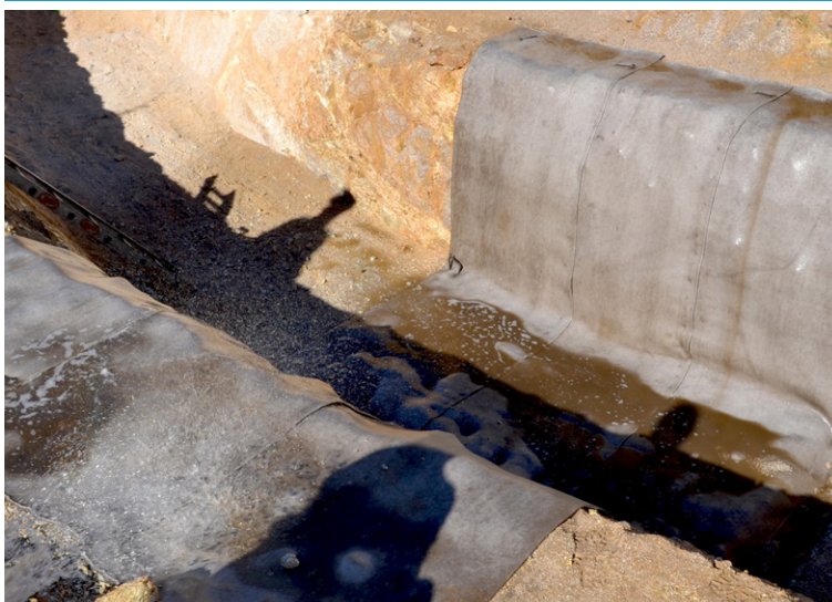
CC hydrated using on-site equipment
