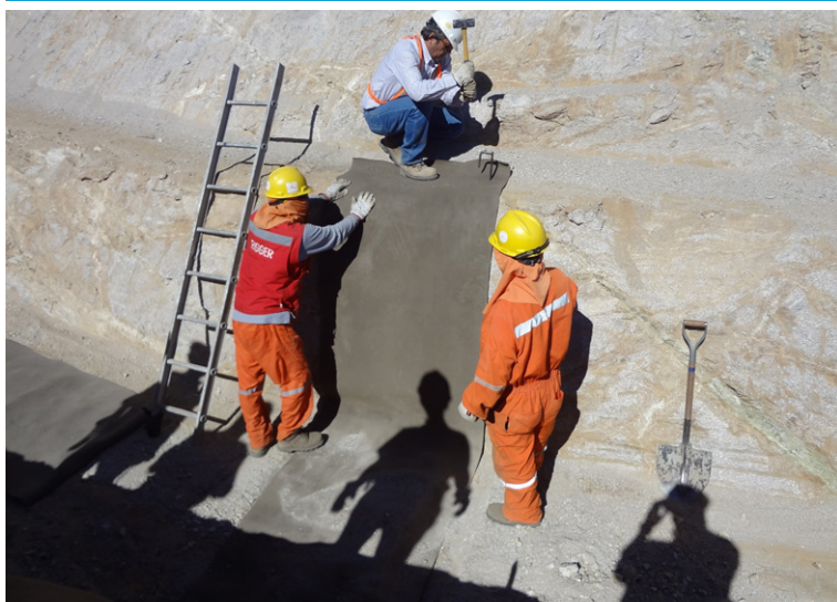
A length of CC being fixed to the crest of the ditch using steel ground pegs
