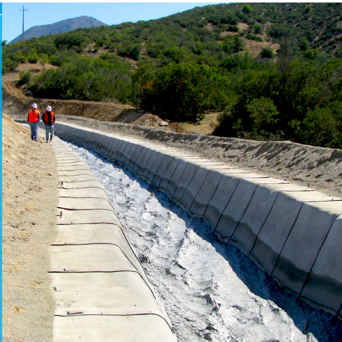
Completed channel lining installation in Chile
