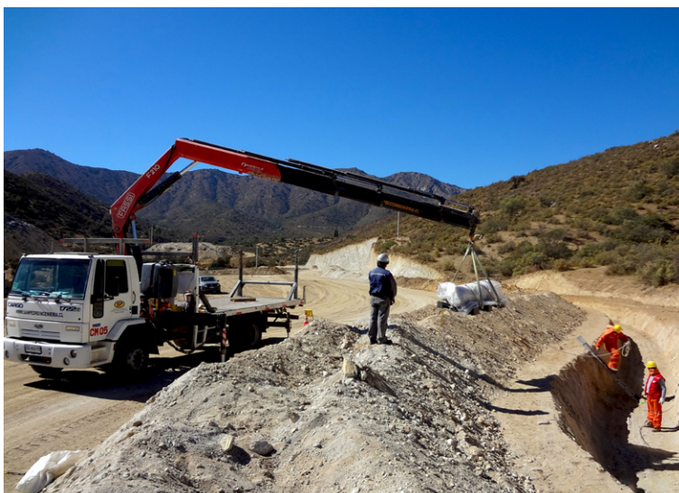
CC8 bulk rolls were cut to length on site, minimising material waste
