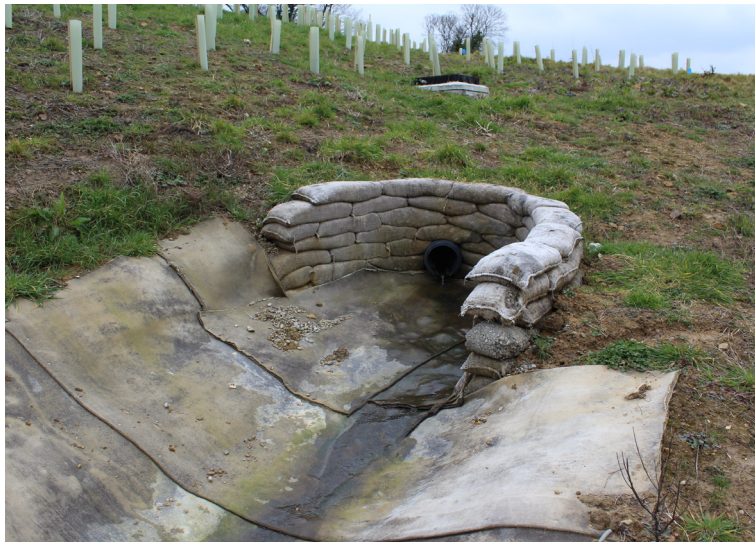
CC termination at concrete sandbag headwall
