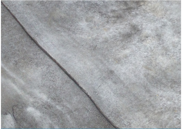
Overlaps were jointed using screws
