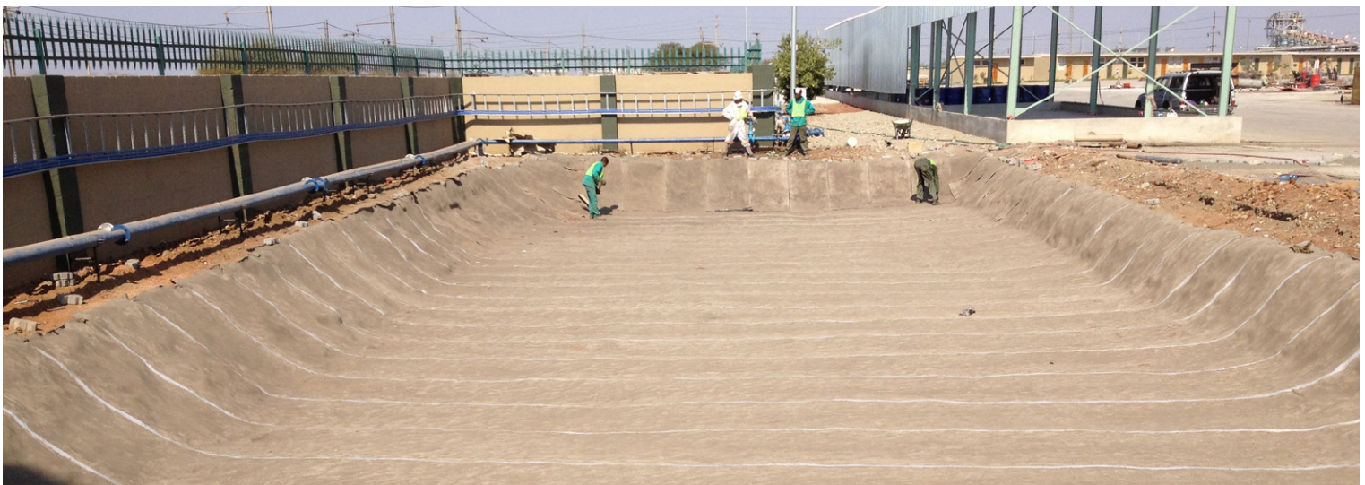
A UV-resistant, waterproof sealant was used to seal the joints on the concrete side
