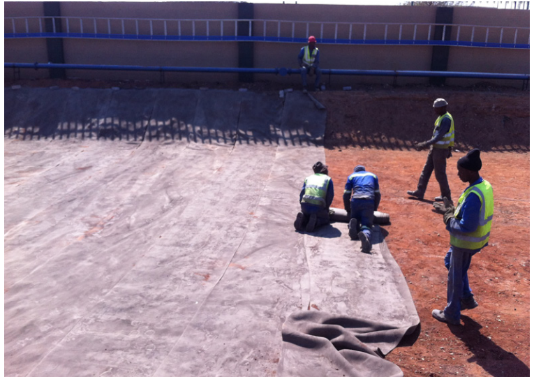
Joints between layers of CC were sealed with a VHB tape underneath
