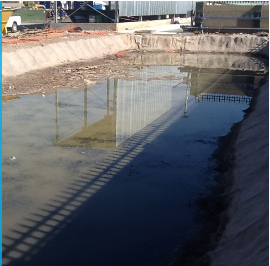
Completed dam lined with CC5™
