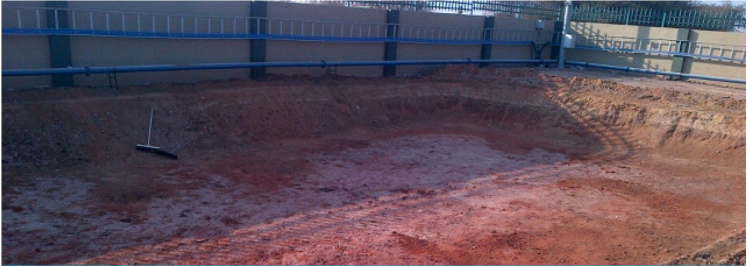
The dam site was excavated and cleared by an on-site team prior to installation of CC
