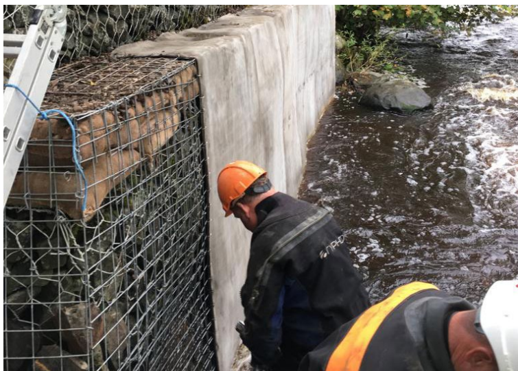
Subsequent layers overlapped by 100mm
