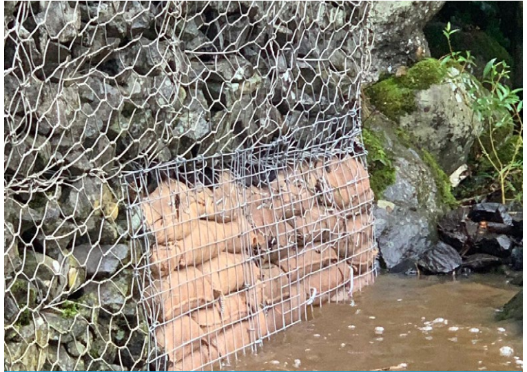
Remediation sections of gabion with sandbags
