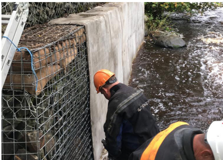
Subsequent layers overlapped by 100mm
