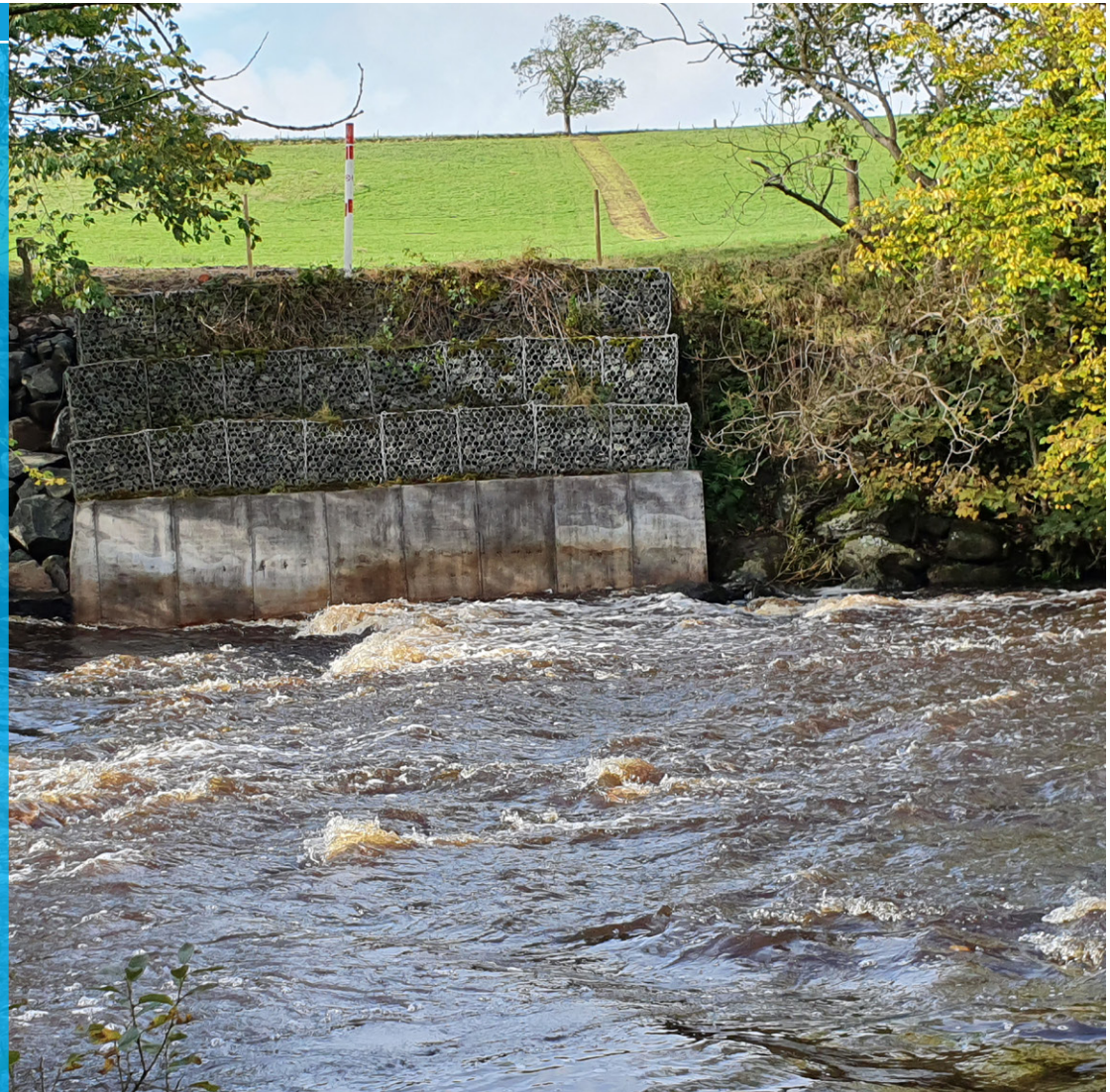
Completed CC installation on the banks of the River Almond, Scotland
