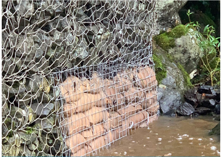
Remediation sections of gabion with sandbags
