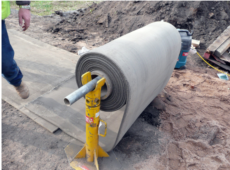
Dispensing 20m pre-cut rolls of CC13 on site before cutting to length
