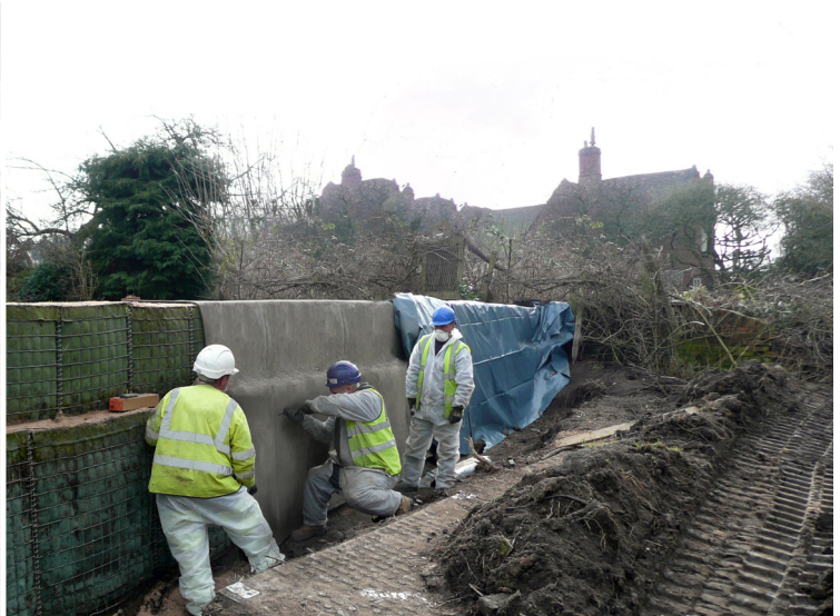
Fixing CC to gabion structures using re-bar staples
