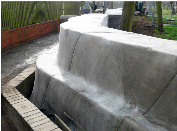
Hydrated CC prior to backfilling toe anchor trench
