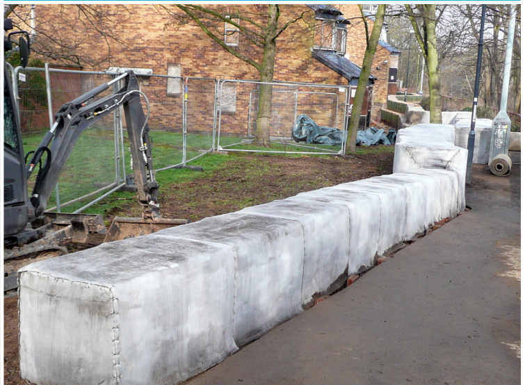
Completed CC lined gabion section
