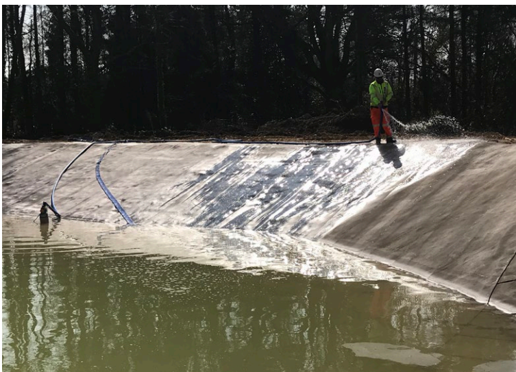
CC8™ Hydrated with a lay flat hose and submersible pump
