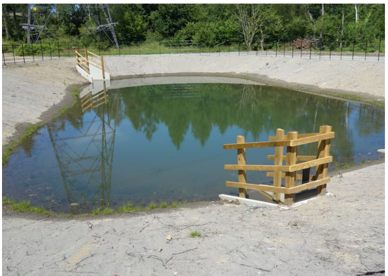
Pond fully lined with CC8™ and clean stone layer
