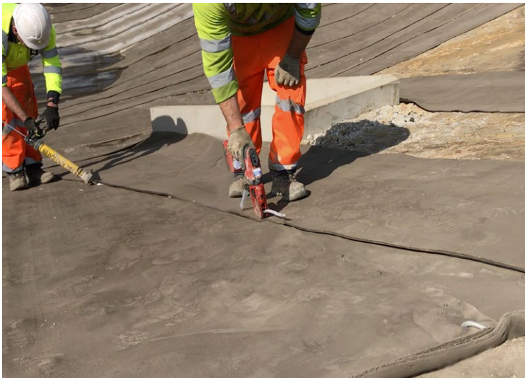
Overlaps secured with adhesive and 30mm screws
