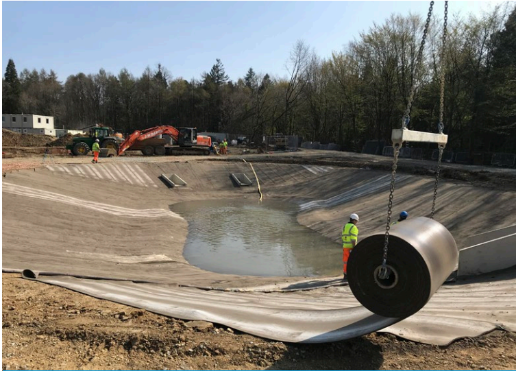
CC8™ lifted and rolled out by spreader beam
