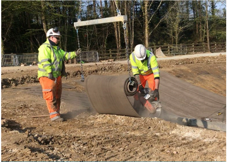
CC8™ cut with disc cutter
