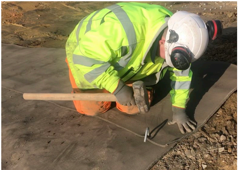
Edges of CC8™ secured with 250mm pegs
