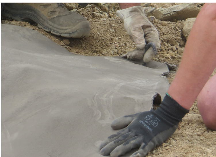
Pegging the CC into the anchor trench
