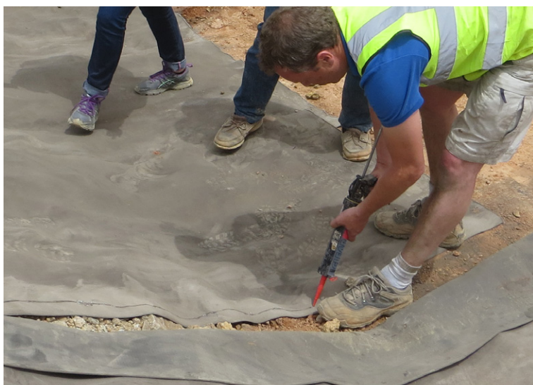
Applying Everbuild Clearfix sealant
