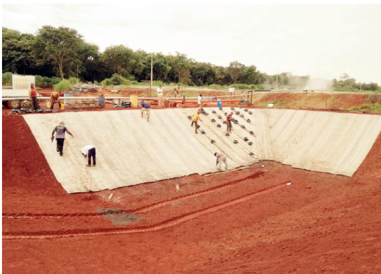
Installation started in middle of long slope, working clockwise
