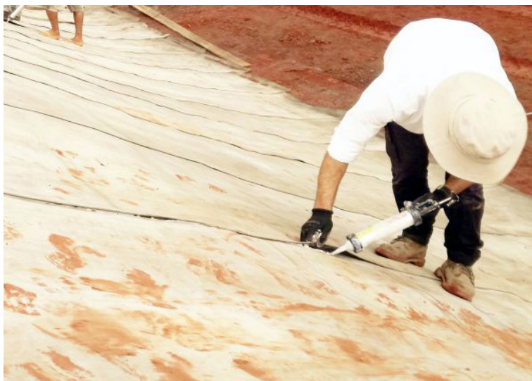
Overlaps were sealed using polyurethane sealant 3M 540
