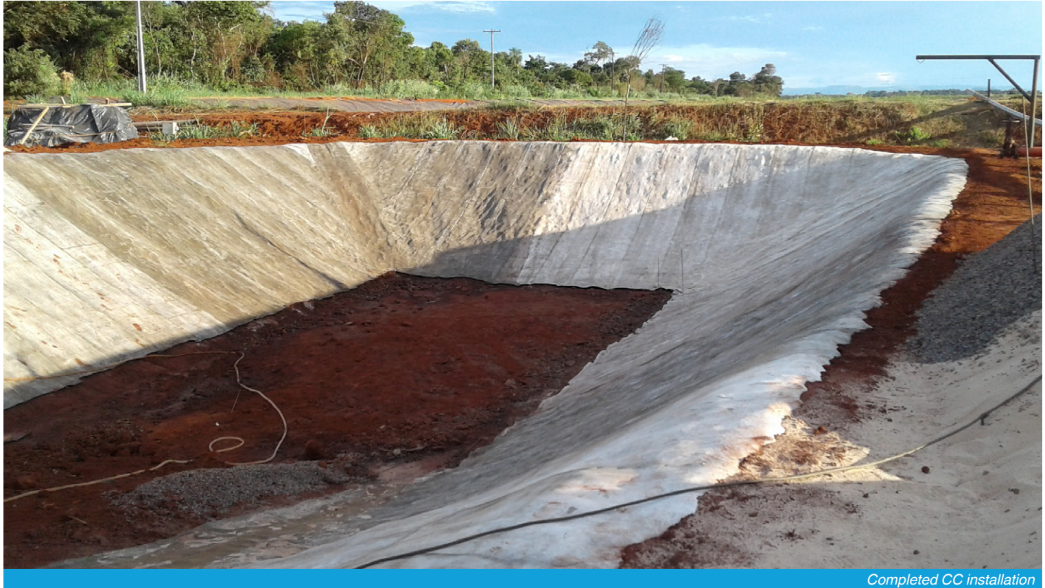
Completed CC installation
