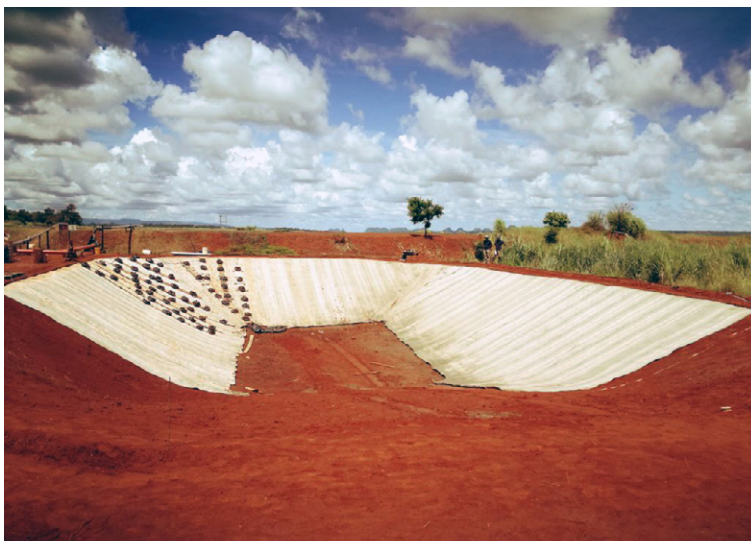
Sandbags were placed along joints while the sealant set
