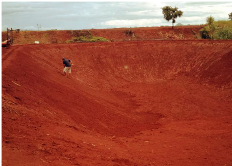
Prior to installation, both lagoons were re-profiled then graded manually
