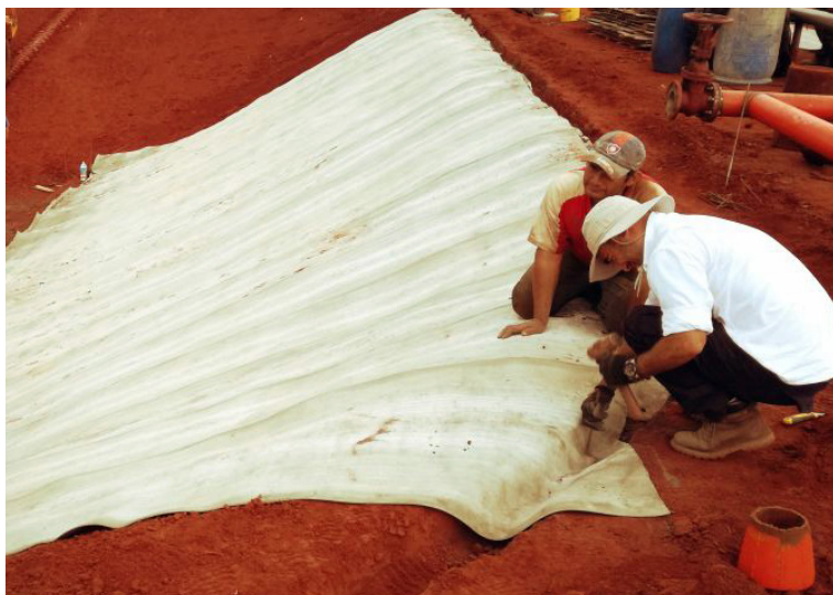
CC was deployed down each slope and pegged in an anchor trench at the crest
