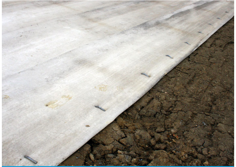
Metal fixings attaching the CC8™ to the clay substrate
