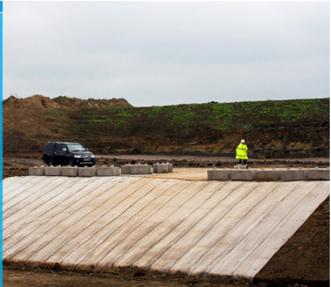
Bank protection installation
