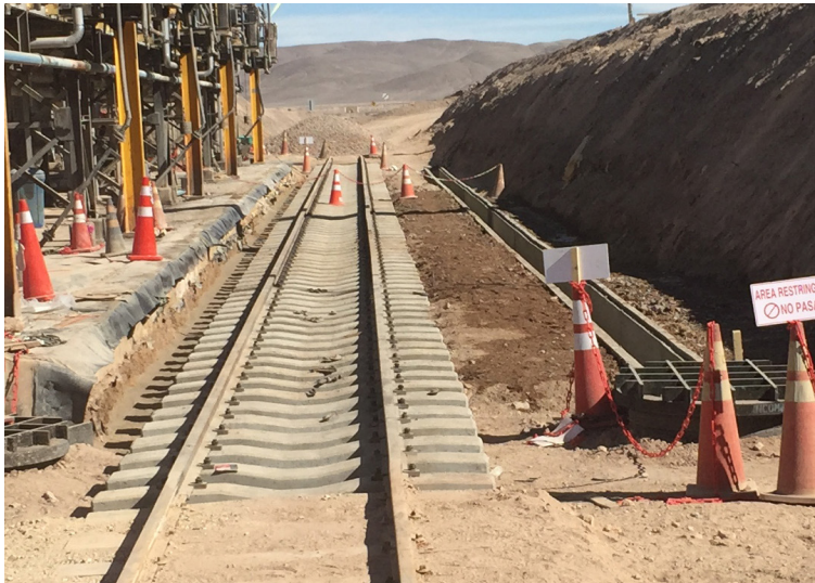
First pre-cast concrete channel installed
