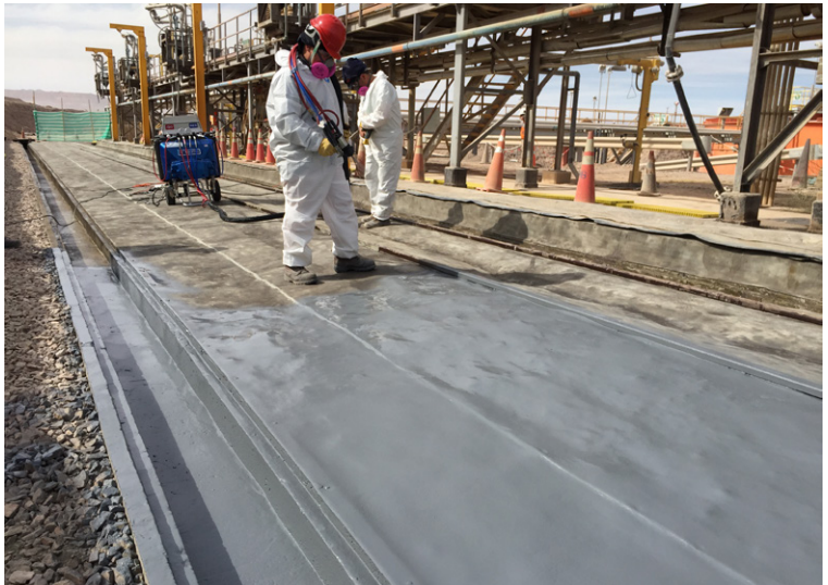
Applying polyuria layer
