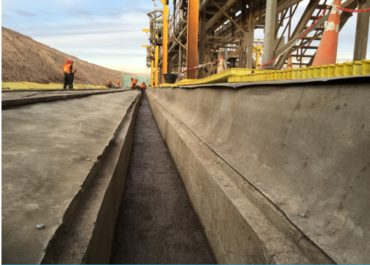
CC screwed to pre-cast concrete channel
