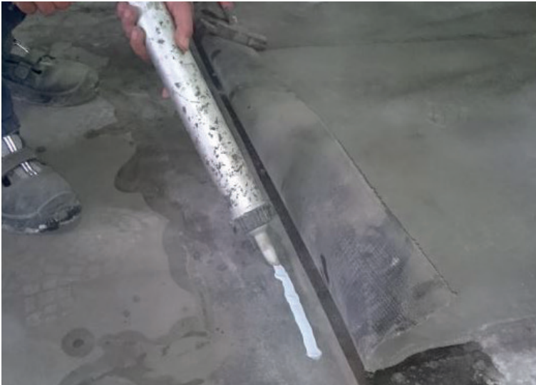
CC joints were sealed using an adhesive sealant
