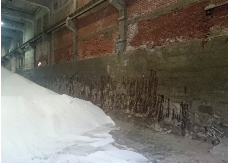
Walls had been corroded by the salt
