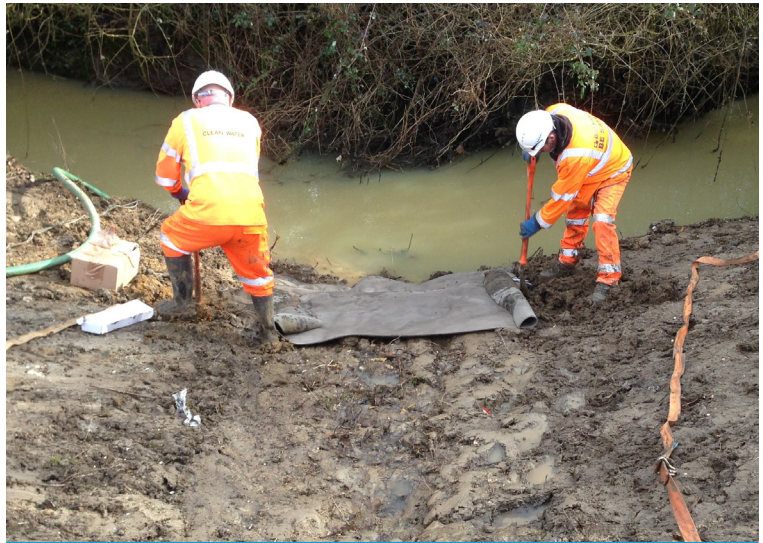
CC was cut to length and installed in a transverse layup working upstream
