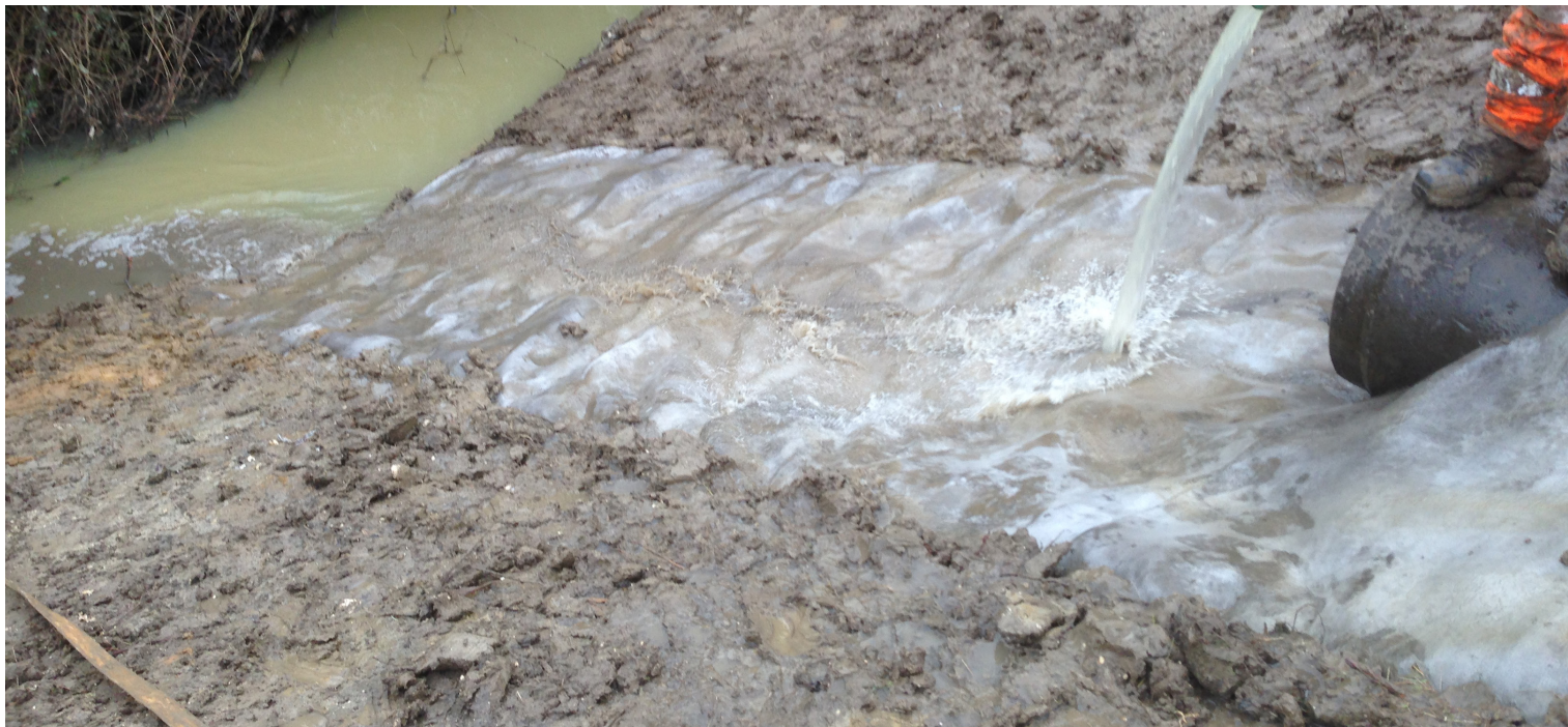
Hydration took place via a pump linked to a nearby stream
