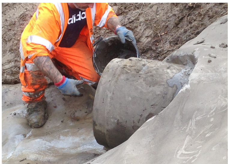
The CC was grouted around the existing pipe
