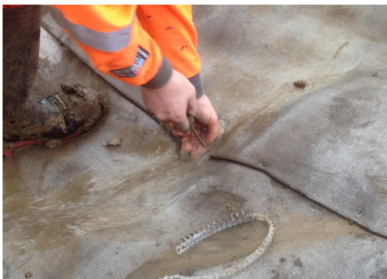
The CC was jointed with stainless screws at 200mm centres
