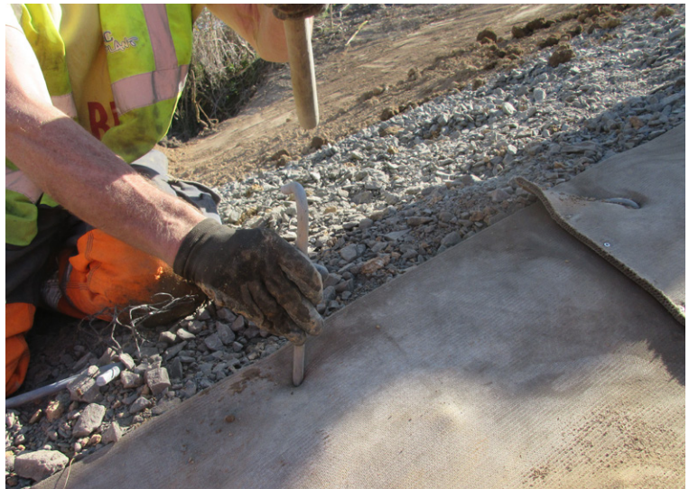
Galvanised steel pegs used to fix the CC8™ to the ground
