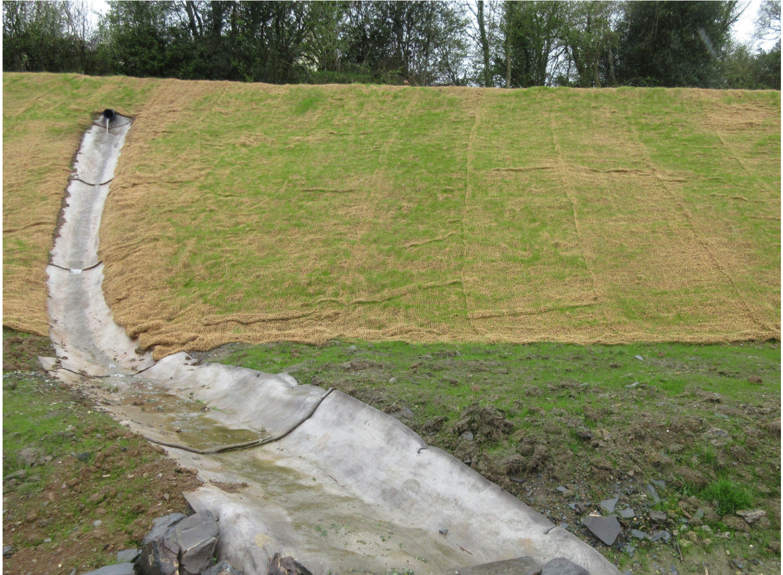
Completed lined channel
