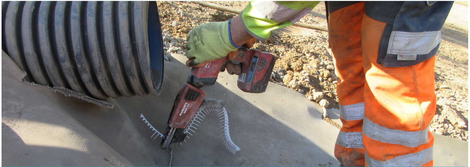
Auto-fed screwdriver being used to joint the CC8™ using 30mm stainless steel screws
