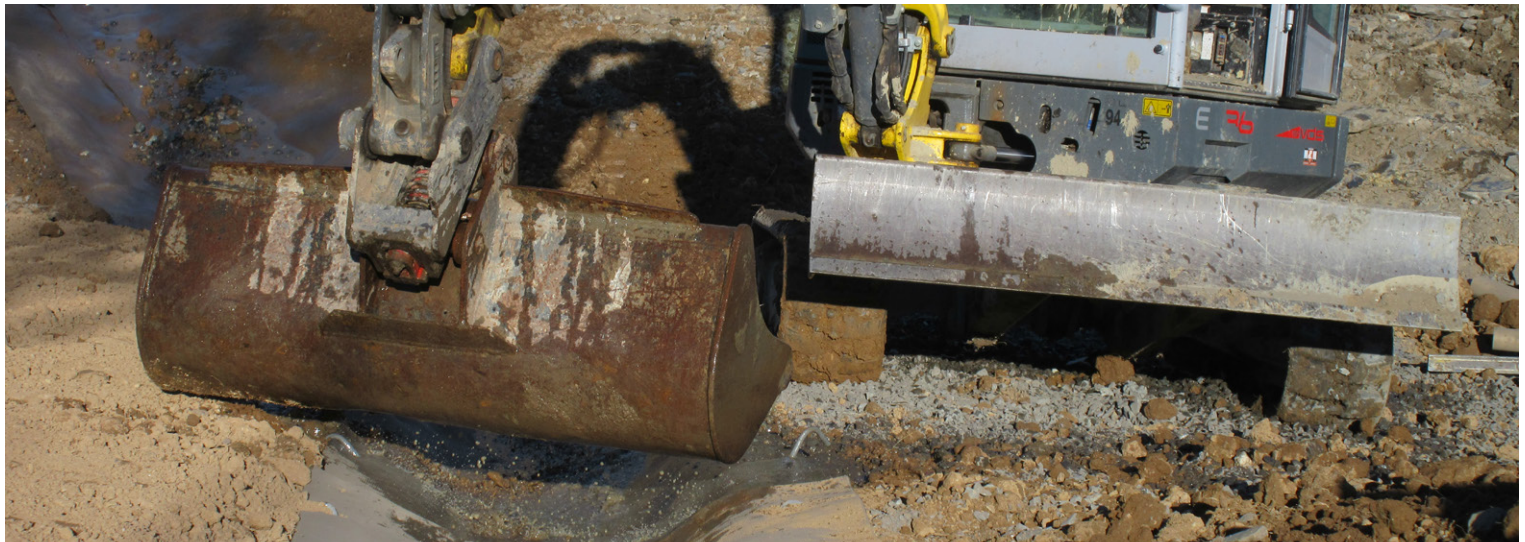
An excavator bucket was used to collect water from a nearby stream to hydrate the CC8™
