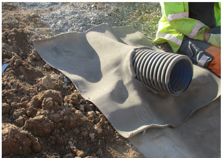
Twin wall carrier pipe installed into outfall channel with a overhang detail
