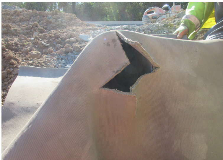
Opening cut into CC8™ material for 250mm dia twin wall carrier pipe
