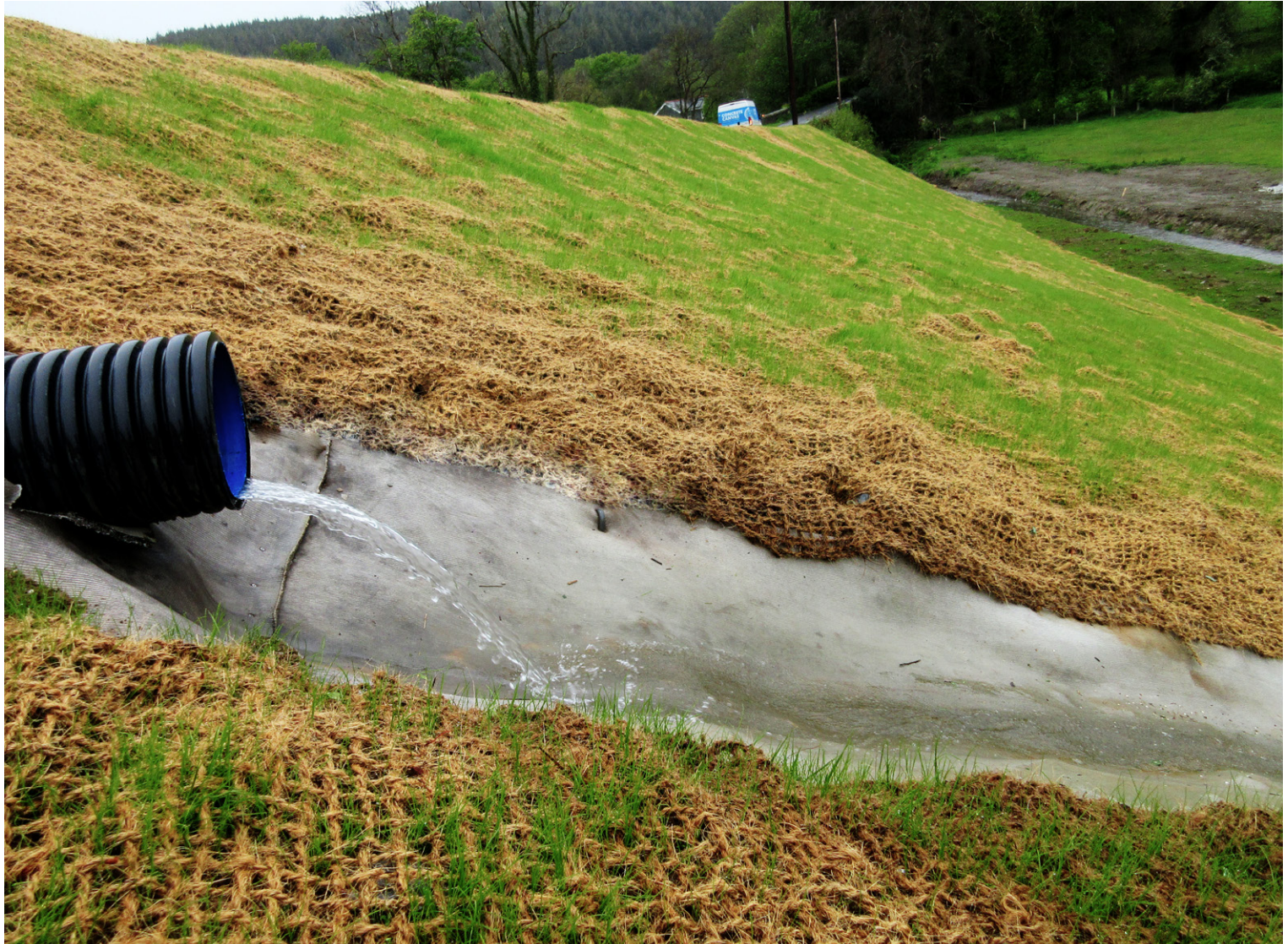
Completed and lined channel with water flowing from the outfall
