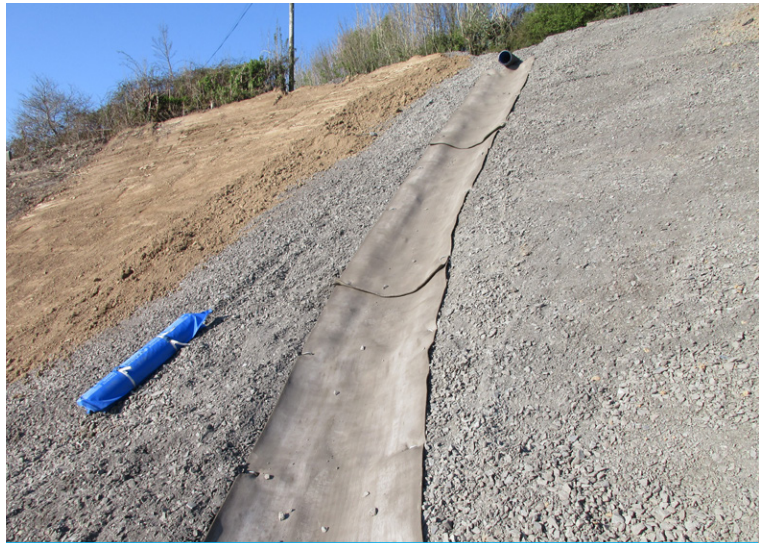
Batched Rolls installed longitudinally down the outfall
