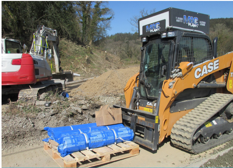
CC8™ Batched Rolls being transported to the top of the outfall
