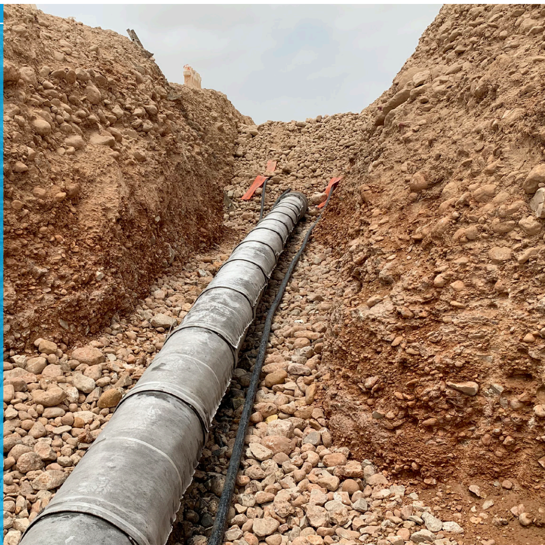
Completed CC pipe protection installation in Salalah, Oman
