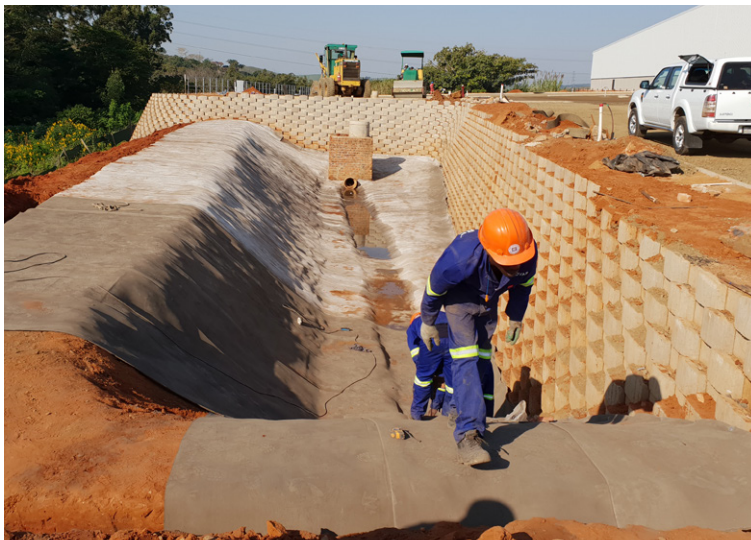
Deployment of CC on second day of installation
