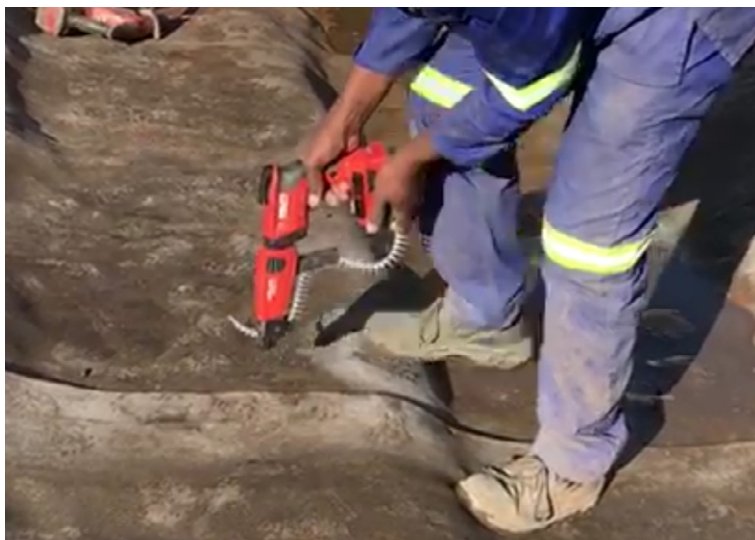
Joining CC overlaps using screws
