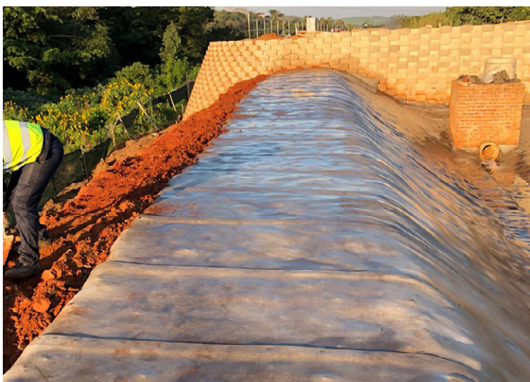
CC termination within anchor trench
