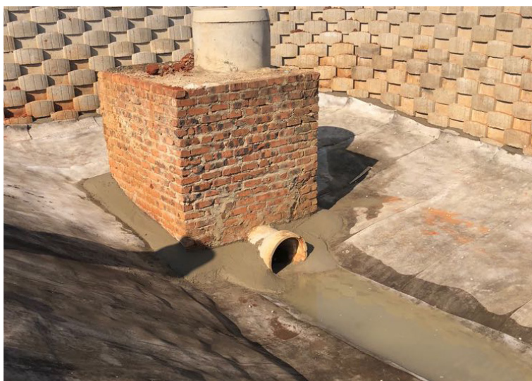
Termination of CC at outlet headwall
