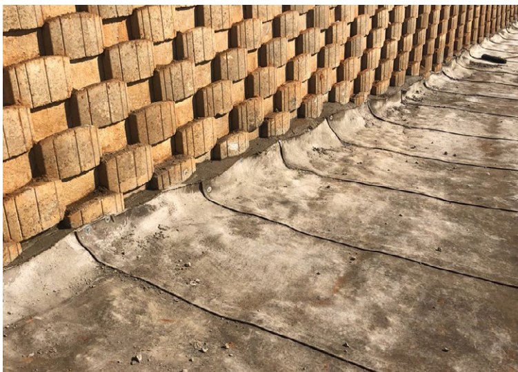
Termination of CC against dry-stack wall
