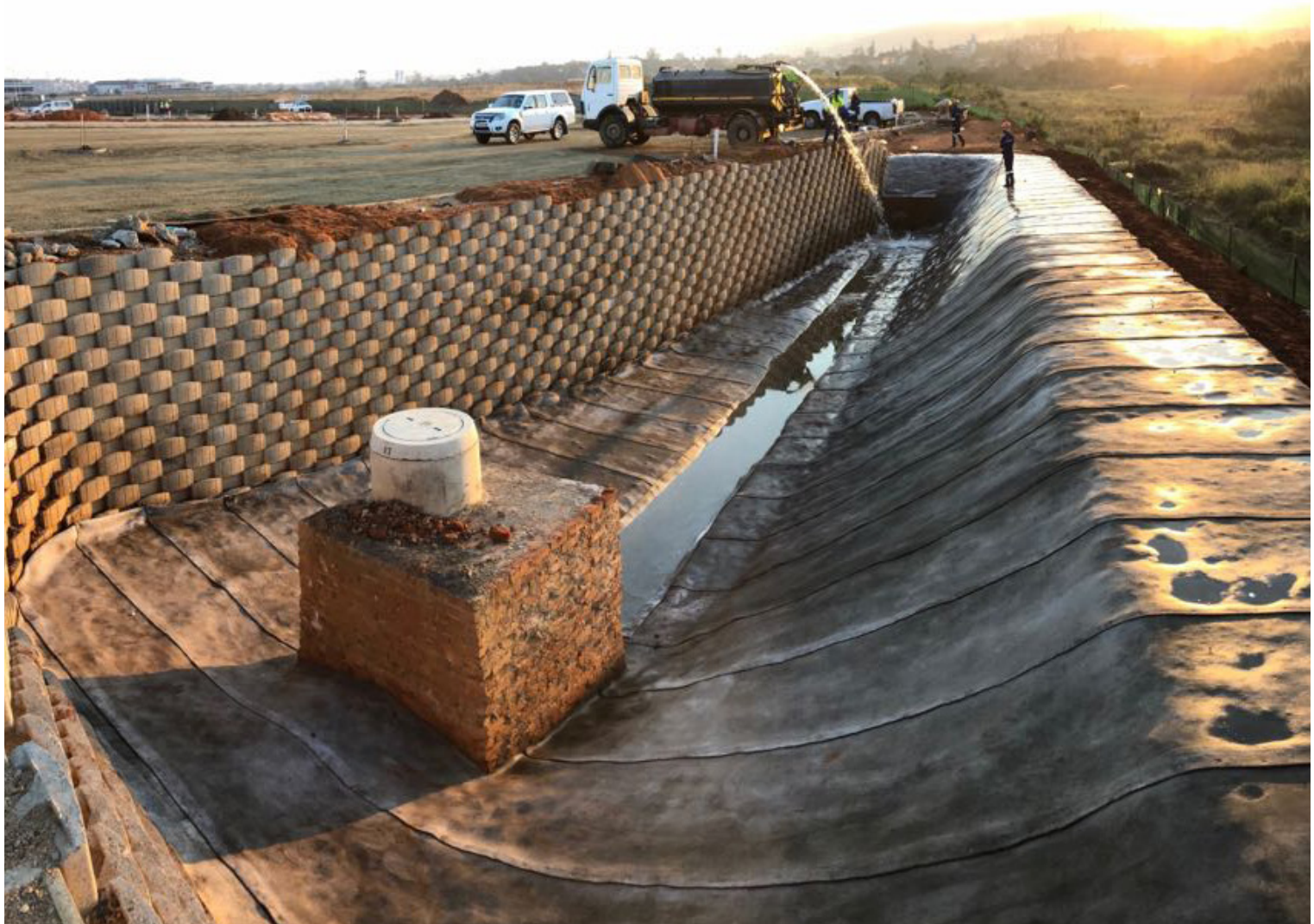
Hydration of completed installation
