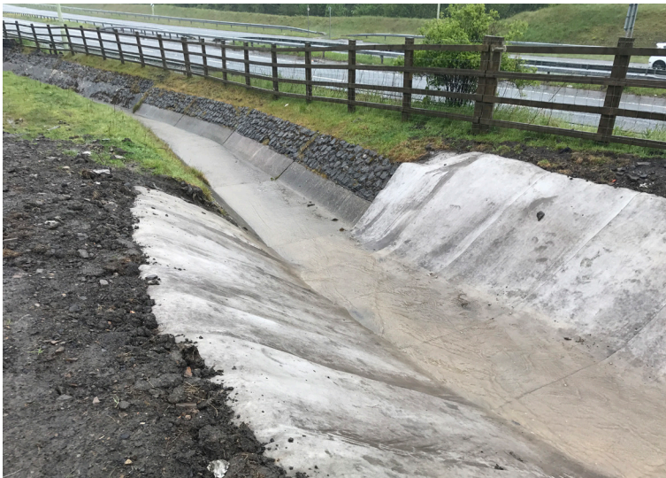
Termination of the CC to the existing concrete channel
