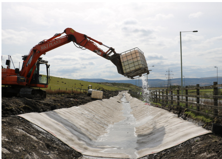
Each section was hydrated when completed
