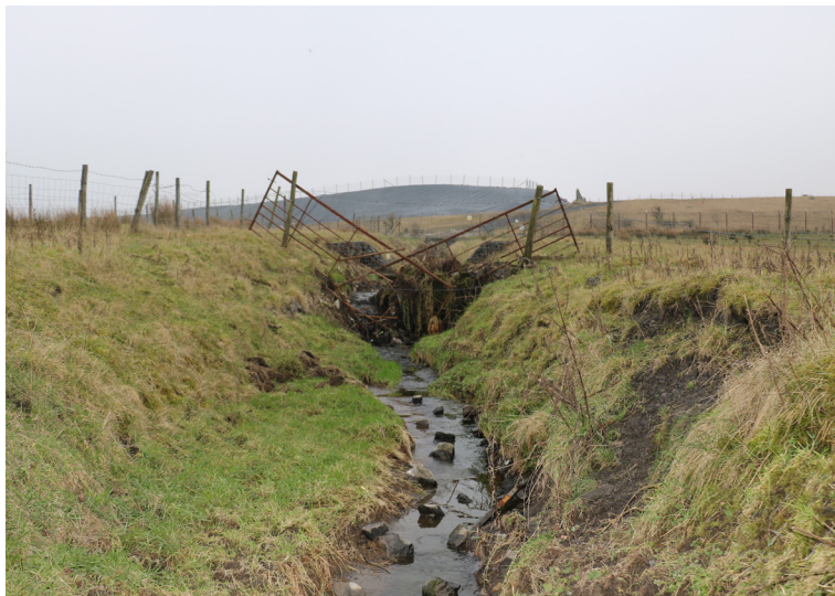
Unlined sections of the channel were overgrown and at risk of blockage
