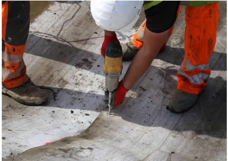
On concrete infrastructure, overlaps were fixed using Hitli concrete fixings
