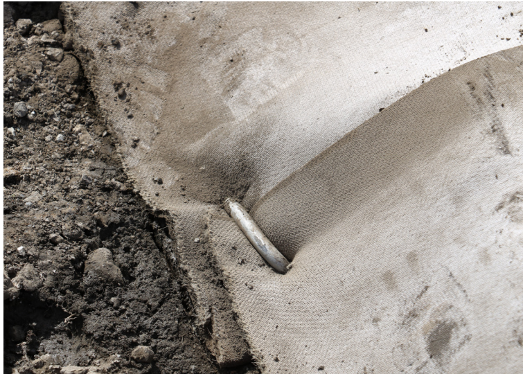
CC was fixed in anchor trenches with ground pegs
