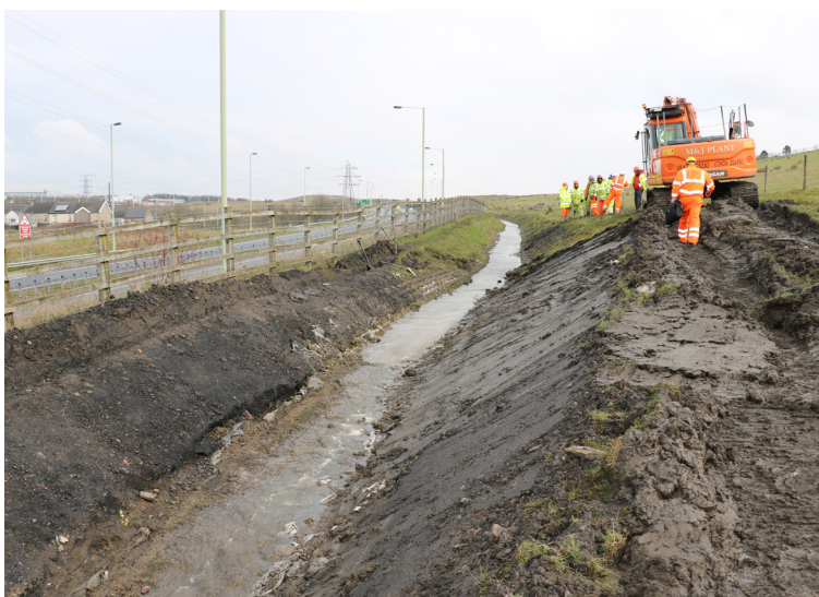
The channel was re-graded prior to works to ensure a successful installation
