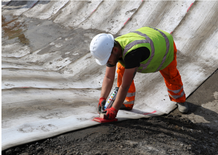
Each additional layer of CC laid was overlapped by 100mm
