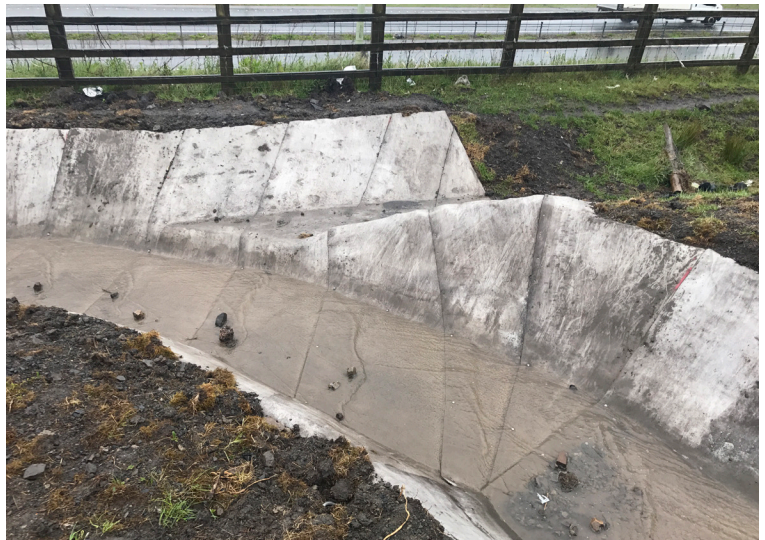
The CC's flexibility was able to accommodate complex sections of the channel
