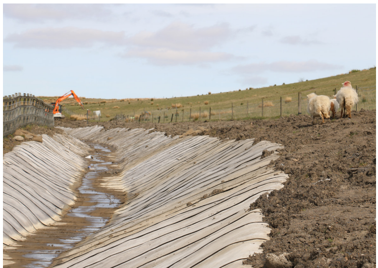
A transverse layup was used to allow for the varying profile width
