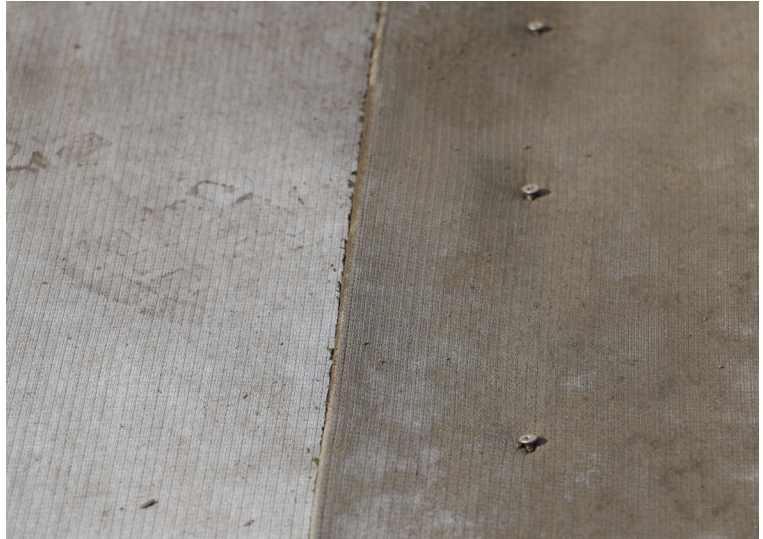
Overlaps were jointed using stainless steel screws on soil substrate
