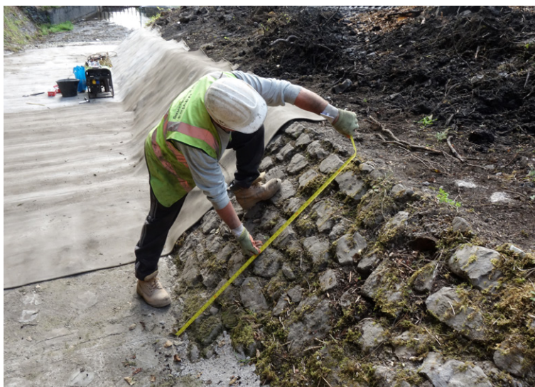
CC was cut to required lengths for each channel section
