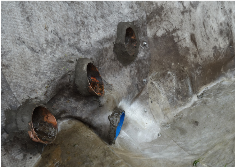
CC cut to accomodate pipe protrusions and edges sealed with grout
