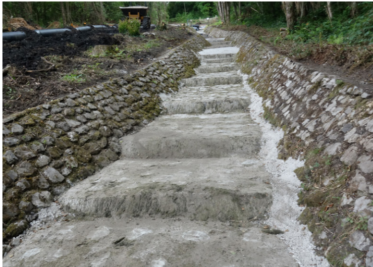
Rocks removed from channel invert and voids filled with fast setting concrete
