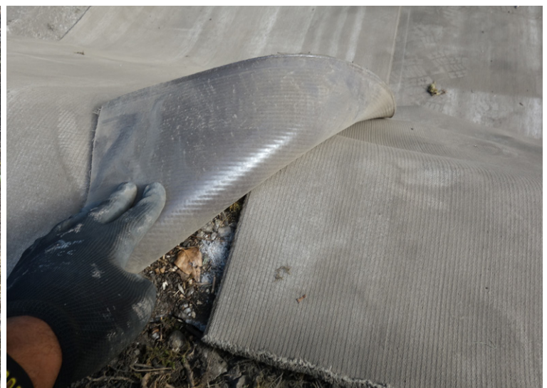
Subsequent layers of CC overlapped by 100mm
