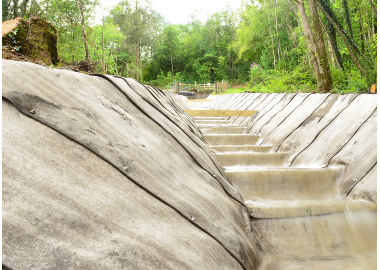
CC was able to accomodate steps created as baffling solution
