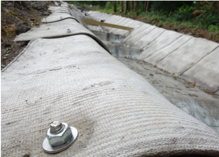
CC edges secured to concrete channel and later backfilled
