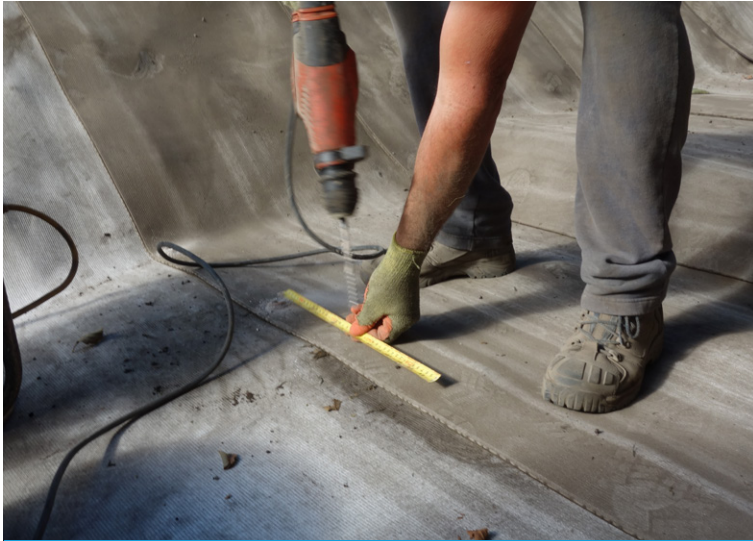
Holes drilled through CC into concrete below for installation of throughbolts
