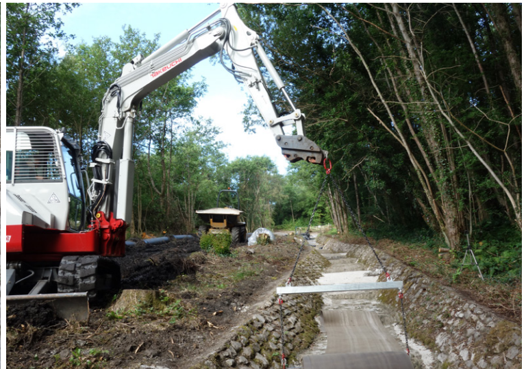
CC deployed from excavator and spreader beam
