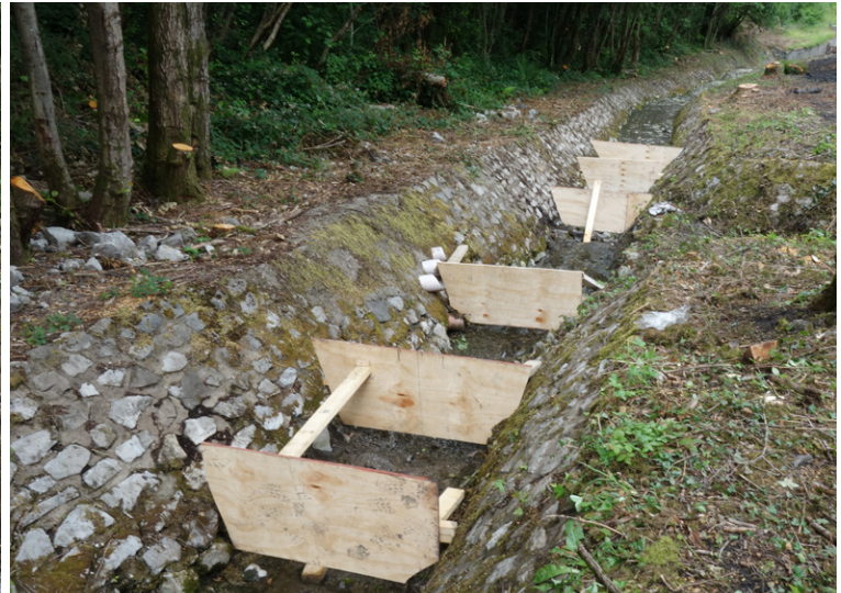
Shuttering was installed for installation of concrete base
