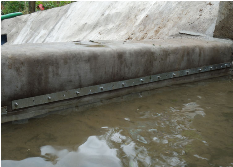
CC termination detail using steel clamping bar
