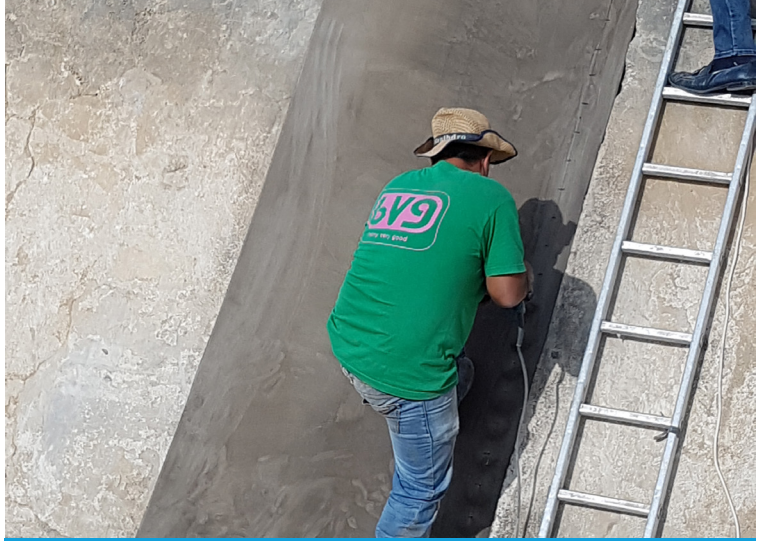
Fixing CC into construction joints
