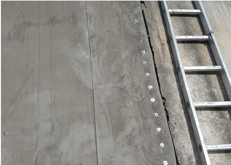
Close up of thru bolts at construction joints
