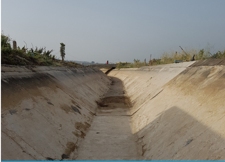
Graded canal section following removal of vegetation
