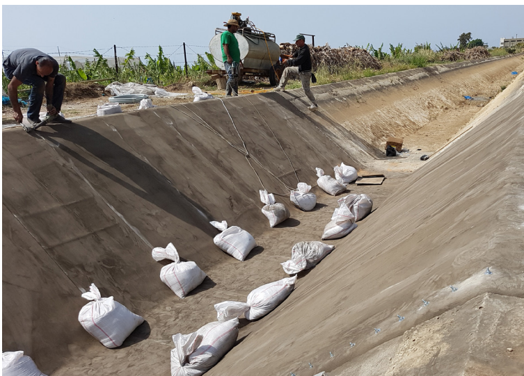
Compressing using sandbags
