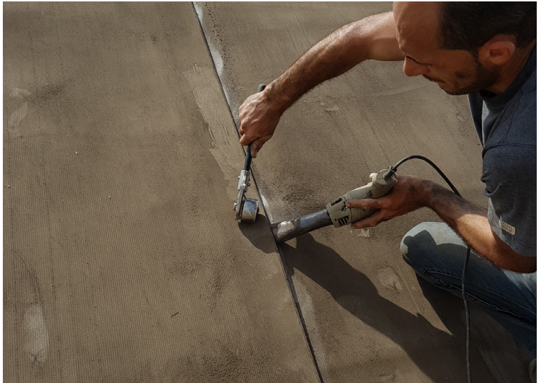
Adjacent lengths of CC overlapped by 100mm by sealing and thermal bonding
