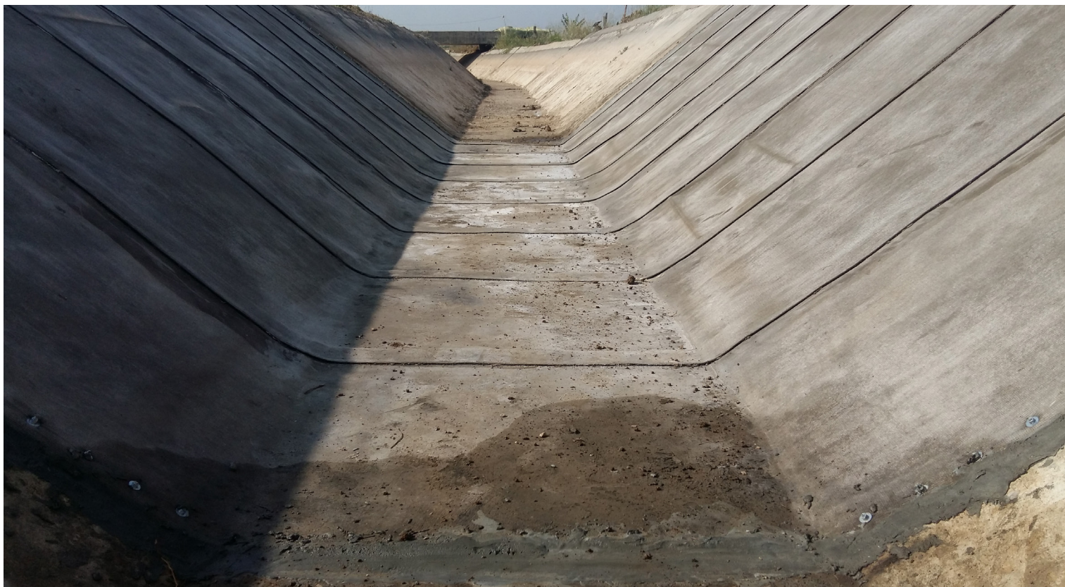
Completed section of channel post installation and close up of grout mortar termination
