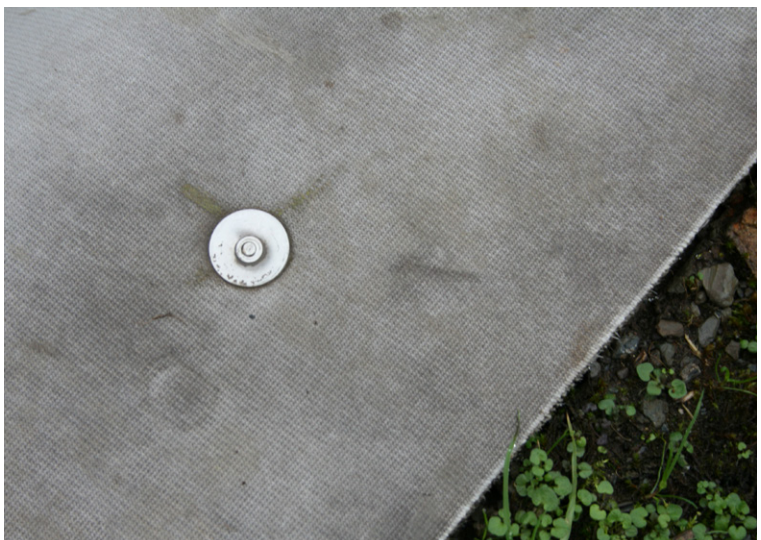
CC5 fixed using 34mm Hilti nails with 25mm diameter
