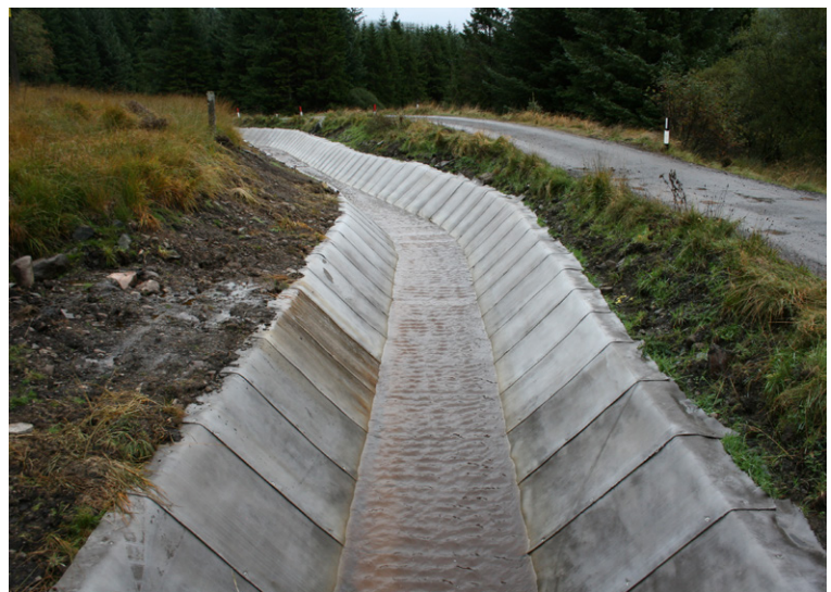
CC layers overlapped in direction of water flow providing natural weep paths
