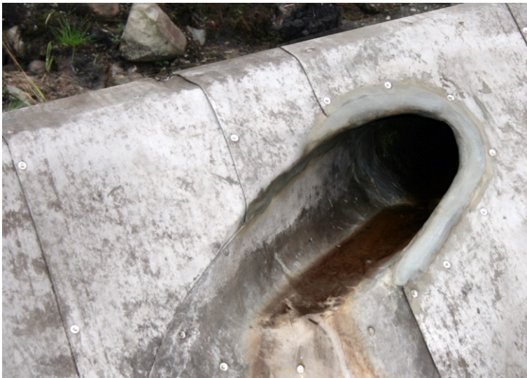
Intermediate intake pipe lined with CC and finished flush with grout
