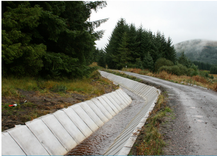
Remediated flume lined with CC5 transverse layers
