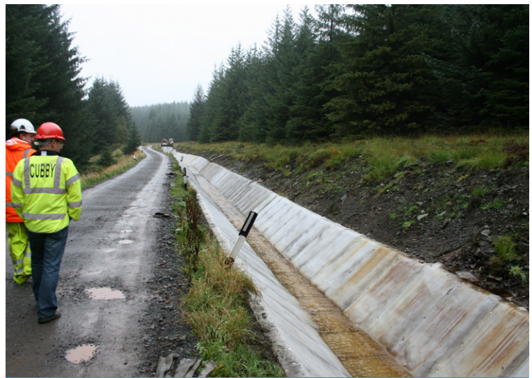
CC installed at rates of up to 600m 2 per day
