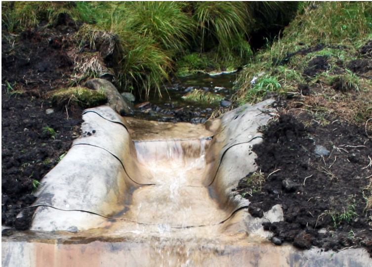
Inlet channels lined with CC to direct bank runoff into flume
