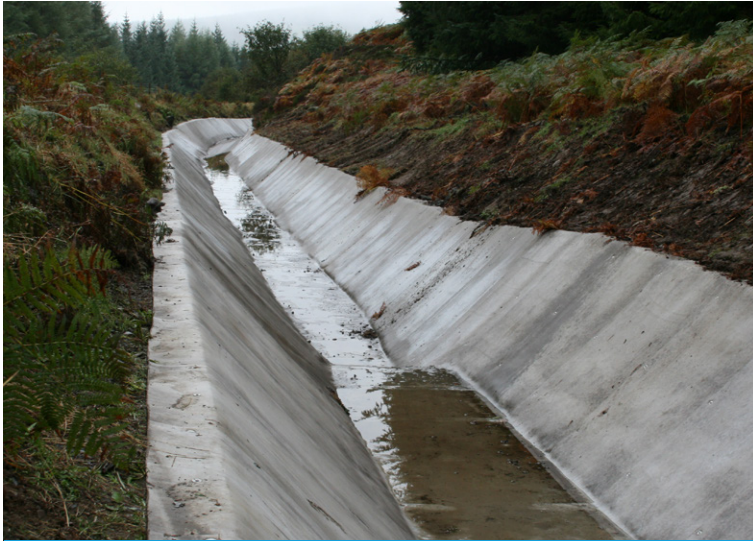
Remediated flume lined with transverse layers of CC5
