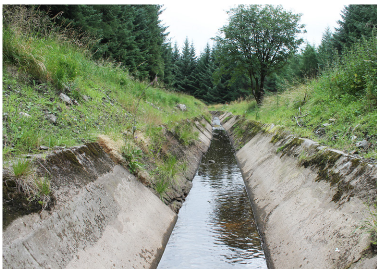
1.5km dilapidated concrete slabbed flume prior to installation
