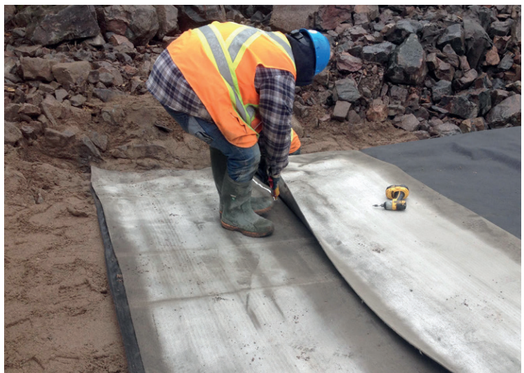
Sealing joints
