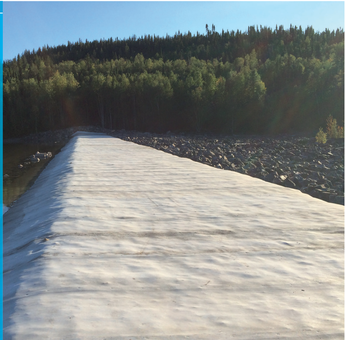
Completed CC weir dam
