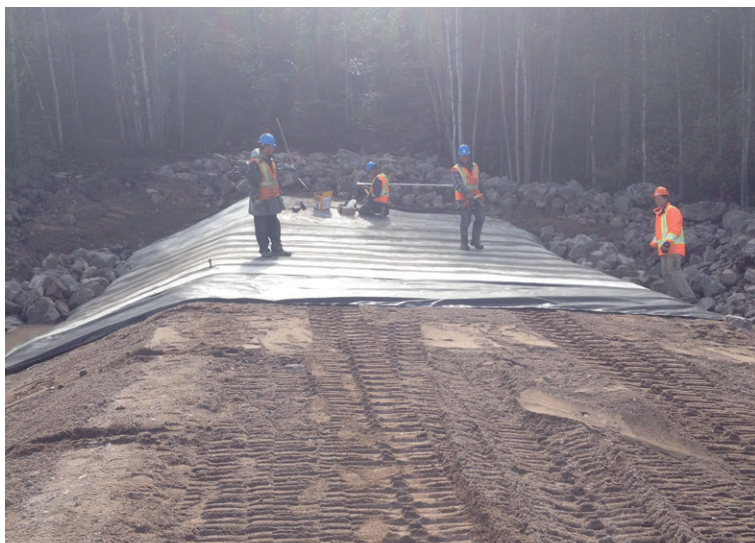
Bulk rolls were deployed transversely across weir dam
