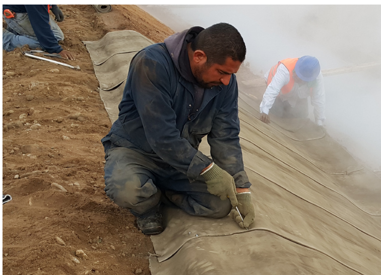
The CC was fixed to the substrate using ground pegs
