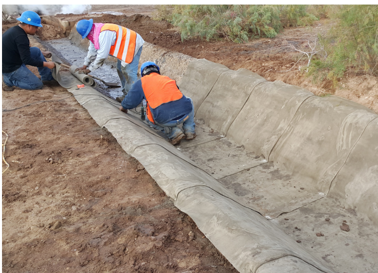
Layers were overlapped by 100mm
