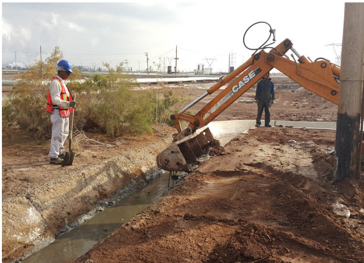
The channel was cleared of debris and water prior to installation
