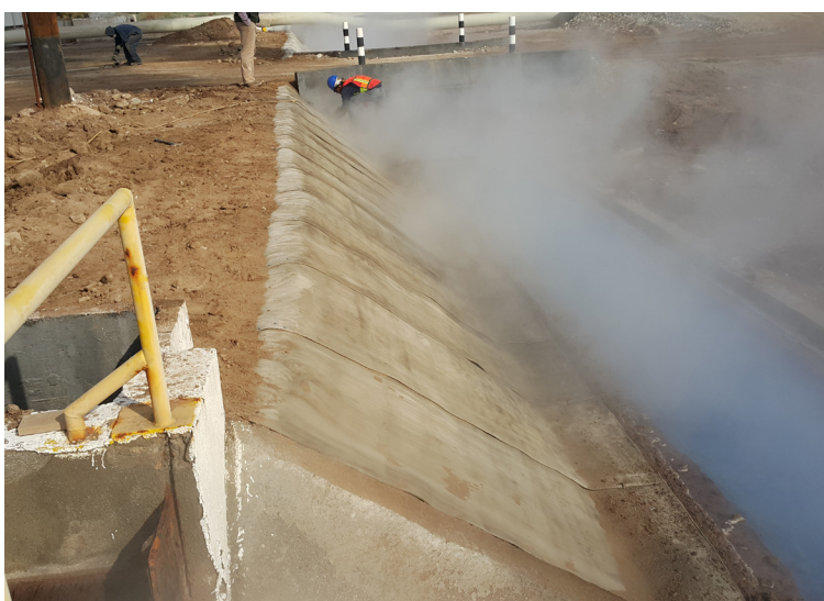
The edges of the CC were captured in anchor trenches
