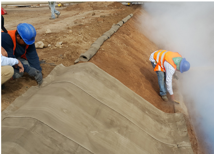
The CC was cut to required length and laid across the crest of the slope
