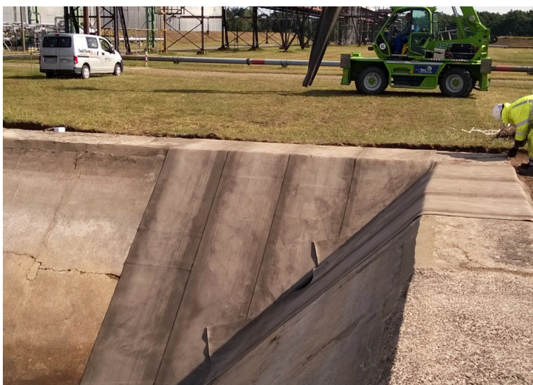
Installation of CC around corner
