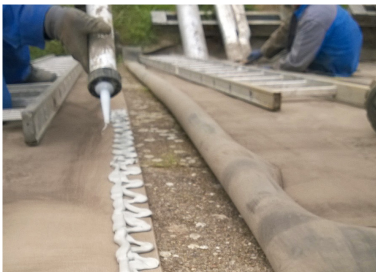
Overlaps sealed using approved adhesive sealant
