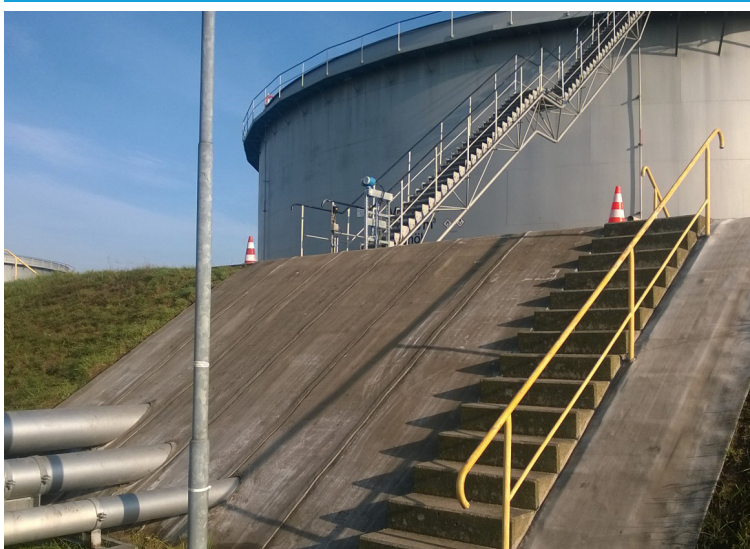
CC installed around pipework and steps
