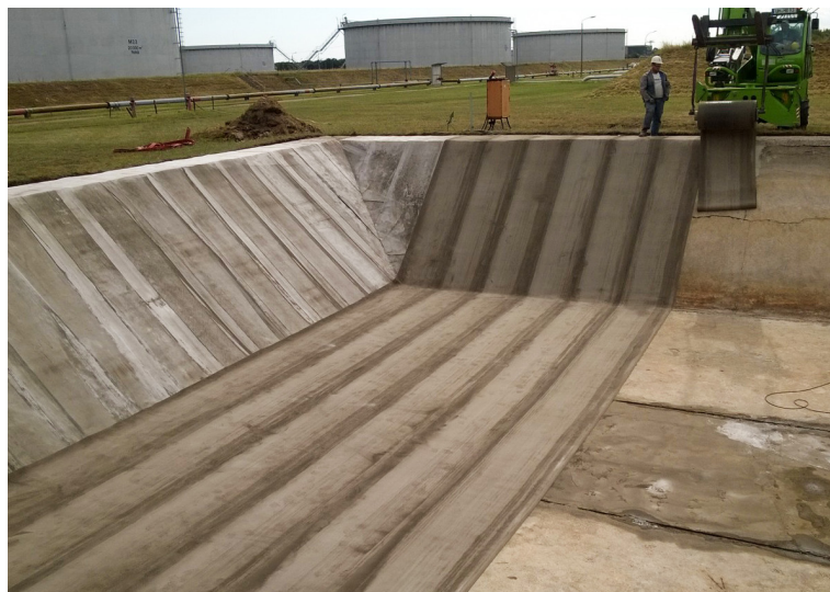
Installation of CC across width of extinguishing lake
