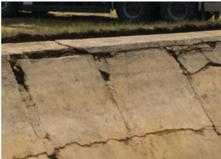
Severe cracking around existing concrete lake
